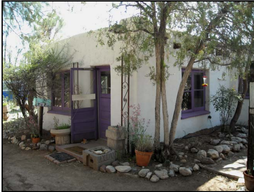
Figure 6. Adobe house at Owen Homesite, view facing southwest (2010).
