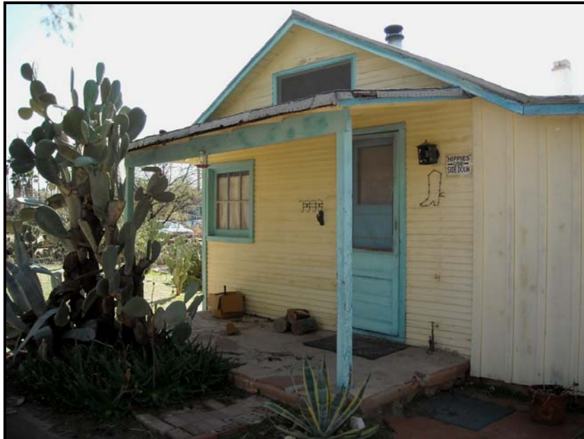
Figure 7. Wood-frame house salvaged from former Tucson Airport, view facing southwest (2010).
