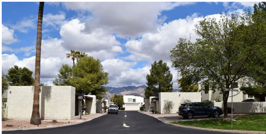
Photograph 4. Overview looking down E. Chorro Circle and Camino del Rio showing Floor Plans A, C, and D (Plan D is to right of frame). View facing north (WestLand Resources 2025 [AZ_PimaCounty_VilladelRio_004])
