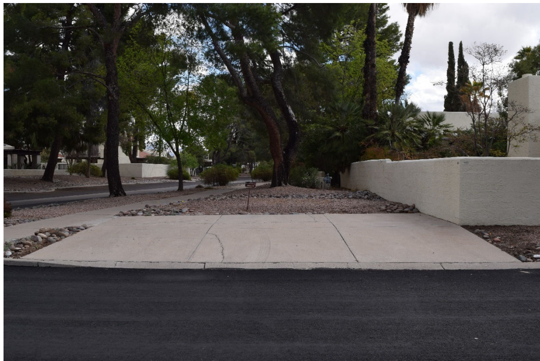
Photograph 20. Example of guest parking at Villa del Rio. View facing east (WestLand Resources 2025 [AZ_PimaCounty_VilladelRio_020])
