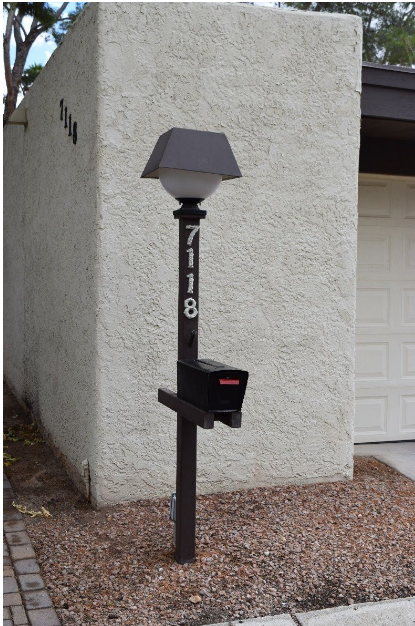
Photograph 19. Typical mailbox and lamp per each residence. View facing east (WestLand Resources 2025 [AZ_PimaCounty_VilladelRio_019])
