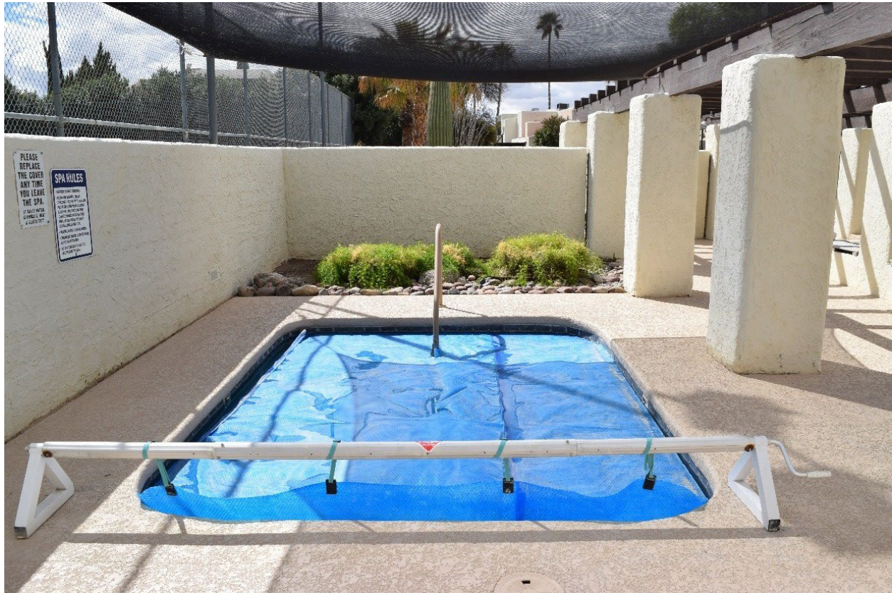
Photograph 9. Overview of the jacuzzi within the pool complex. View facing south (WestLand Resources 2025 [AZ_PimaCounty_VilladelRio_009])
