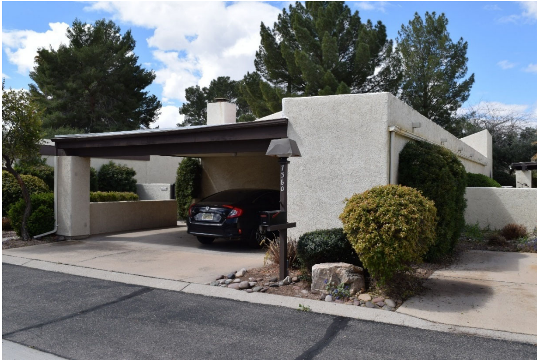
Photograph 1. Typical one-story unit representative of Floor Plan A at 7360 E. Cascada Circle built in 1978. View facing southwest (WestLand Resources 2025 (AZ_PimaCounty_VilladelRio_001))
