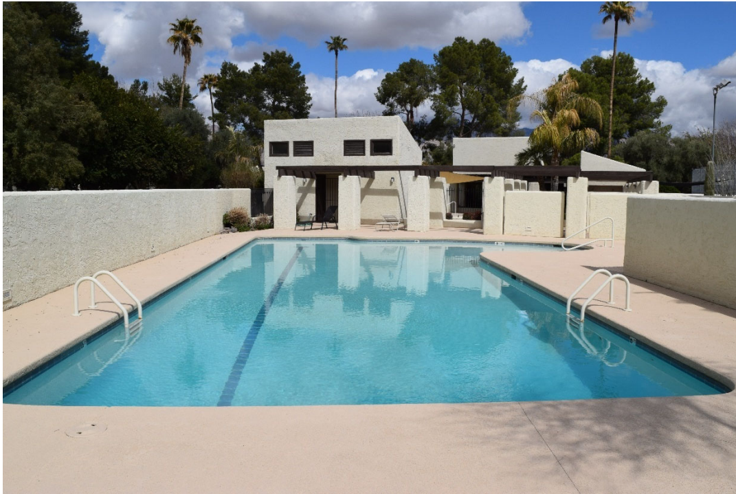
Photograph 10. Overview of the south pool within the pool complex. View facing south (WestLand Resources 2025 [AZ_PimaCounty_VilladelRio_010])
