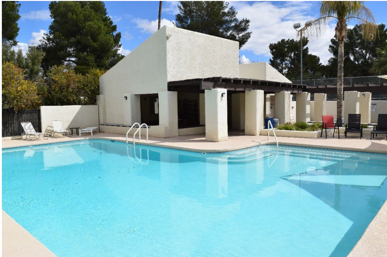
Photograph 8. Overview of the north pool and changing room within the pool complex. View facing northeast (WestLand Resources 2025 [AZ_PimaCounty_VilladelRio_008])
