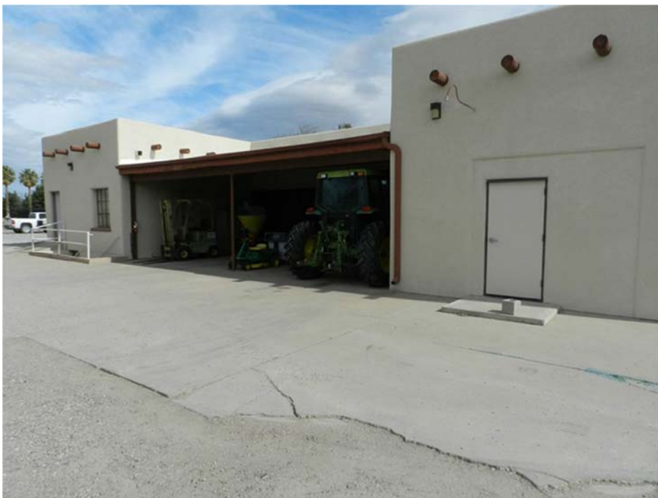
Figure 10: The headquarters with the Administrative Building looking northeast. Photo by: Caitlin Brown (2014).
