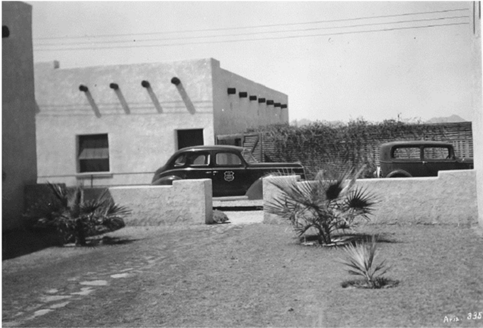
Figure 11: The headquarters with the Administrative Building looking west (ca. late 1930s). Photo Courtesy: Heather Dial (TPMC).
