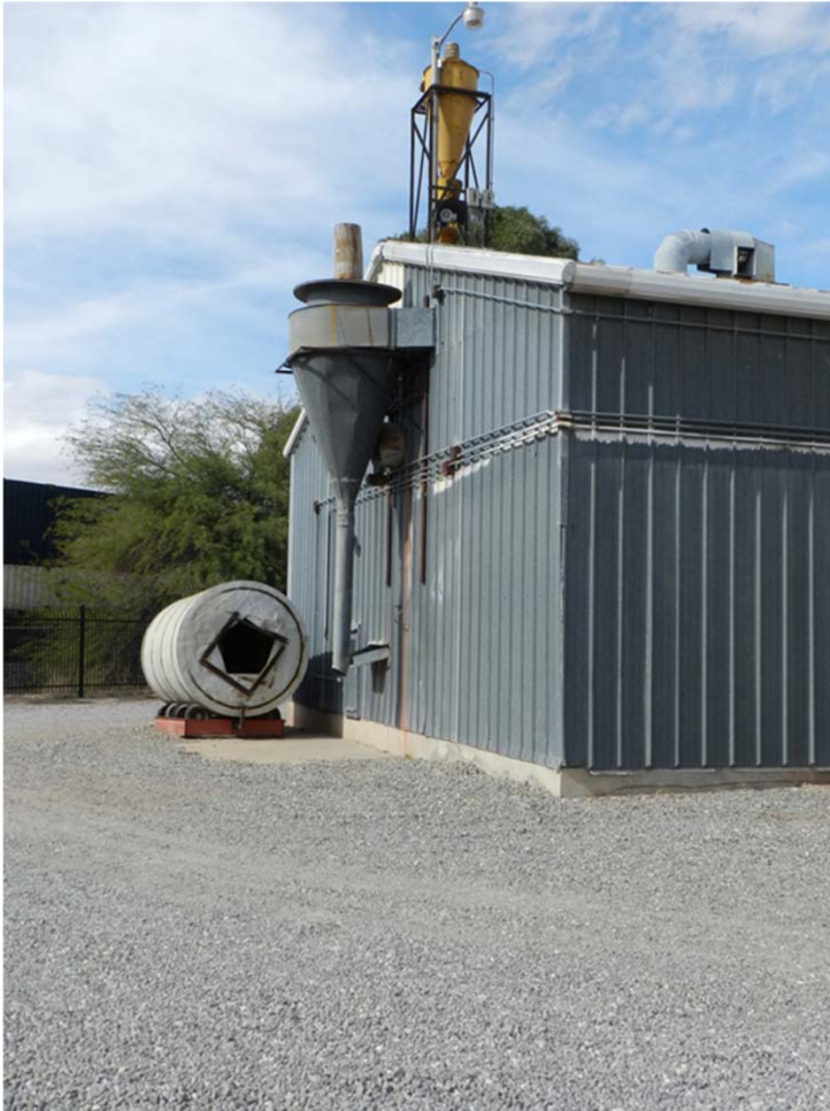
Figure 14: Seed Storage Building, looking west. Photo by: Caitlin Brown (2014).
