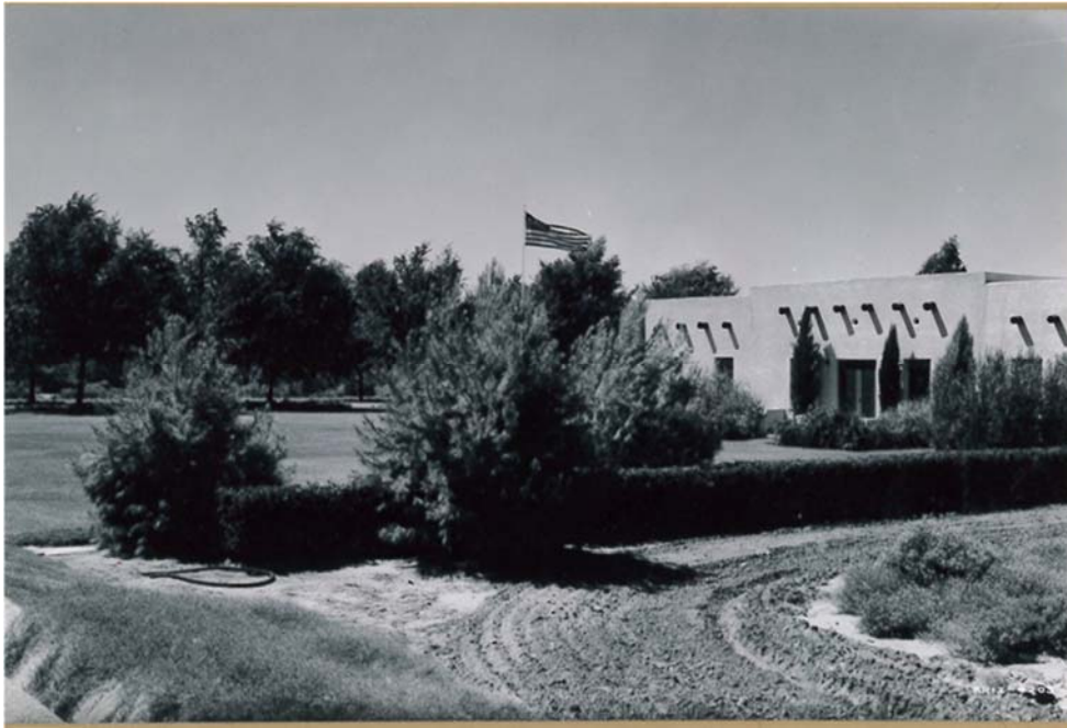
Figure 7: The headquarters with the Administrative Building looking southwest (unknown date). Photo Courtesy: Heather Dial (TPMC).
