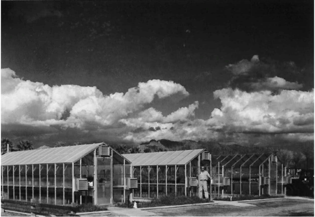
Figure 32: Greenhouses prior to demolition (unknown date). Photo Courtesy: Heather Dial (TPMC).
