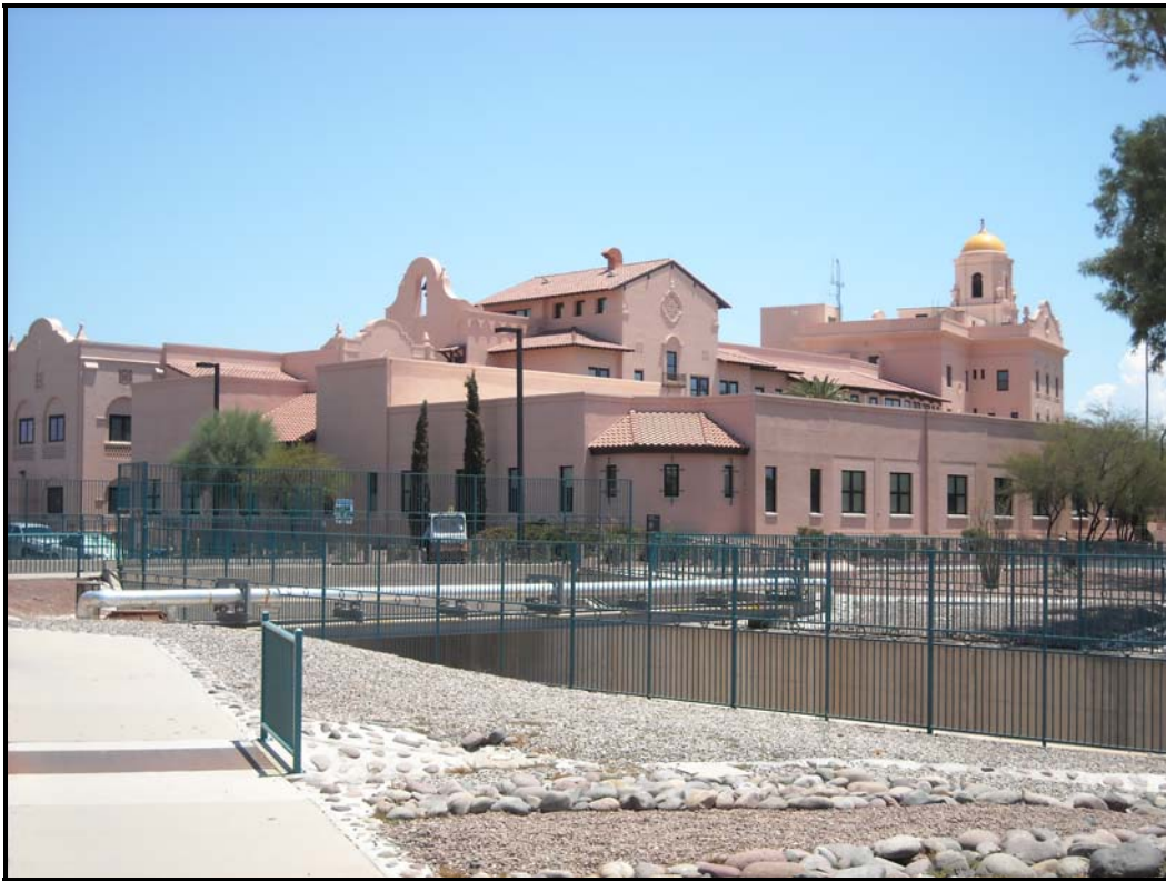
Photograph 25. Veteran's Administration Hospital No. 51, main building, view facing southeast (2010).
