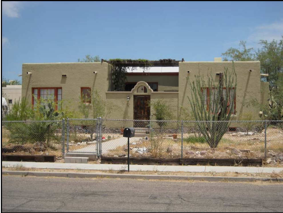
Photograph 9. Former superintendent's residence at St-Luke's-In-The-Desert, view facing north-northwest (2010).
