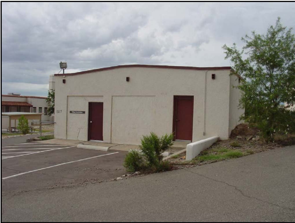
Photograph 43. Former garage (San Xavier-7), view facing east (2010).
