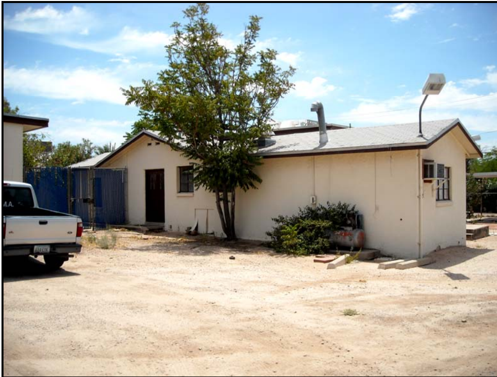
Photograph 6. Crippled Children's Ward, Comstock Children's Hospital, view facing southeast (2010).
