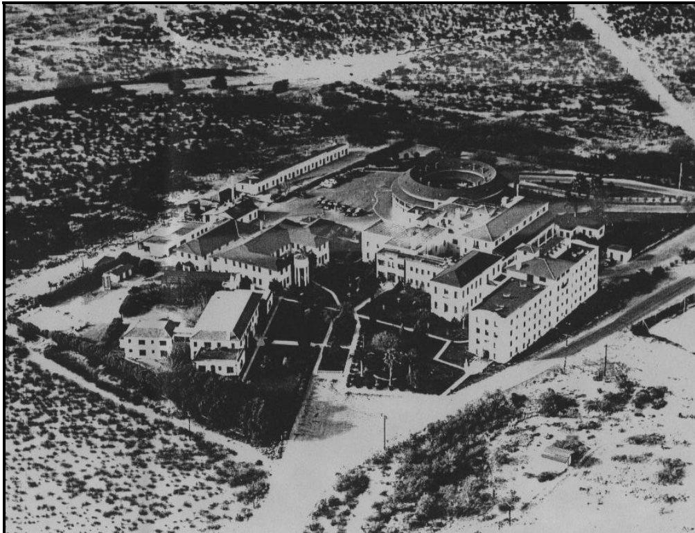
Photograph 2. Aerial photograph of St. Mary's Hospital, circa 1950, before the rotunda (sanatorium) was demolished (Photo No. MS 1251 ; courtesy of the Arizona Historical Society, Tucson).
