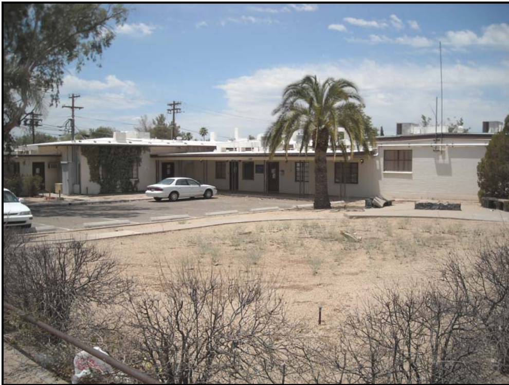
Photograph 5. Comstock Children's Hospital, main building, view facing southwest (2010).
