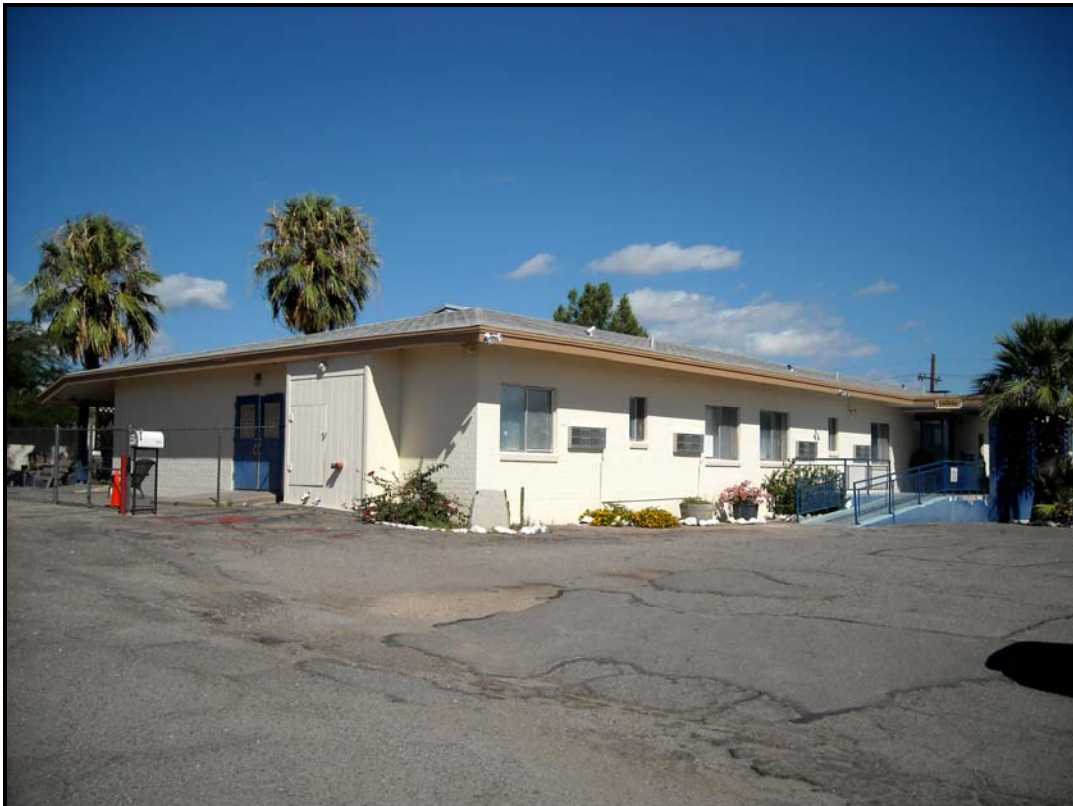
Photograph 56. Main hospital building at the former Arizona State Elk's Association Hospital, view facing northwest (2010).
