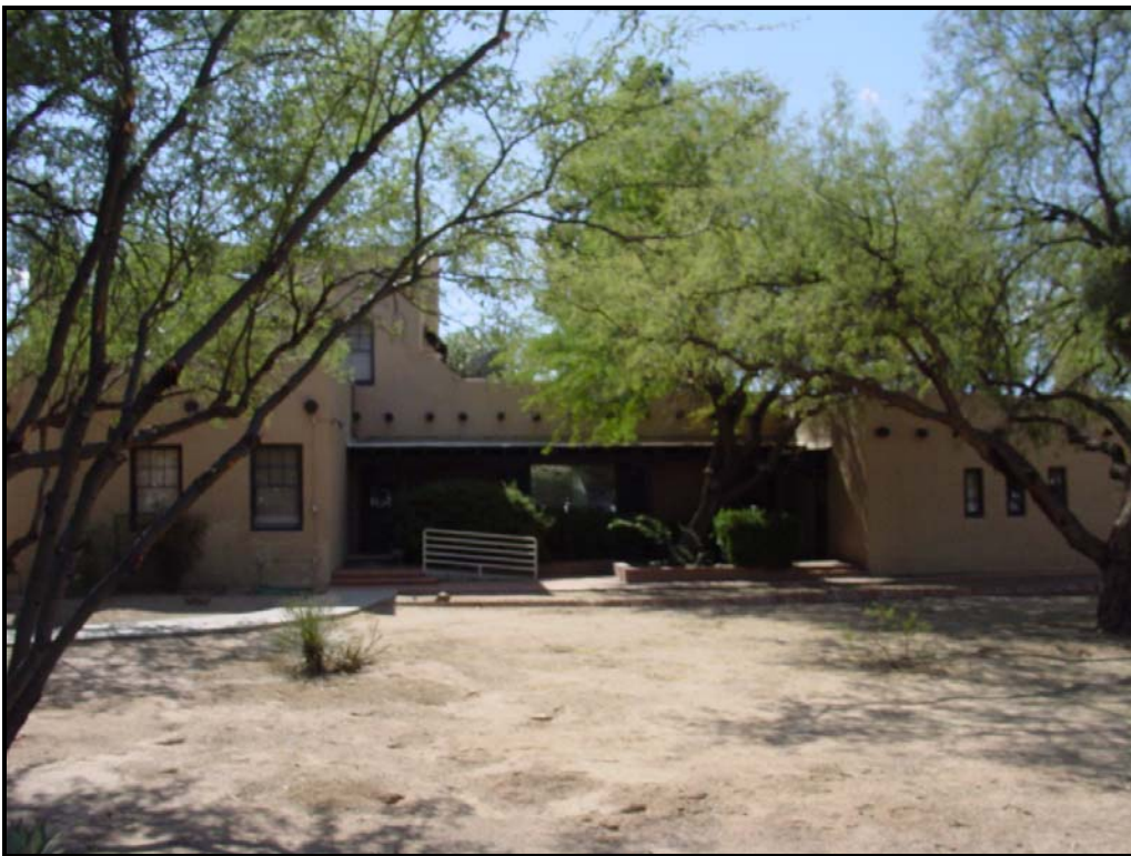
Photograph 22. North elevation of the Erickson Residence at the former Desert Sanatorium, view facing west (2010).
