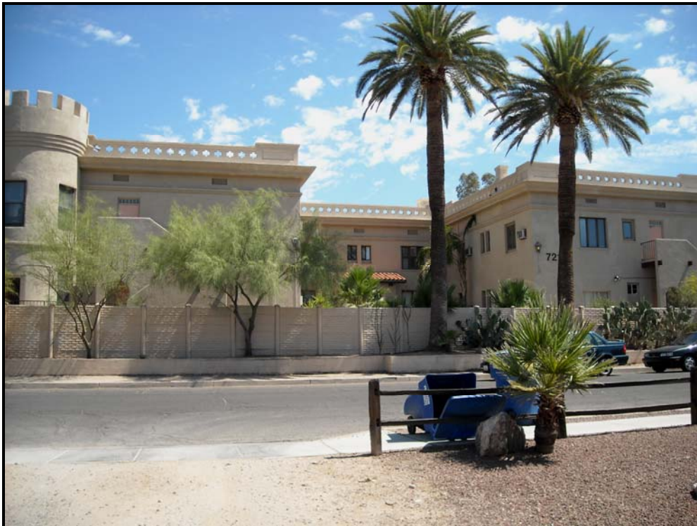
Photograph 3. Whitwell Hospital, now The Castle Apartments , view facing north-northeast (2010).
