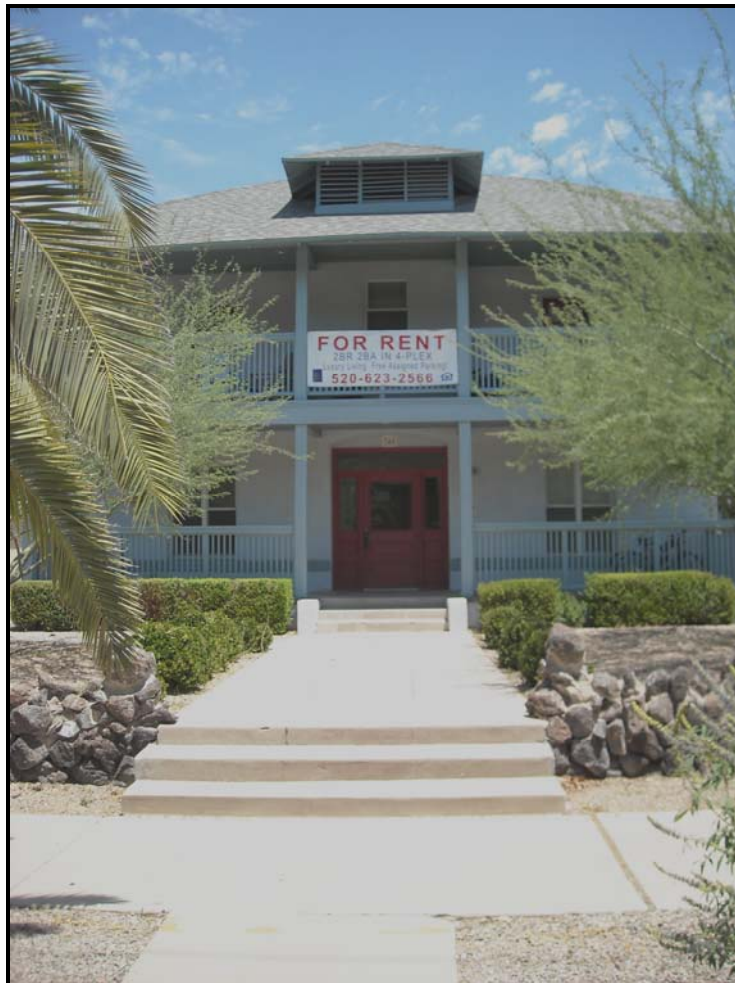
Photograph 13. Detail of south façade of Carter's Hotel Rest Sanatorium, view facing north (2010).
