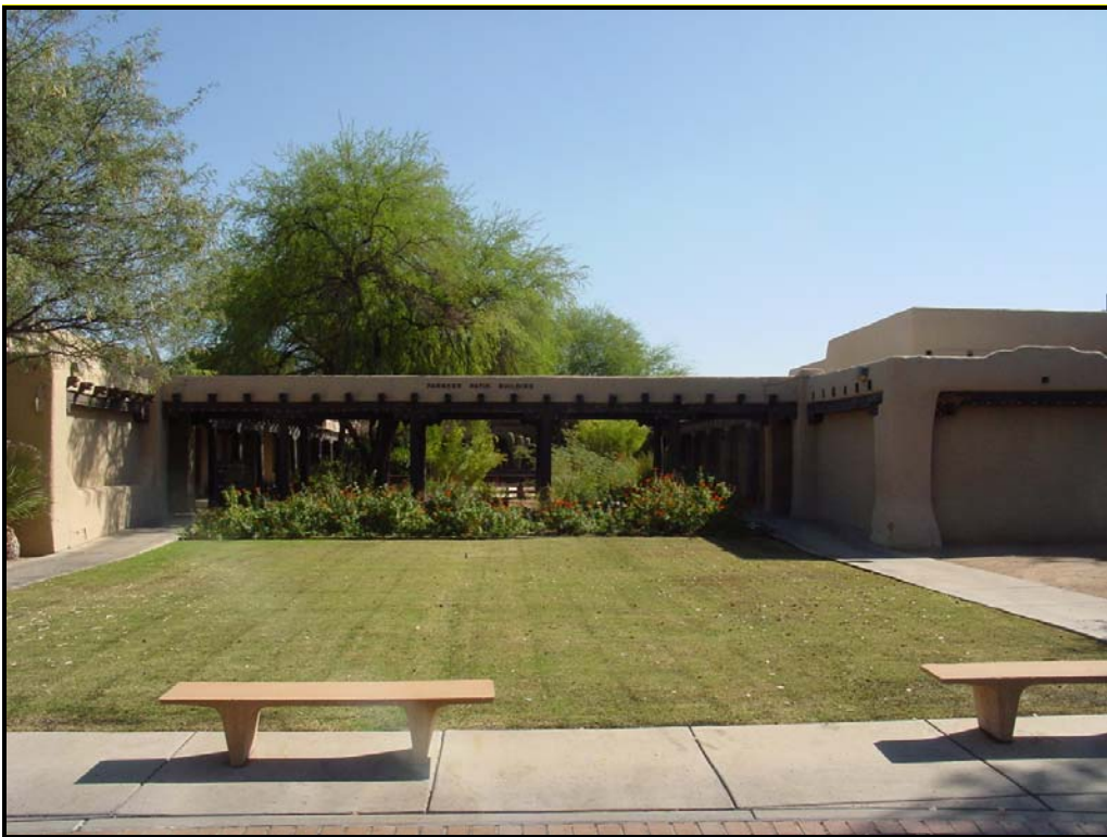
Photograph 15. West elevation of Patio Building (Institute of Medical Research) at the former Desert Sanatorium (now Tucson Medical Center), view facing east (2010).
