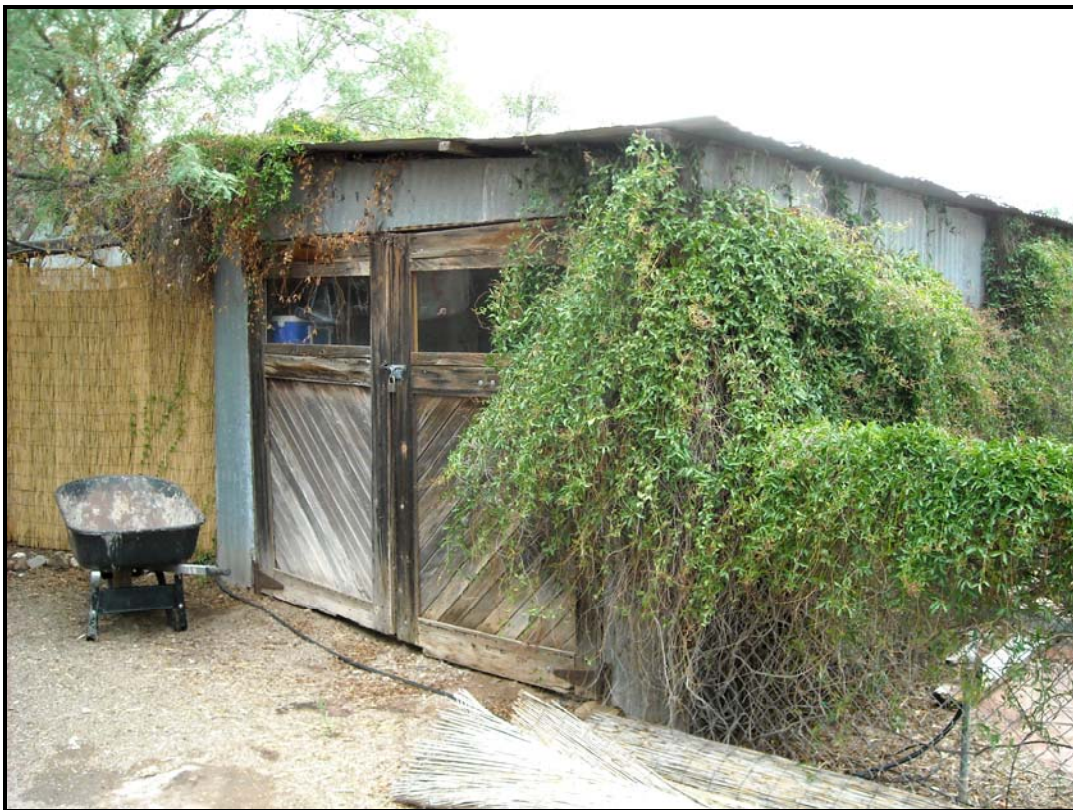
Photograph 52. Garage at former Owen Homesite, view facing southwest (2010).
