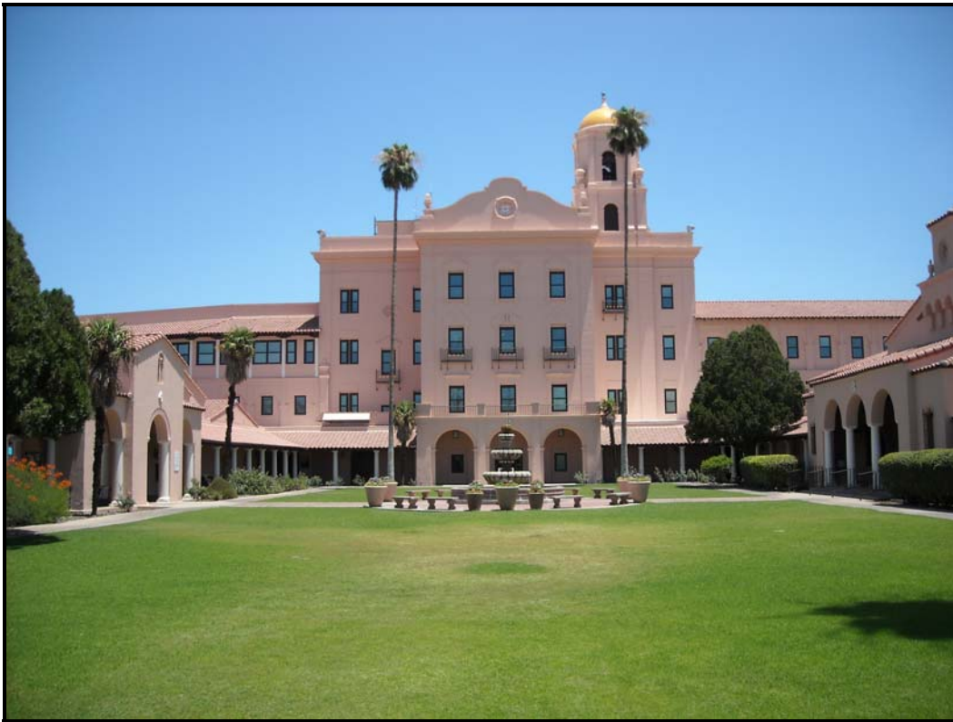
Photograph 26. Veteran's Administration Hospital No. 51, interior courtyard of main building, view facing east (2010).
