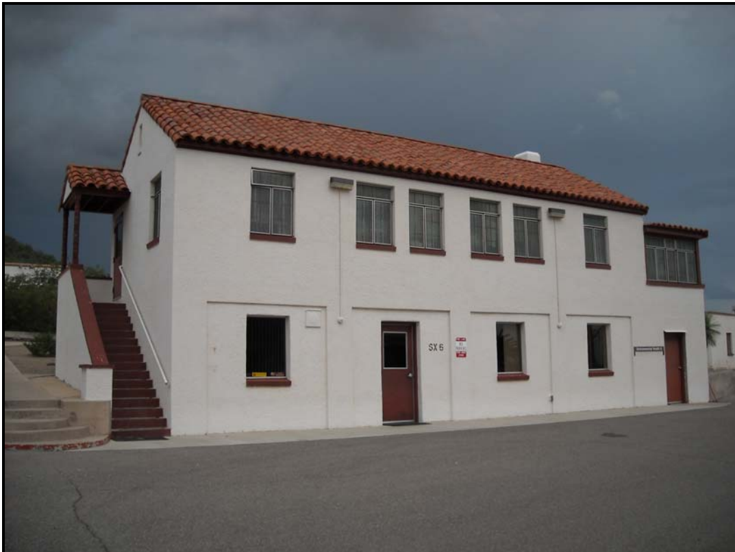
Photograph 42. Former nurse's residence (San Xavier-6), view facing west-northwest (2010).
