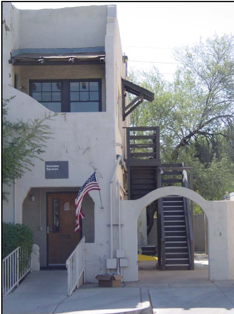
Photograph 19. Detail of northeast corner of the Arizona Building (Desert Sanatorium), view facing west (2010).
