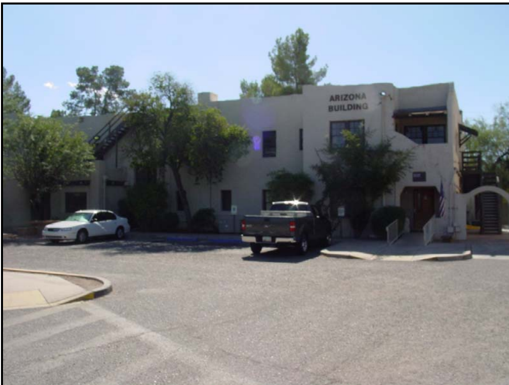
Photograph 18. East elevation of the Arizona Building (nurse's residence) at the former Desert Sanatorium (now Tucson Medical Center), view facing west-southwest (2010).
