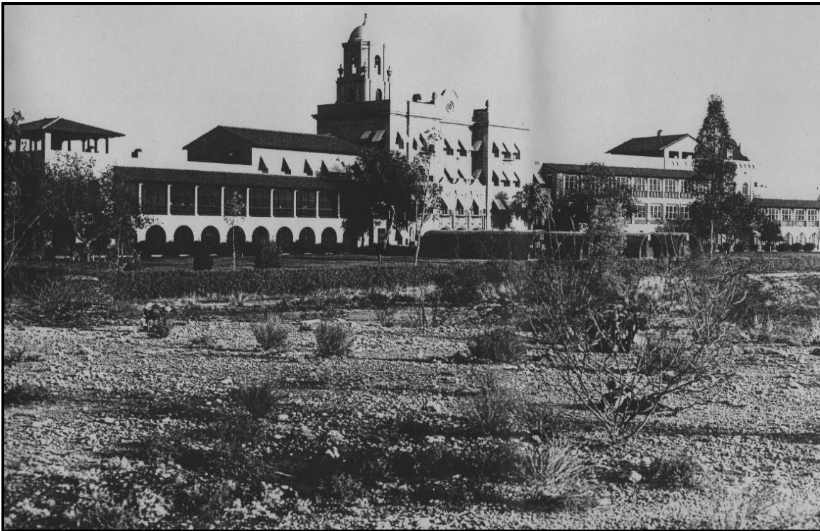
Photograph 31. Veteran's Administration Hospital No. 51, 1955 (Photo No. MS 1251, courtesy of Place and Place Architectural Collection, Arizona Historical Society, Tucson).
