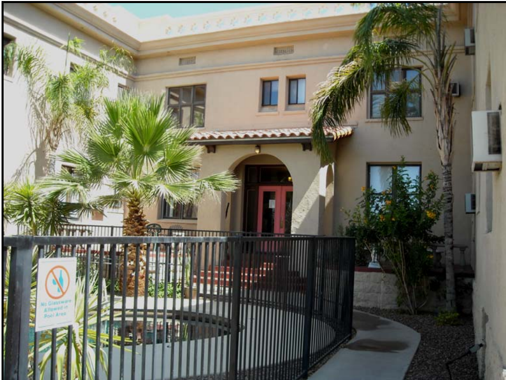
Photograph 4. Whitwell Hospital, entry and courtyard, view facing north (2010).
