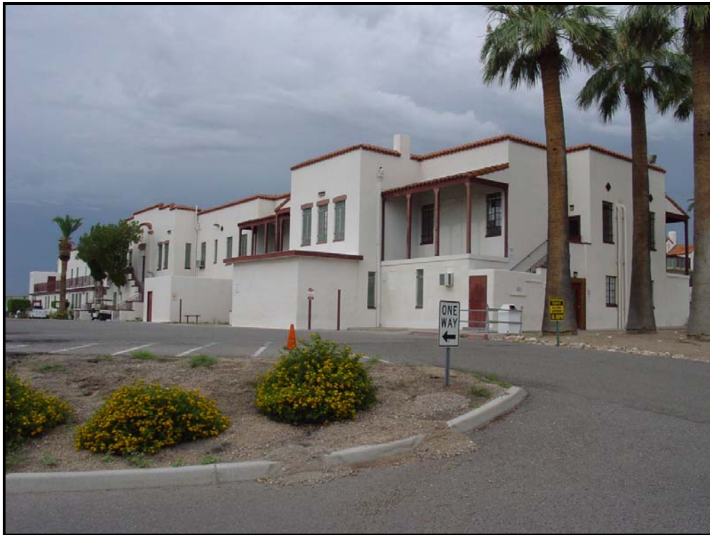
Photograph 37. Main hospital building (SX-1) at the former San Xavier Sanatorium, view facing southeast (2010).
