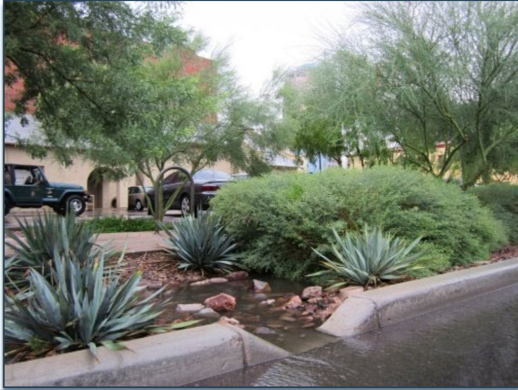
Figure 3.9. Type 2 Curb Opening for a new curb, Scott Ave. Source: Wheat Design Group.
