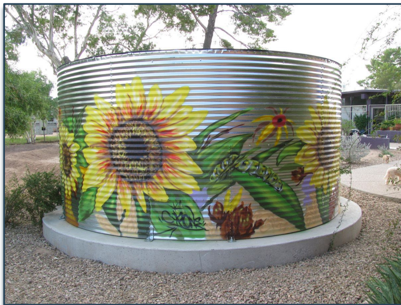
Figure 3.36. Metal cistern. Source: Southern Arizona Rain Gutters.
