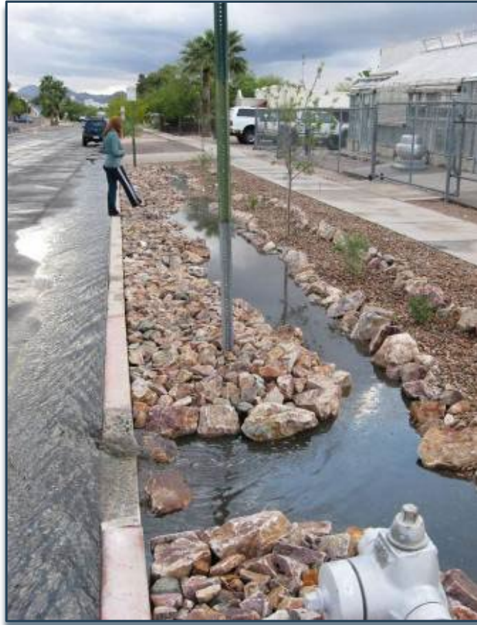
Figure 3.4. Rocked streetside stormwater harvesting basin. Source: Watershed Management Group
