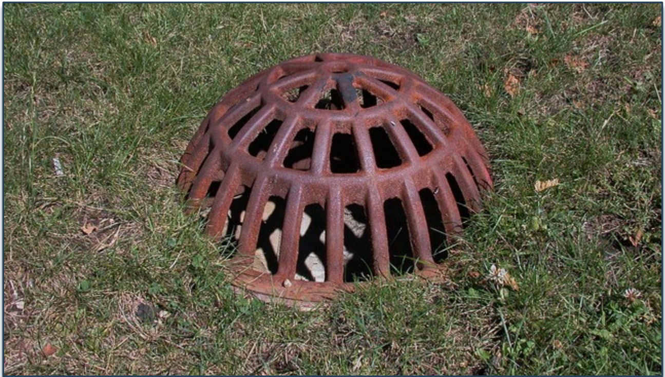
Figure 3.5. Dome overflow grate flush with the surface. Source: Aaron Volkening
