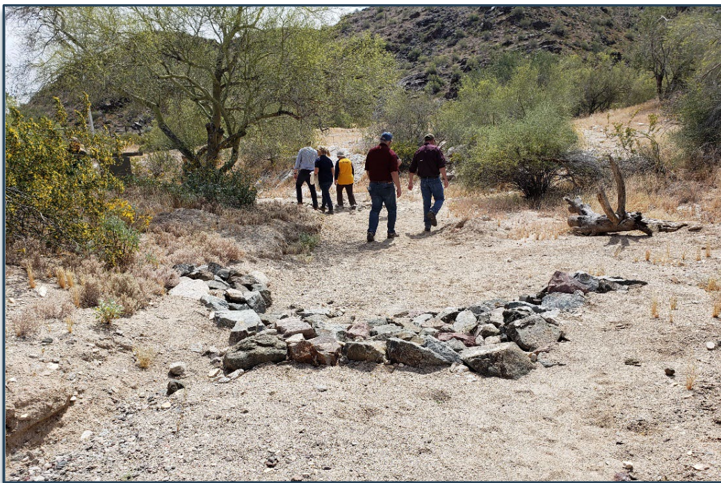
Figure 3.26. One Rock Dam. Source: Holistic Engineering and Land Management.
