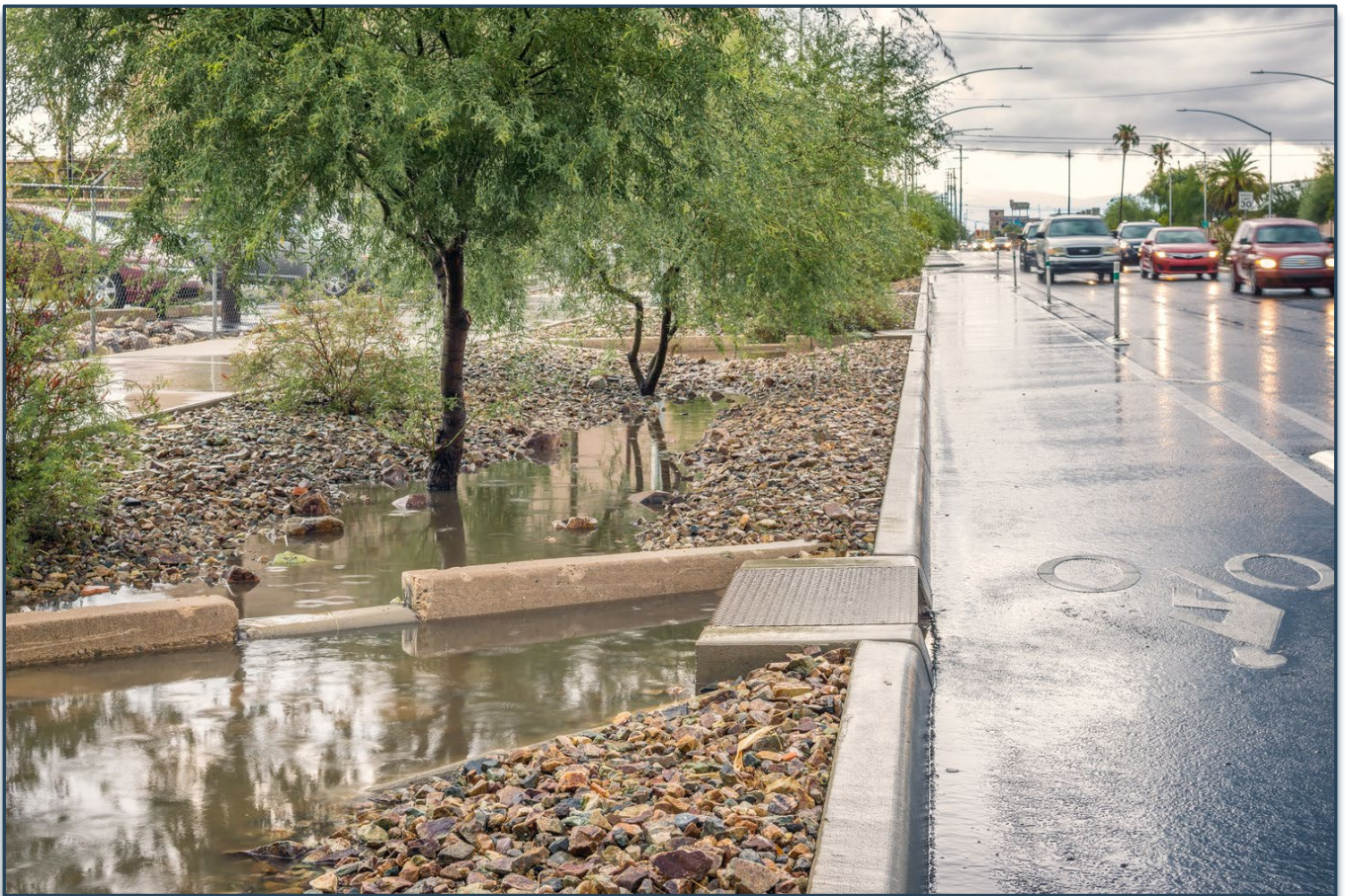
Figure 3.24. Saint Mary's Road concrete check dam. Source: Wheat Design Group.
