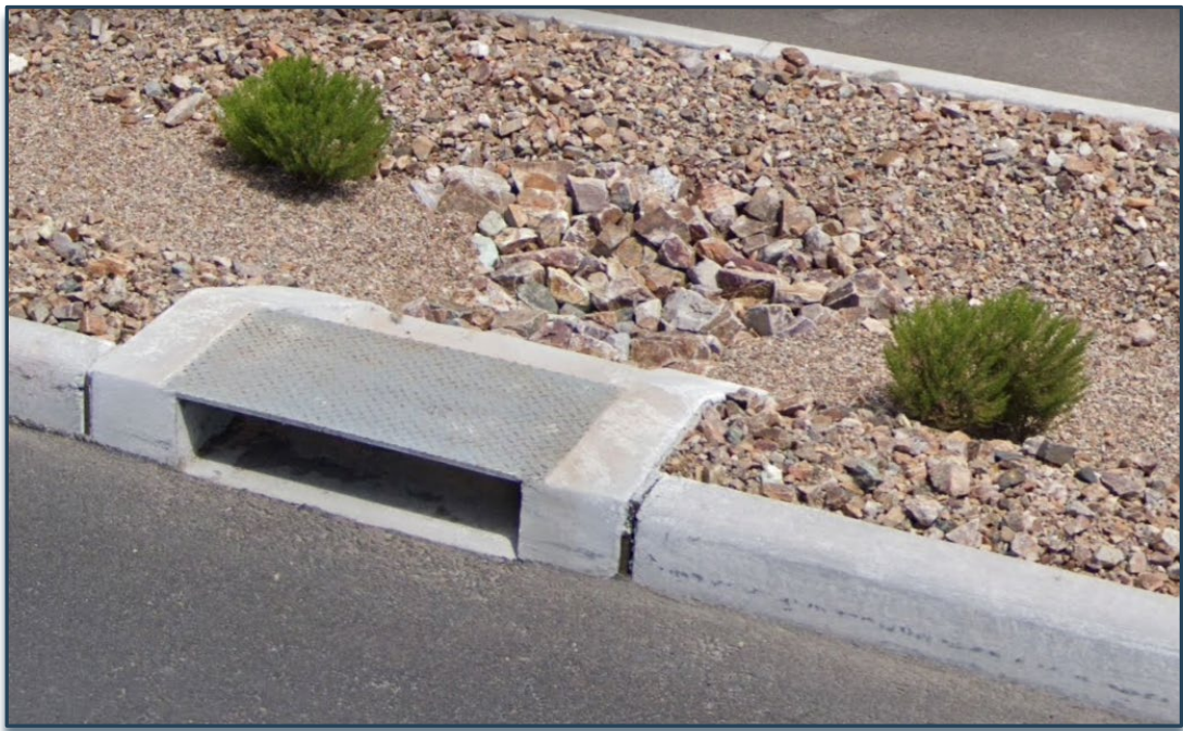
Figure 3.8. Curb opening Type 1, Grant Rd. Source: Google.
