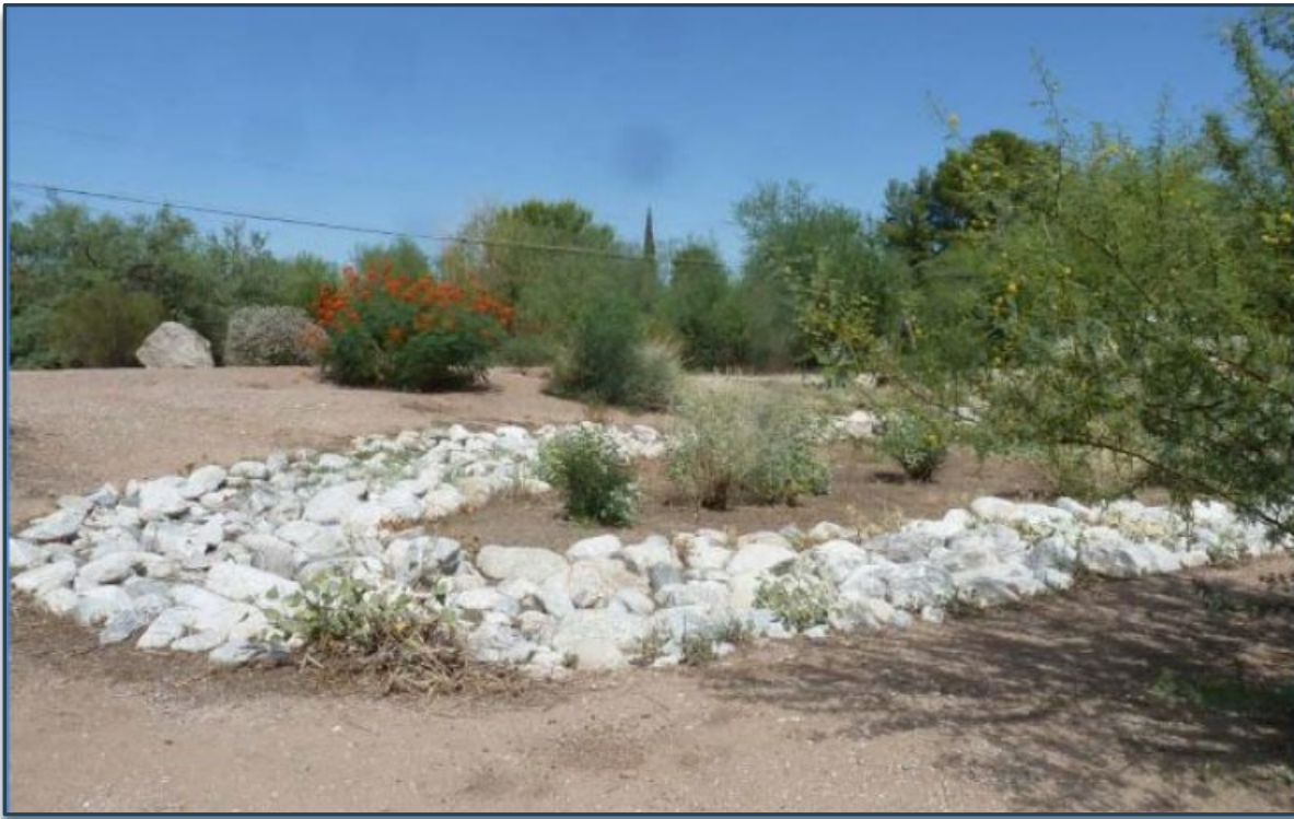
Figure 3.18. Infiltration trench. Source: Wheat Design Group.
