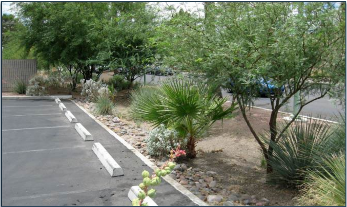
Figure 3.14. Flush curb at edge of asphalt parking lot. Source: Watershed Management Group.
