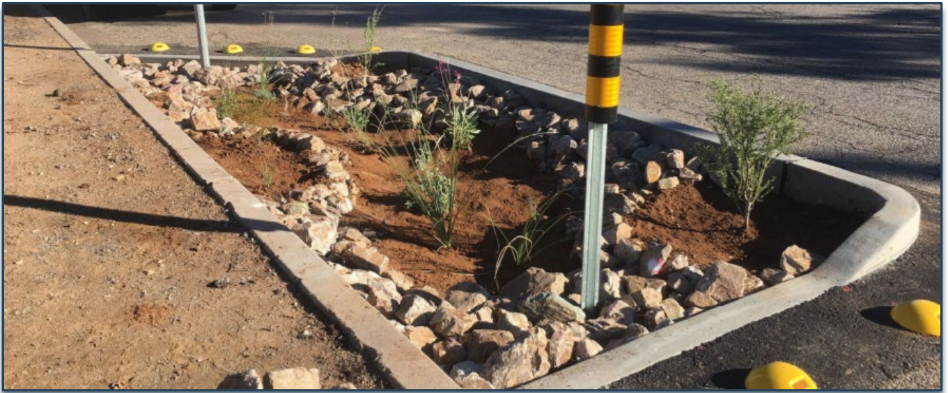
Figure 3.40. Newly planted chicane. Source: Tucson Clean and Beautiful.
