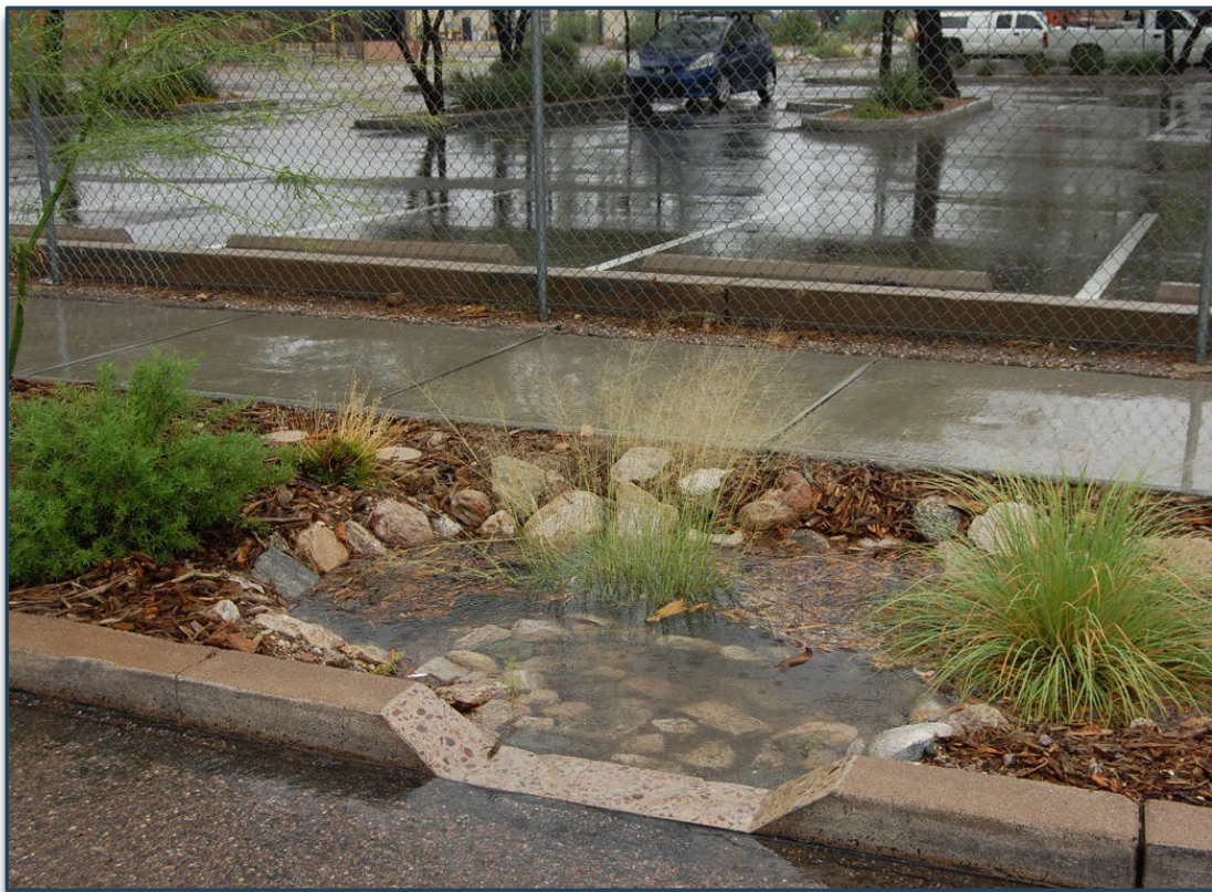
Figure 3.10. Type 2 curb retrofit, Tucson Association of Realtors. Source: Watershed Management Group.
