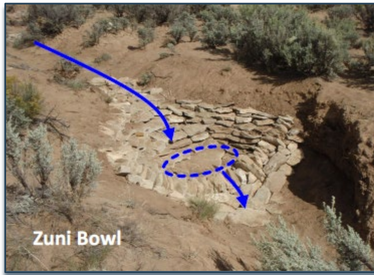
Figure 3.30. Photo of Zuni bowl showing flow path. Photo Credit: Quivira Coalition.
