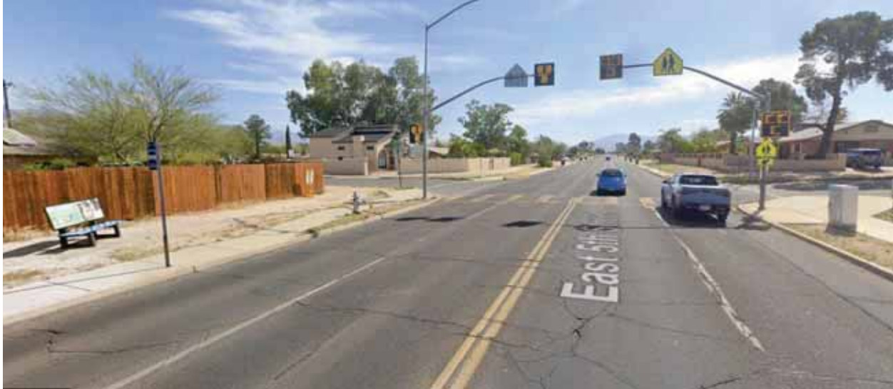
Figure 9. Irving Circle HAWK Crossing on 5th Street
