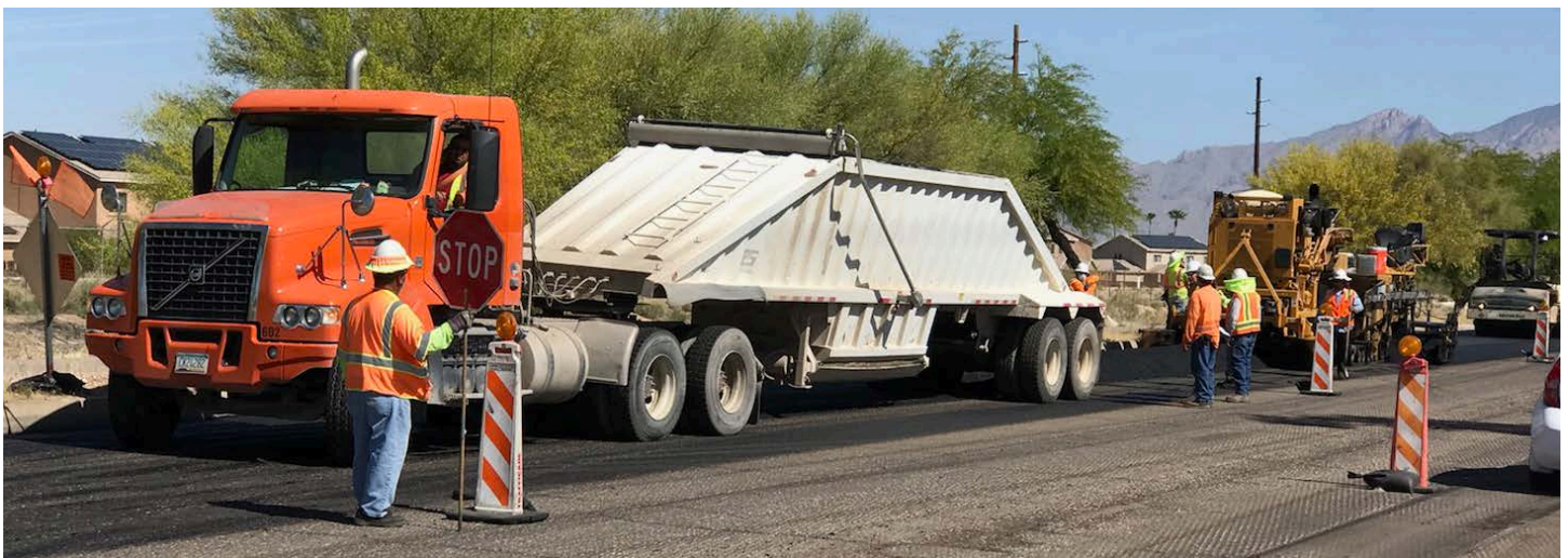
Asphalt paving is applied on Wilmot Road.
