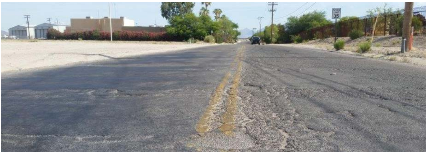
Plumer Avenue before repaving.
