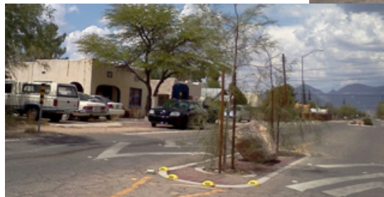
Combined speed hump with landscaped center median
