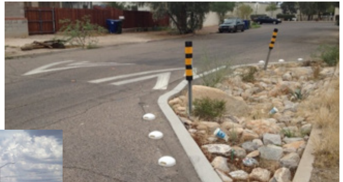
Combined speed hump with curb extension
