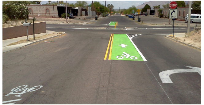
A median island/diverter on Glenn Street restricts through movements for cars while providing a refuge for cyclists traveling on the Fontana Bicycle Boulevard.
