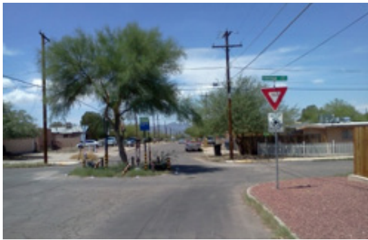
Traffic circles with yield signs slow motor vehicles and limit delay for cyclists.
