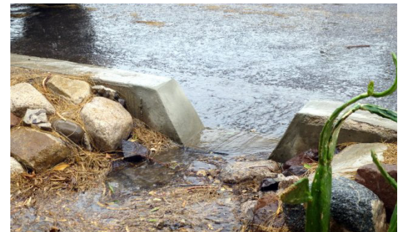
Curb cuts allow stormwater runoff to enter a landscaped basin in the public right of way (Photo credit: Watershed Management Group)
