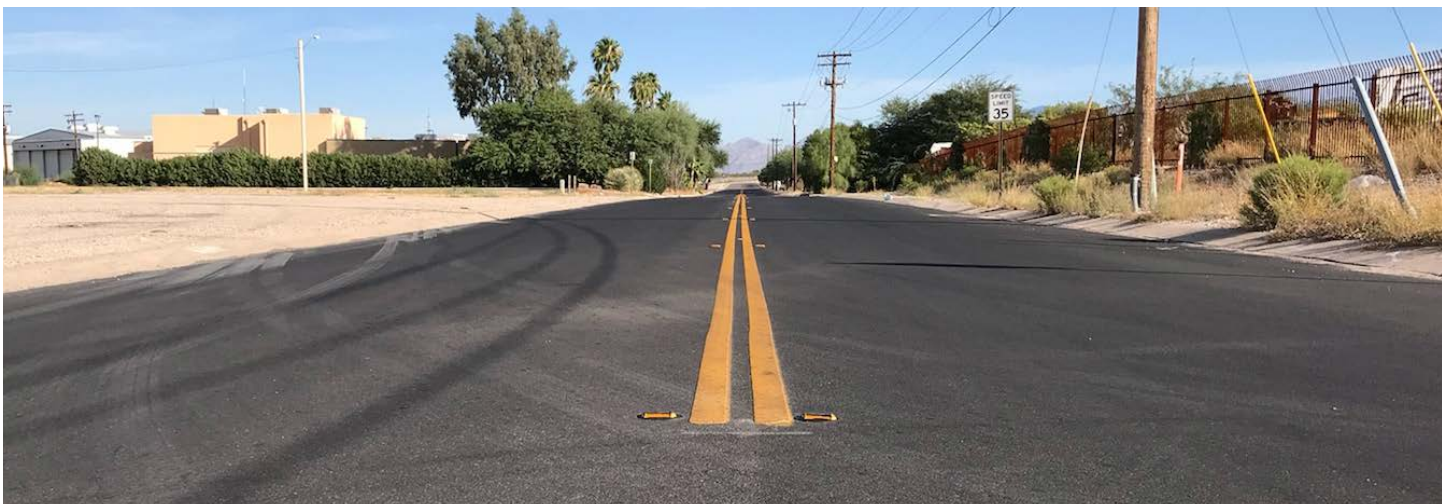
Plumer Avenue after repaving.
