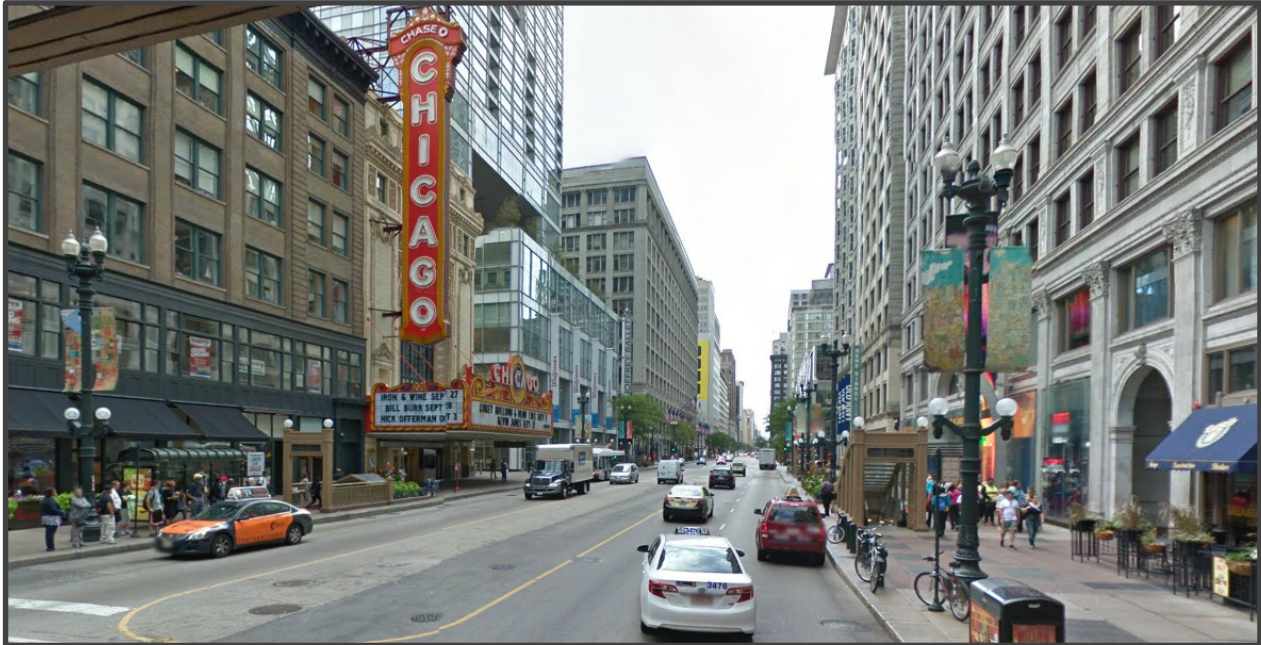
Figure 24. State Street – Street View (after reopening)
