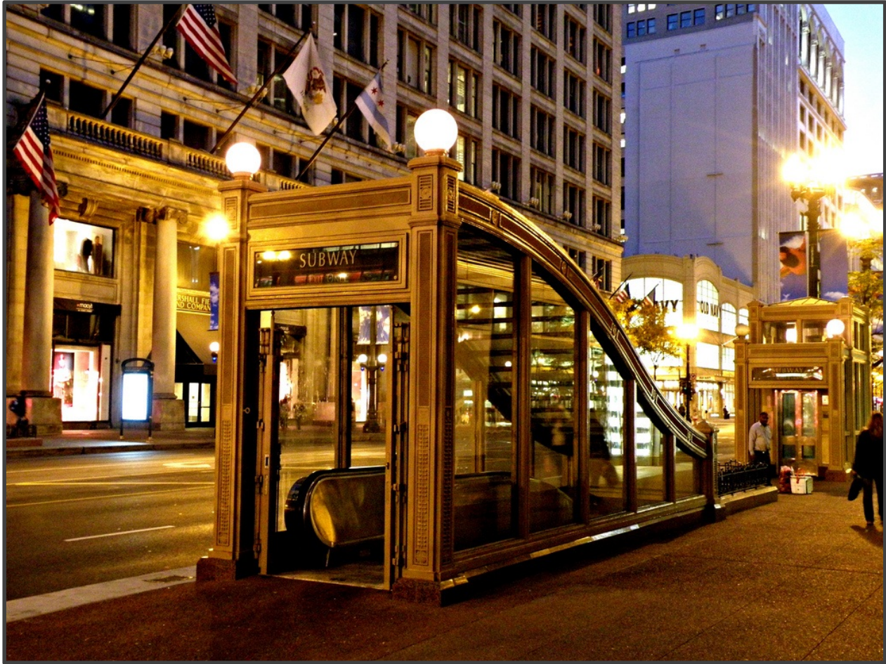
Figure 25. State Street – Subway Entrances
