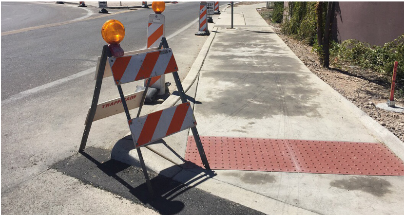
Image 5.2 A new curb ramp in downtown Tucson
