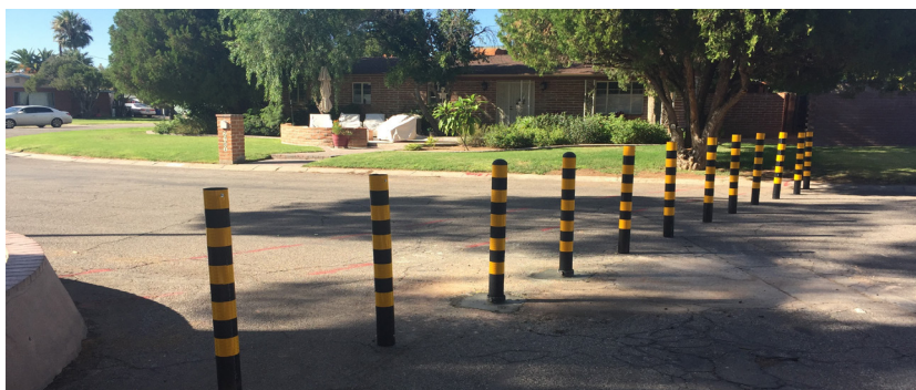
Image 4.31 and 4.32 A Half Closure (above) and Full Closure (below)
