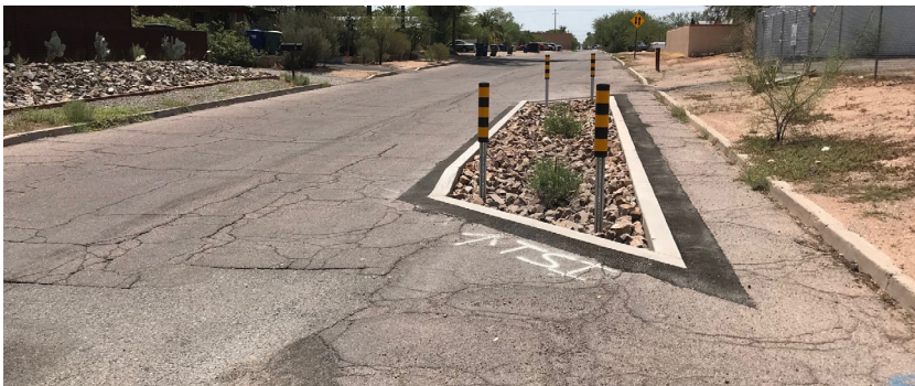
Image 4.24 A leftward Lateral Shift on a residential street in Tucson
