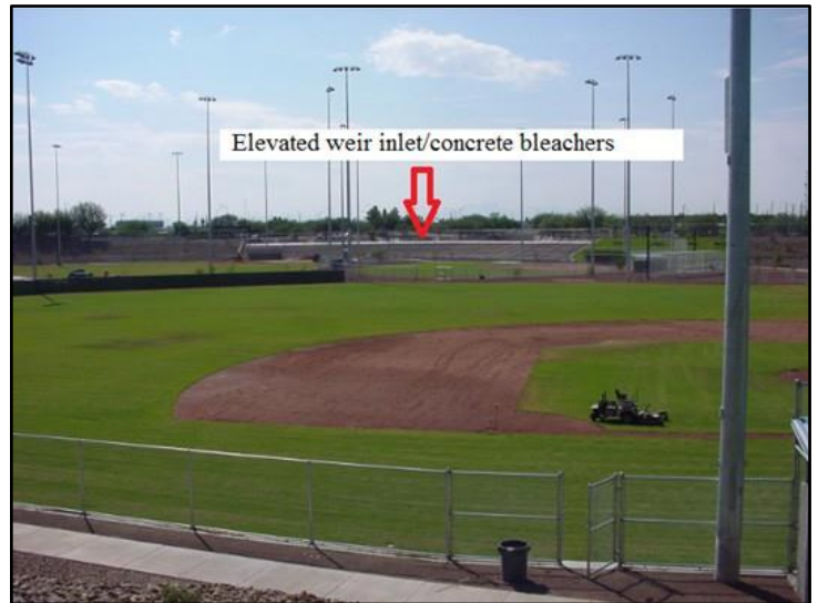
Figure 19: Phase 2A - Cherry Field basins are now a combination sports facility and flood control detention reservoirs maintained by Pima County.
