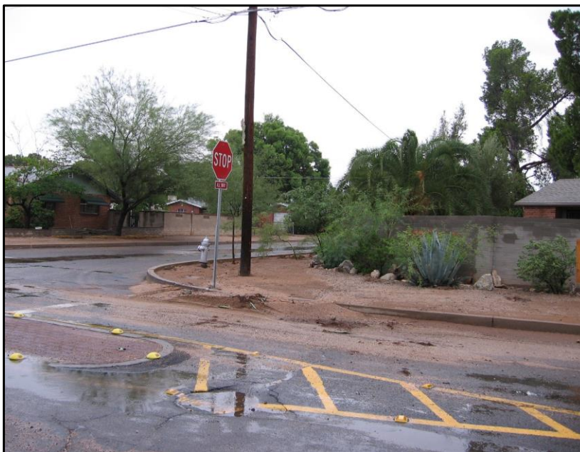
Figure 15. Erosion in right-of-way.
