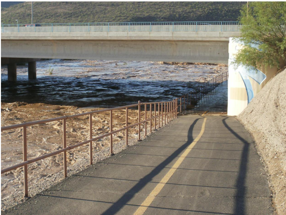
Figure 27: Santa Cruz River Bike Lane Underpass – flooded
