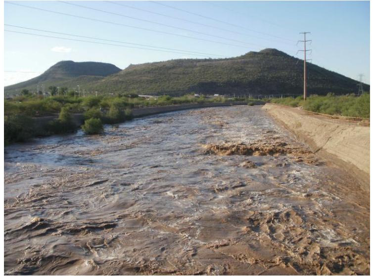
Figure 8: Santa Cruz River bank protection
