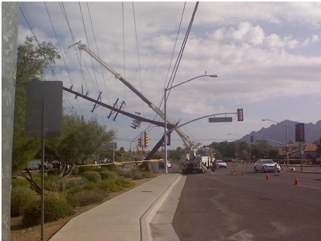
Figure 6: Downed power lines along Oracle Road following a storm event
