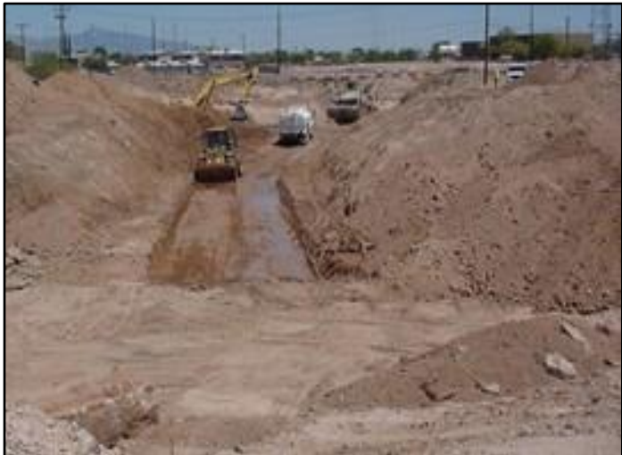
Figure 20: Phase 2B - Park Avenue Basin 2 Under Construction
