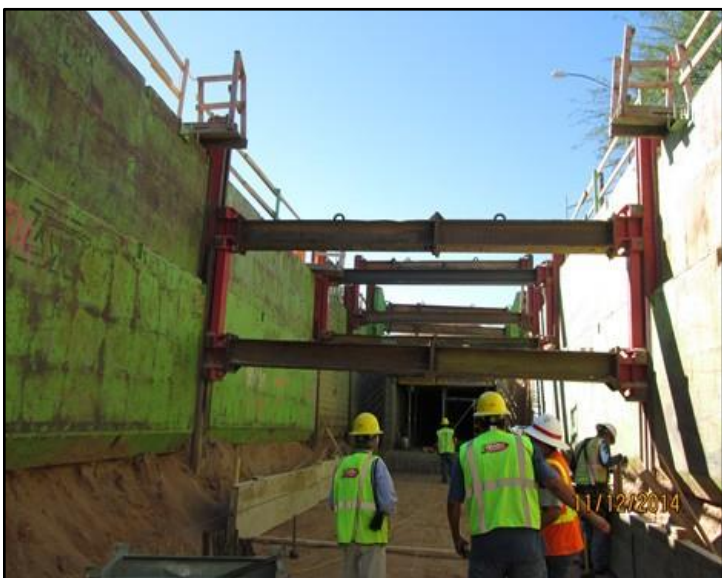
Figure 22: Construction of High School Wash storm drain
