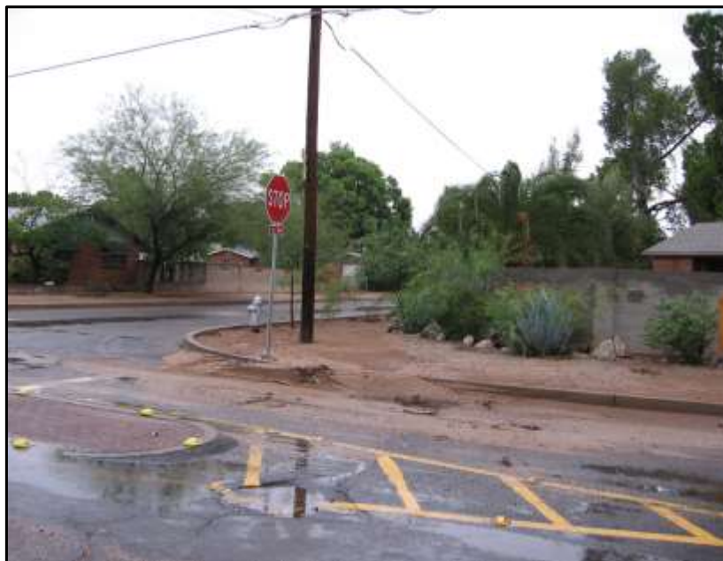
Figure 21: Erosion in right-of-way.
