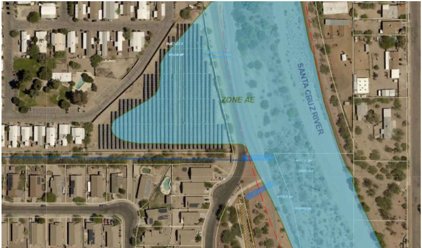
Figure 12: Solar infrastructure in HOA common area is elevated above the overbank waters of the Santa Cruz River for the reduction of electrical costs to this manufactured home subdivision community.
