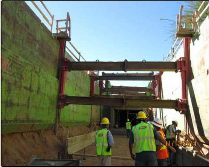
Figure 29: Construction of High School Wash storm drain
