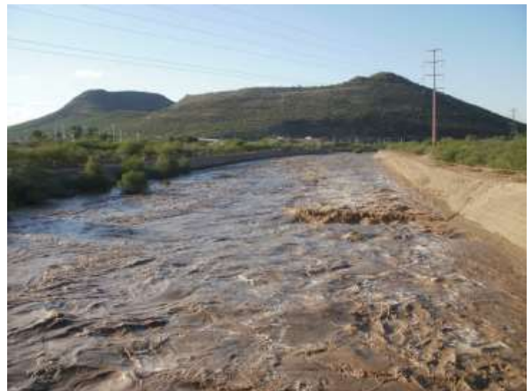
Figure 11: Santa Cruz River bank protection
