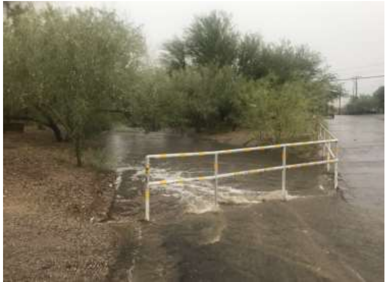
Figure 37: Streets are part of the urban stormdrain system (J. Hayt)
