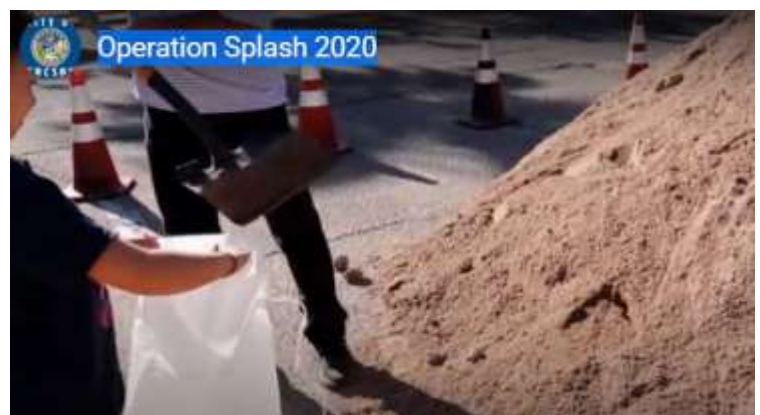
Figure 54: Sandbagging is an easy and cost-effective technique to battle flooding
