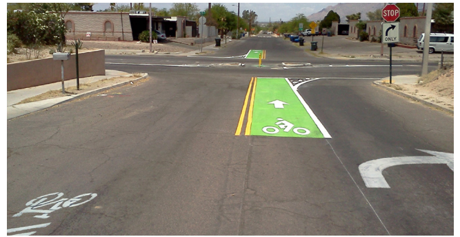
A median island/diverter on Glenn Street restricts through movements for cars while providing a refuge for cyclists traveling on the Fontana Bicycle Boulevard.
