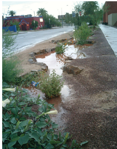
A landscaped basin along Park Avenue captures water during a storm (Photo credit: Watershed Management Group)
