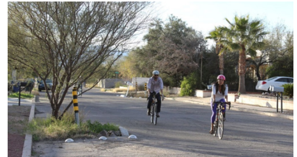
Landscaped curb extension on Elm Street collects stormwater after a rain
