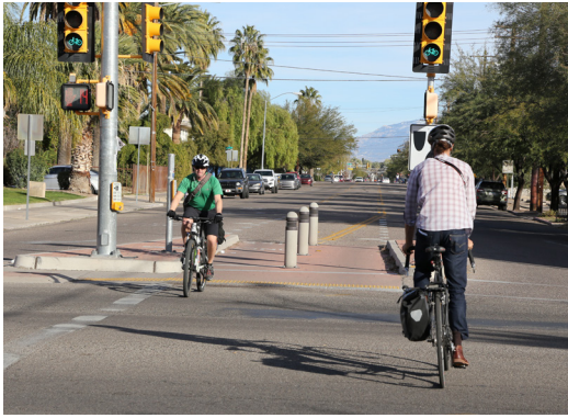
Bicycle and Pedestrian signalized crossing (TOUCAN) on the Third Street/University Bicycle Boulevard at Stone Avenue.
