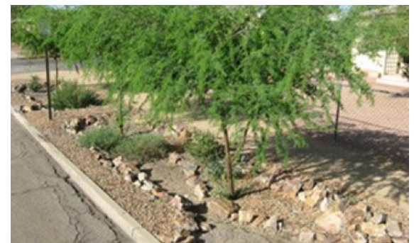
A curb cut and bioswale captures stormwater while native trees provide shade for cyclists and pedestrians.
