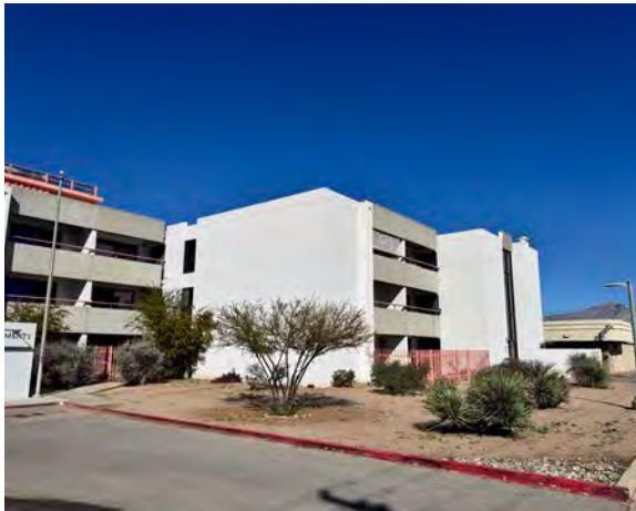
View of the northeast portion of the Craycroft Towers (1635 North Craycroft Road).
