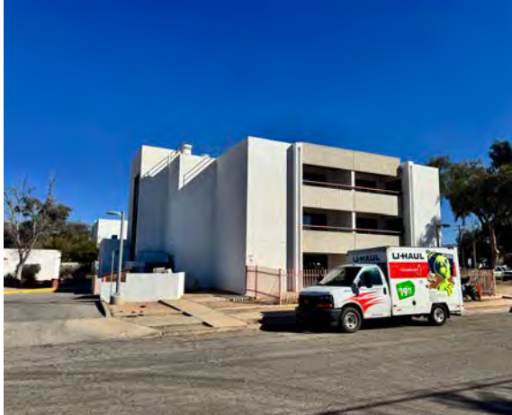
View north of Craycroft Towers (1635 North Craycroft Road) from East Lee Street.
