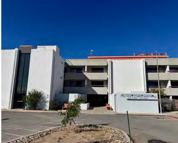
View of Craycroft Towers (1635 North Craycroft Road).
