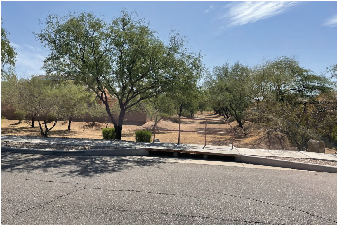
Southern detention basis (facing east), easterly flow to detention basin
