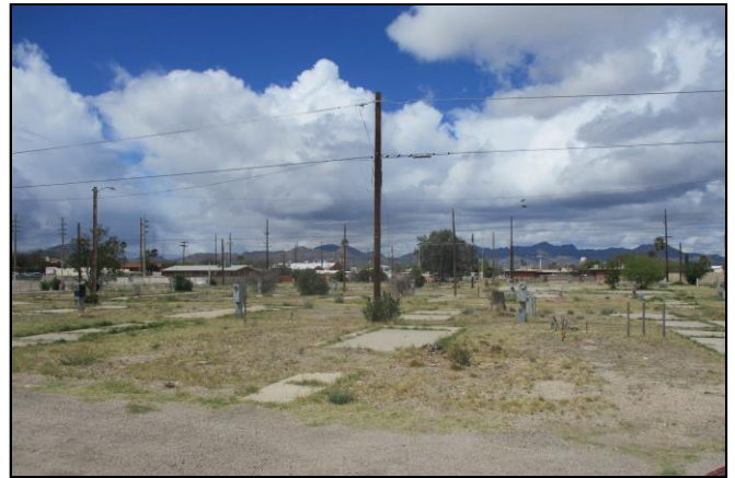
Picture 16 – View of typical concrete slabs throughout the Property.
