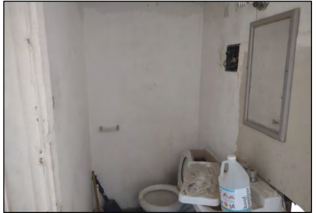
4: Interior of the on-site office building
