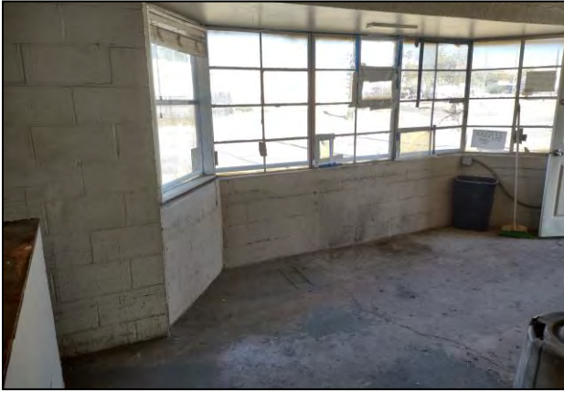
1: Interior of the on-site office building
