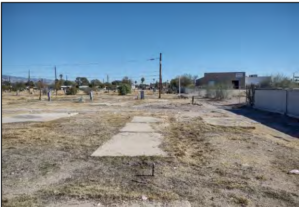
5: View of exterior concrete foundations
