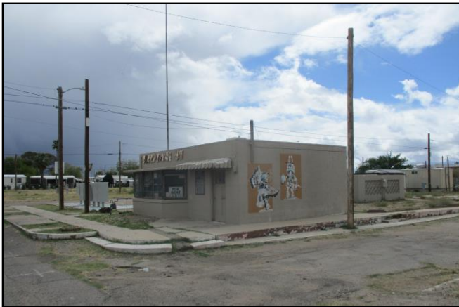
Picture 15 – View of the “office” building at the north side of the Property.
