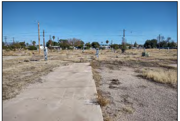
6: View of exterior concrete foundations
