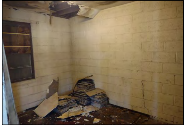
2: Interior of the on-site office building
