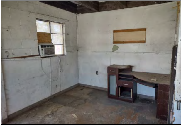
3: Interior of the on-site office building
