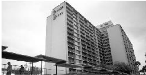
Tucson House, Tucson's largest public housing site
