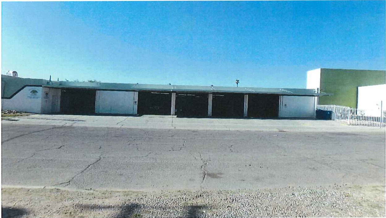
331 E Adams Street to be demolished, north face
