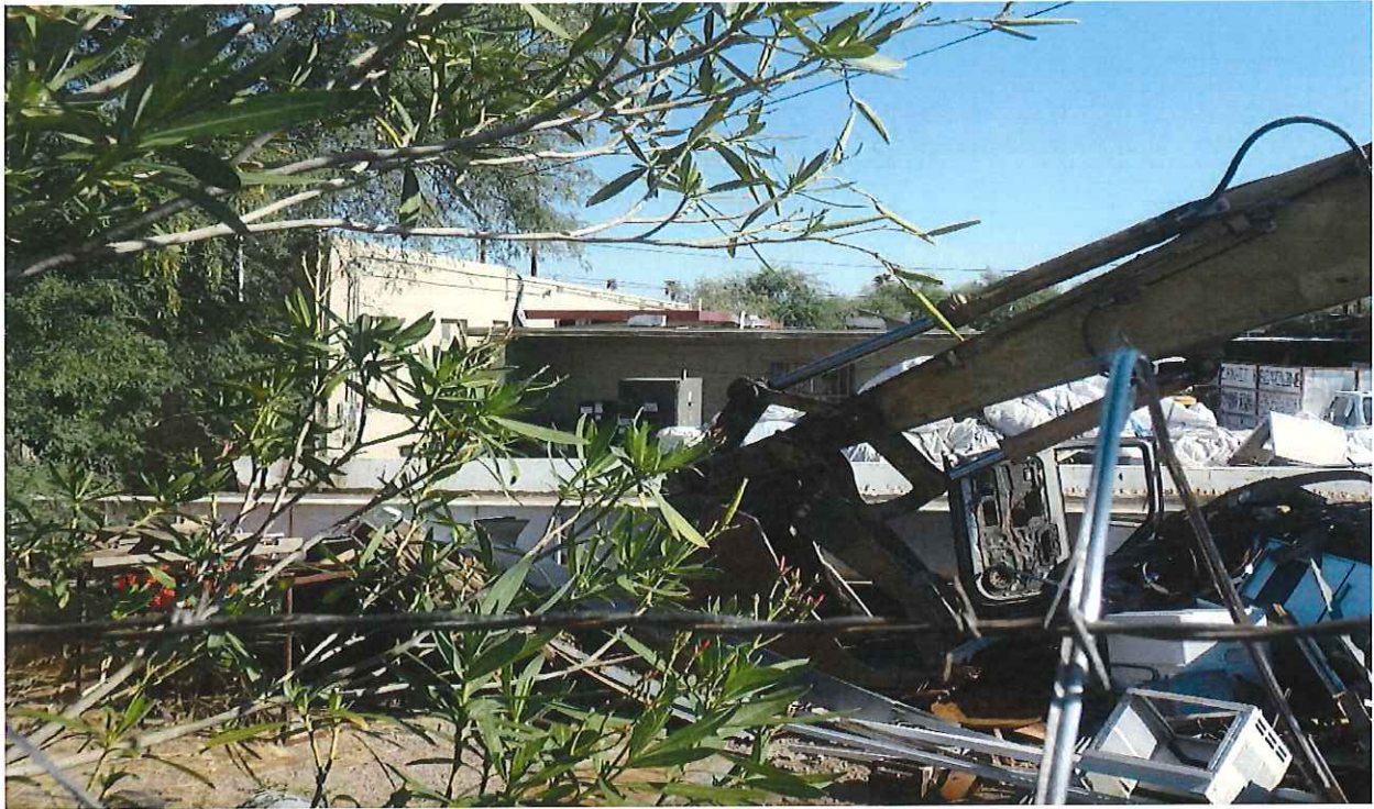
1435 N. 11 th Avenue, CAN-IT Recycling to be demolished
