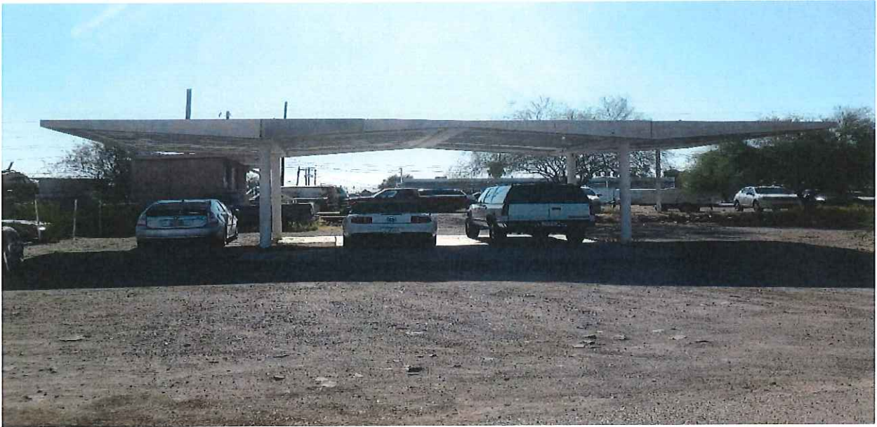
Parking cover to be demolished
