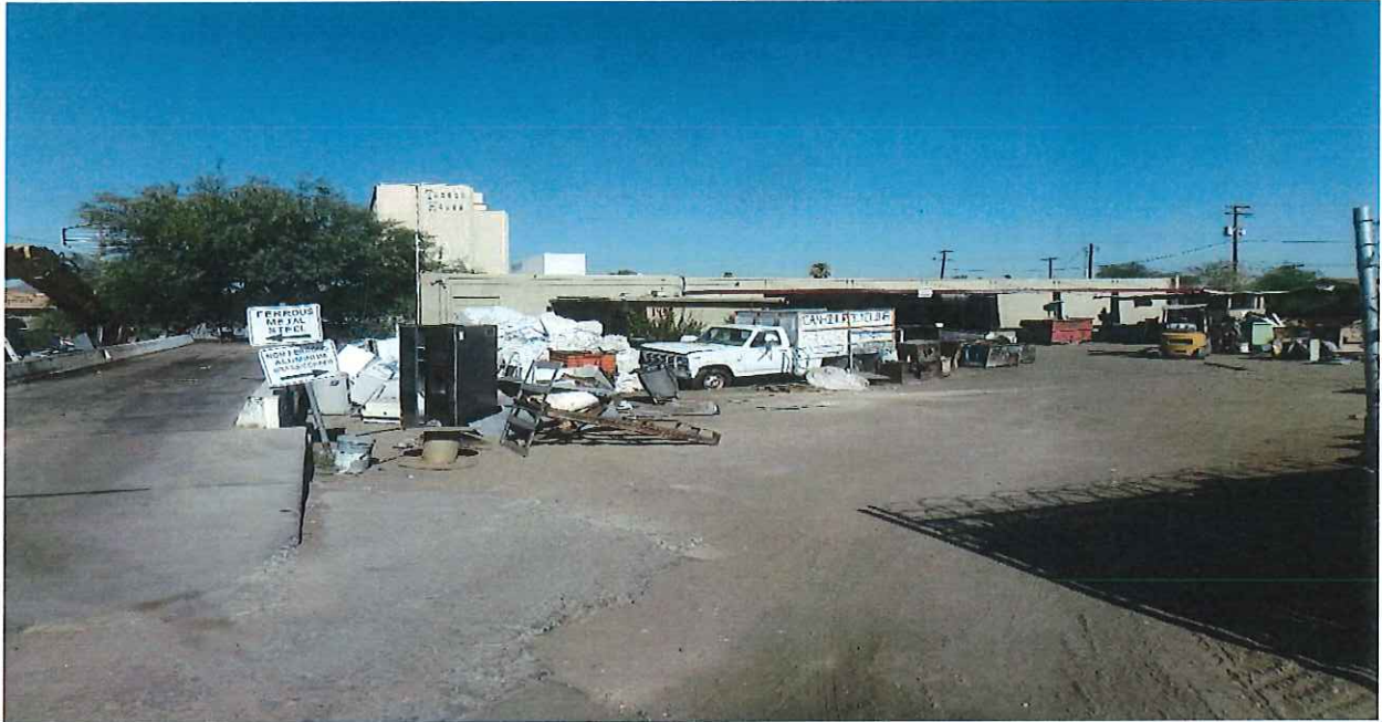
1435 N. 11 th Avenue, CAN-IT Recycling to be demolished
