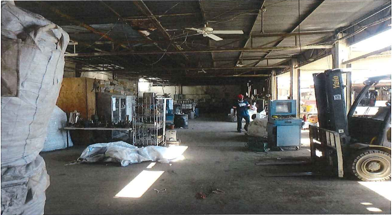
1435 N. 11 th Avenue, CAN-IT Recycling to be demolished
