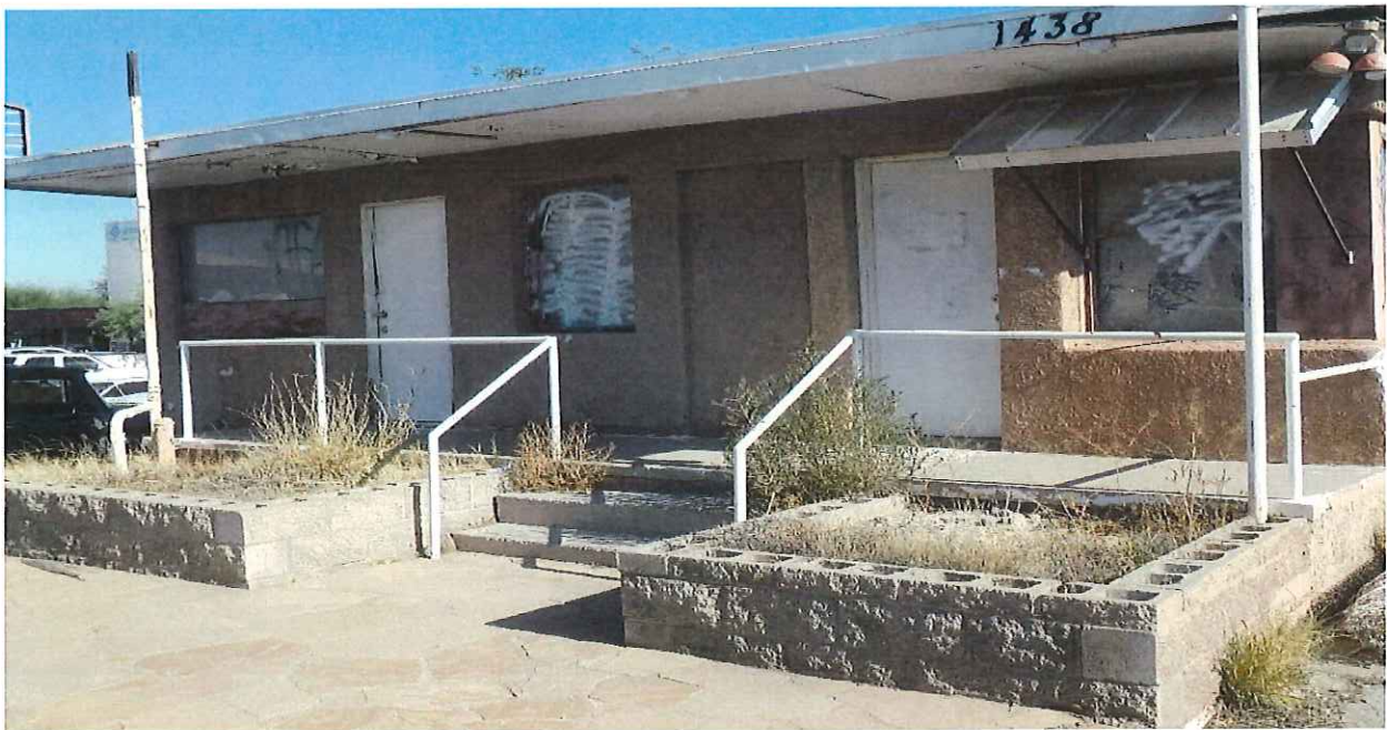
1438 N. 11 th Avenue to be demolished
