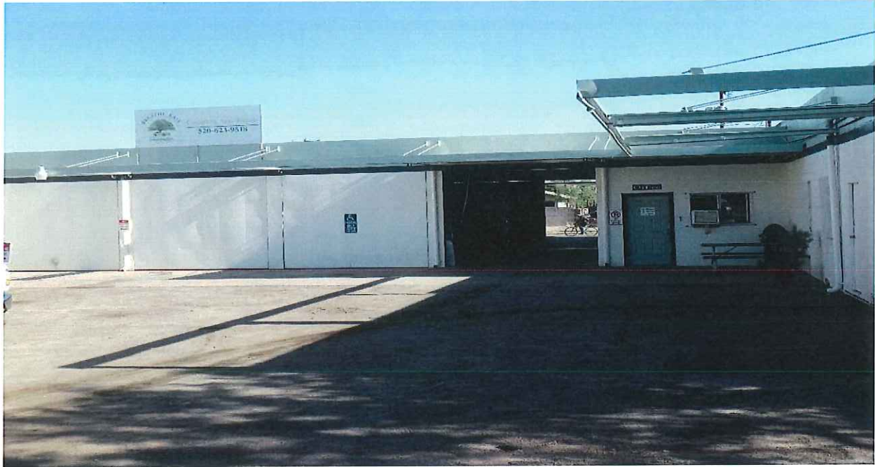
331 E Adams Street to be demolished, south face
