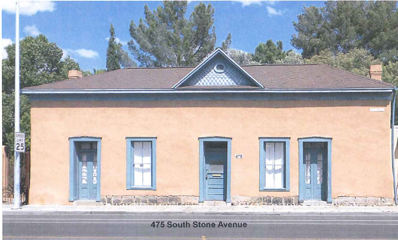
475 S. STONE AVE. VELASCO OFFICE BLDG - ARMORY PARK
