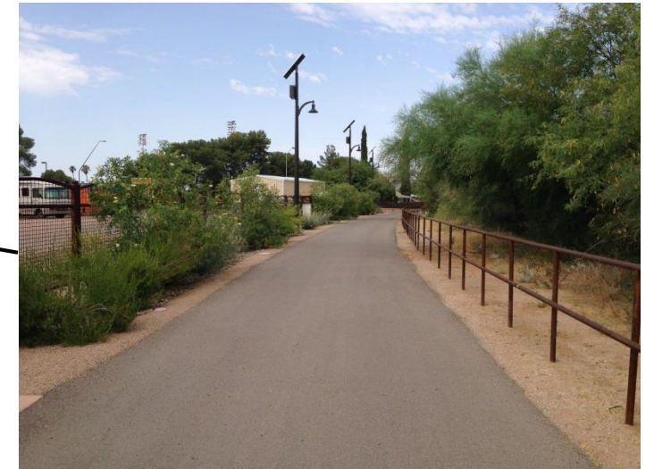
S Tucson Boulevard to Parkway Terrace
