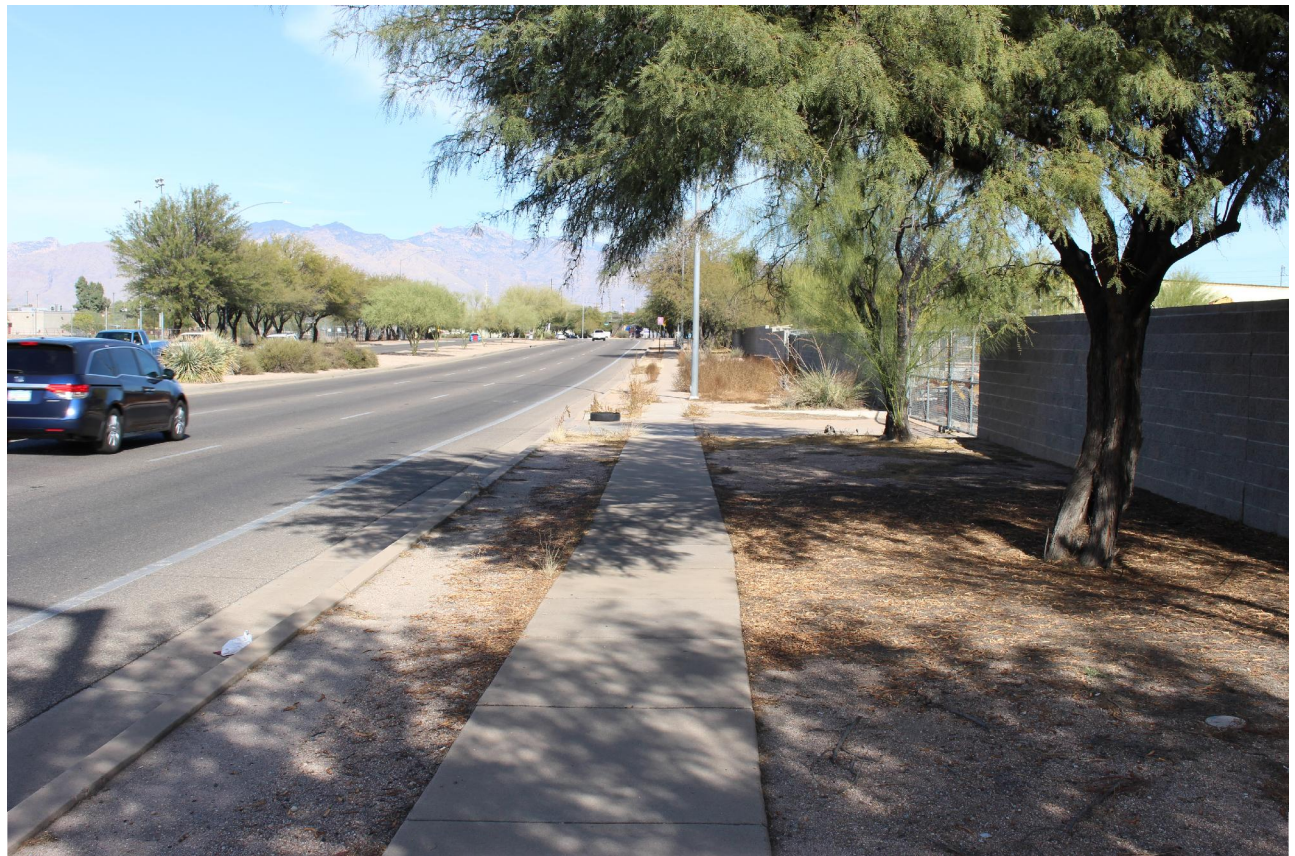
BEFORE - KINO PKWY. LOOKING NORTH
