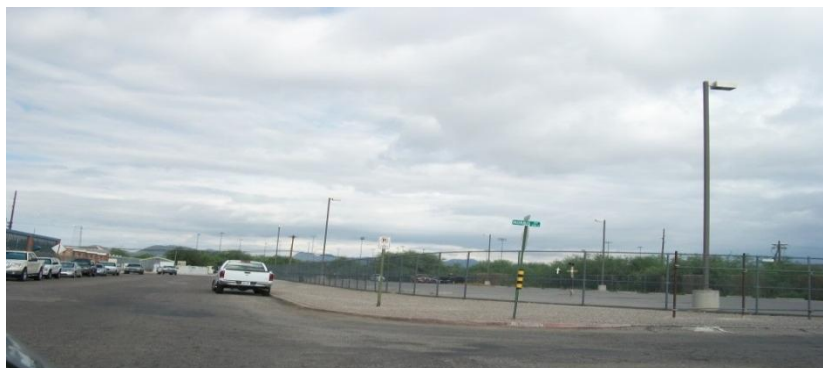
TUSD Parking Lot (looking west on 15 th St.)
