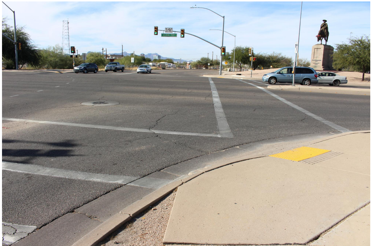
BEFORE - INTERSECTION OF 15TH ST. AND KINO PKWY. LOOKING WEST
