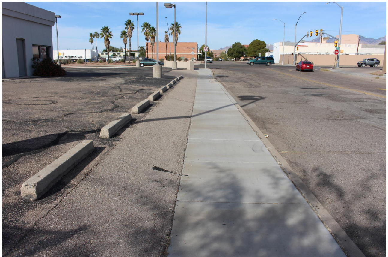
BEFORE - PARK AVE. LOOKING NORTH
