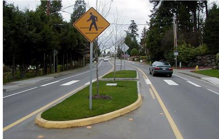
Example of a median island crossing on a two-lane street with a center turn lane.
