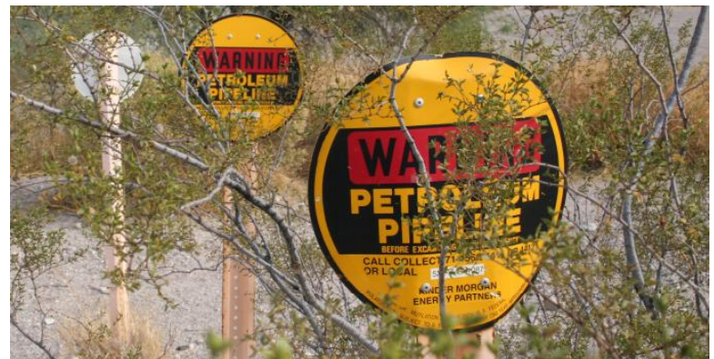
Natural Gas Line Along the Greenway Alignment
