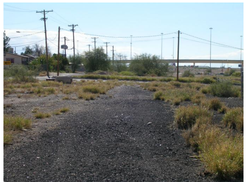
Past Railroad Use Creates Potential Environmental Issues that Must be Addressed During Design
