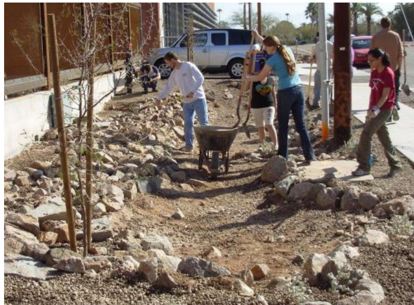
Rock edging along swale edges prevents erosion.
