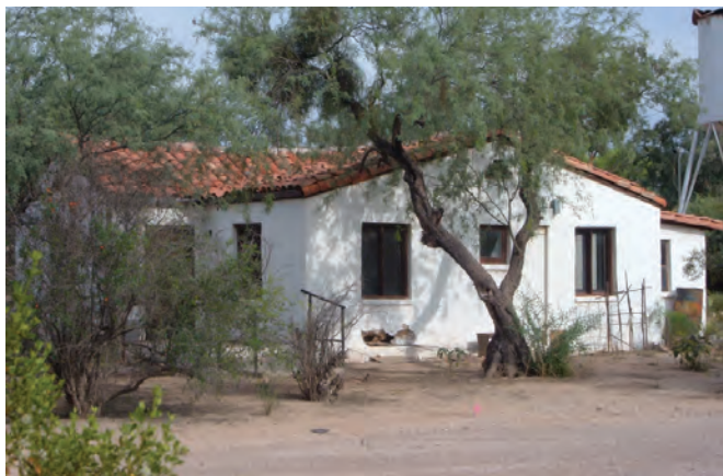
Figure 104: Adkins Residence looking southeast, August 2008.
