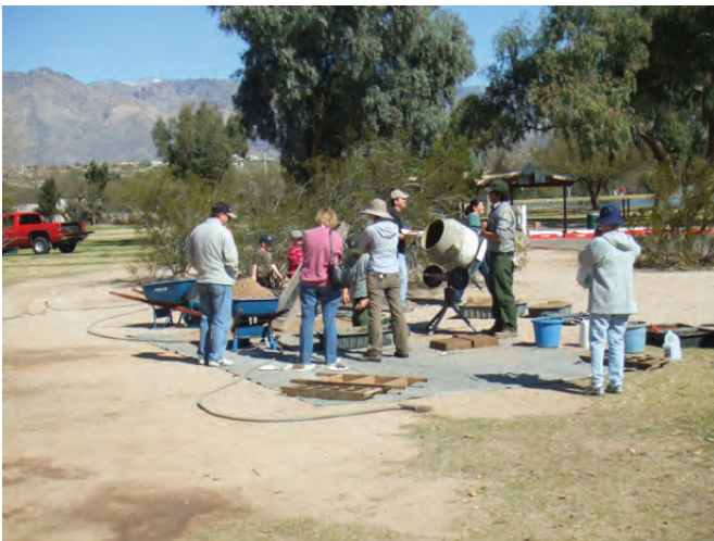
Figure 185: Making adobe during a public event near the Fort Lowell Hospital Ruins.
