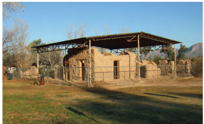
Figure 62: Existing view of Fort Lowell hospital.
