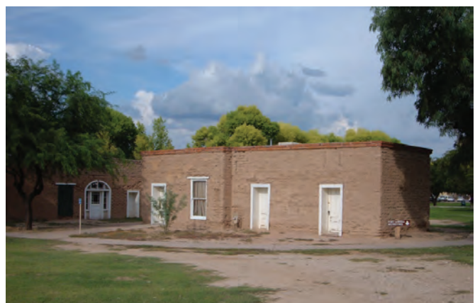
Figure 107: Fort Lowell Museum - Kitchen Reconstruction, facing northeast, 2008.
