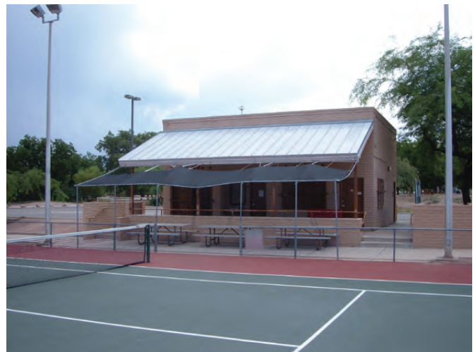
Figure 145: Fort Lowell Tennis Center.
