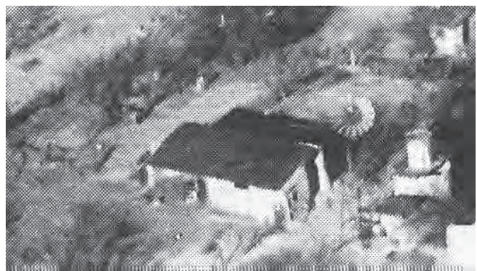
Figure 41: Officer's Quarter #1, facing southwest, 2008.
