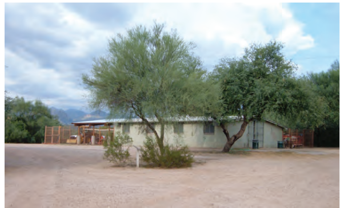
Figure 164: Existing Maintenance Building.
