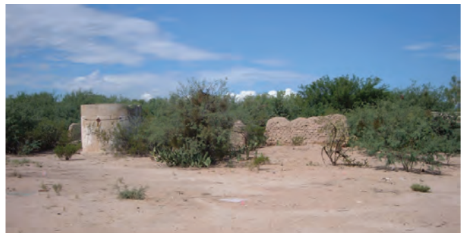
Figure 40: Officer's Quarter #1, facing southwest, 2008.
