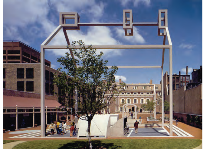
Figure 31: Franklin Court in Philadelphia serves as a useful example of the “ghosting” proposed for Officer’s Quarters #6 & 7.
