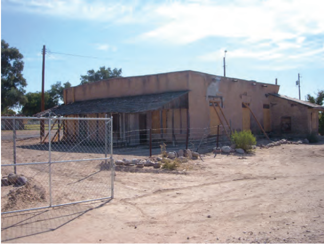
Figure 52: 2008 view of Officer's Quarters #3 from the northwest.
