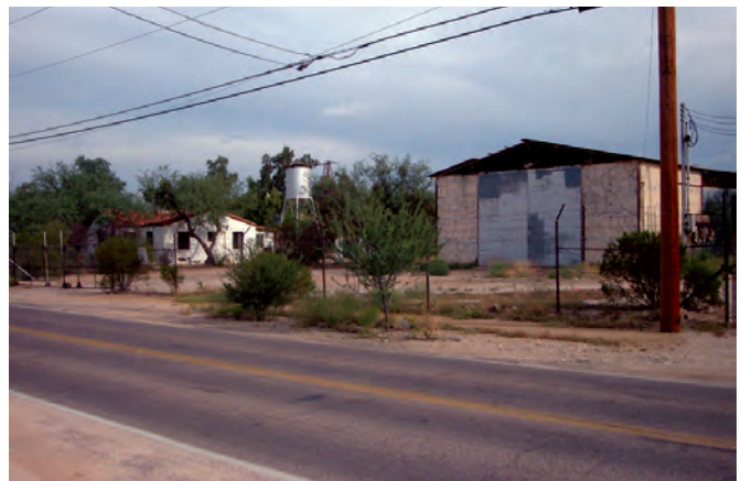
Figure 102: View from Fort Lowell Road looking southeast towards Adkins residence (left) and Adkins Steel Fabrication Shed, August 2008.
