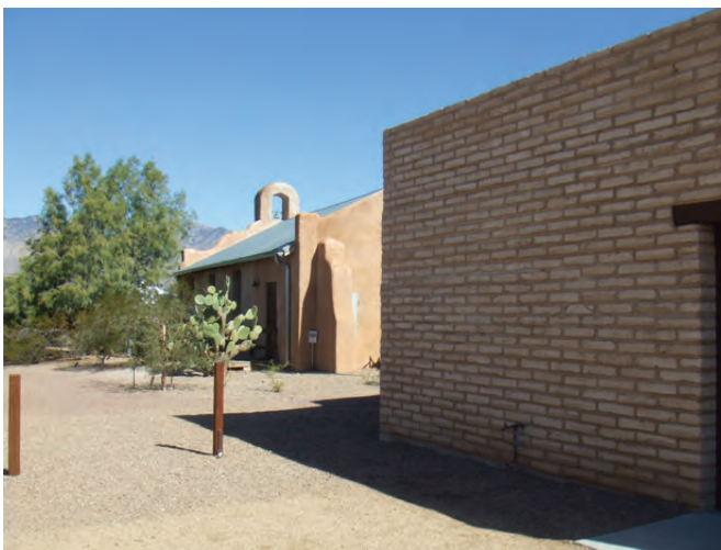
Figure 70: The new restroom building (foreground) at historic San Pedro Chapel was constructed with stabilized adobe blocks. Stabilized adobe is one material that could be used to construct contemporary buildings at Fort Lowell Park.
