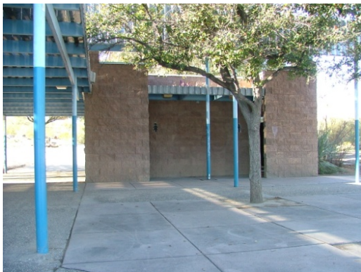
Marina Restroom Building
