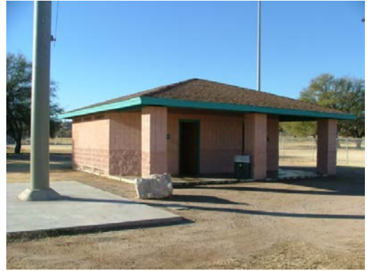
Baseball / Softball Field Restroom Building
