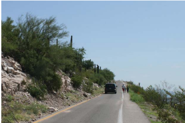
Vehicular/Pedestrian use of roadway
