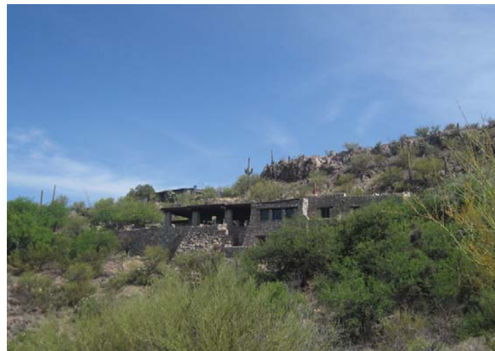
CCC era building, Colossal Cave Mountain Park Photo: WSA, 2009
