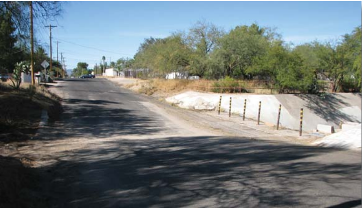
Retaining walls on the north and south sides of E. Lee Street allow that path to cross E. Lee with an at-grade street crossing with transition grades and curb ramps on the north and south sides.
