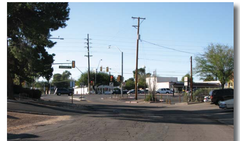
This photo of Chantilly Drive at the Pyramid Credit Union shows the topography challenge for the driveways into the credit union (left side of photo) and the room available to narrow the street paving and push the horizontal curve to the west (right side of photo) in order to transition the grade change at the credit union.
