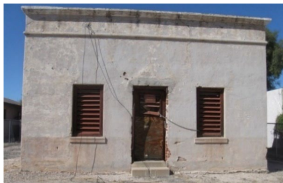
Figure 41: Old water tower at 2218 E. 1 st
