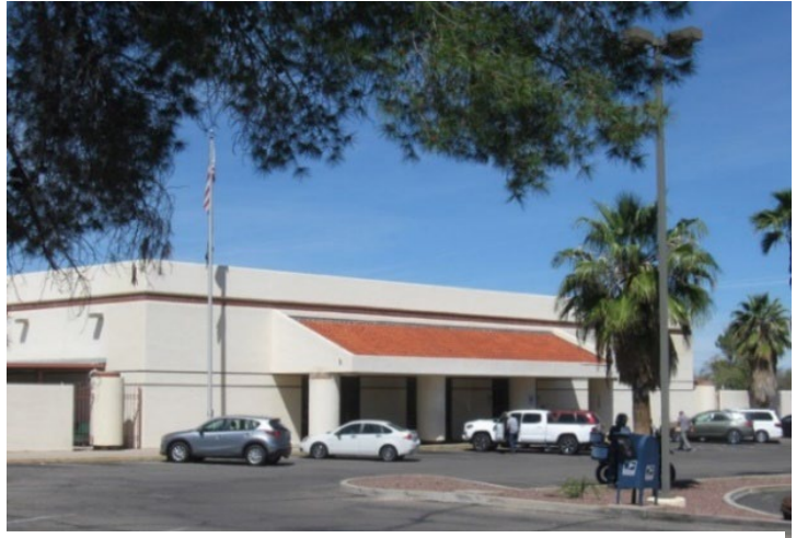
Figure 22: Sun Station Post Office.
