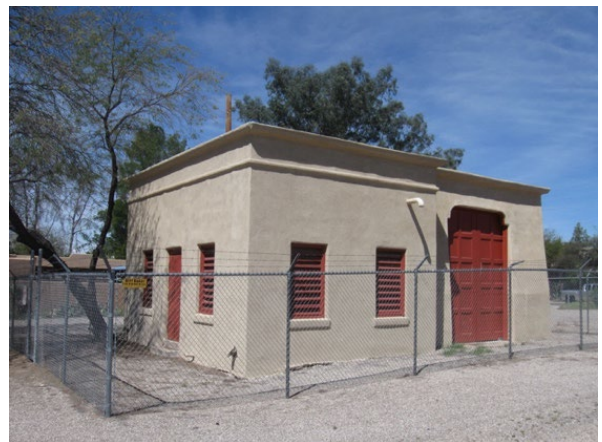
Figure 42: Renovated first floor of water tower on SW corner of 1 st Street and Tucson Boulevard.
