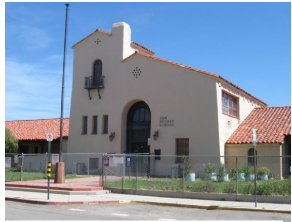
Figure 13: Sam Hughes Elementary School.
