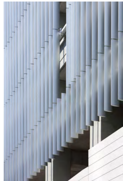
PAINTED METAL VERTICAL FIN SCREEN WALL
