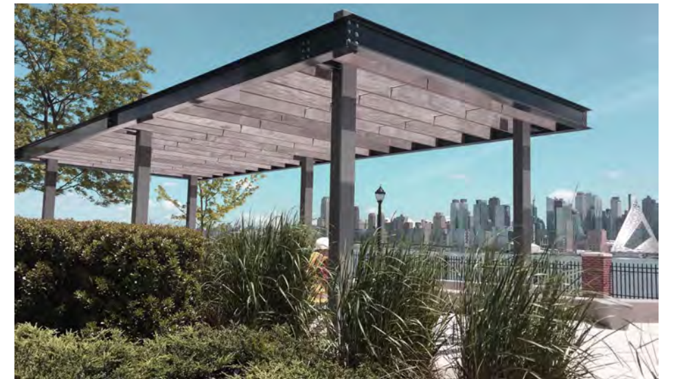
PAINTED METAL CANOPY / SHADE STRUCTURE
