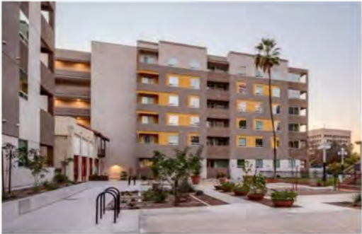
The Flin 110 S Church Avenue, Tucson, AZ 85701
