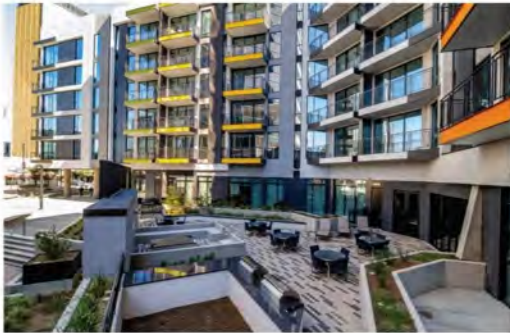
RendezVous Urban Flats 20 S Stone Avenue, Tucson, AZ 85701
