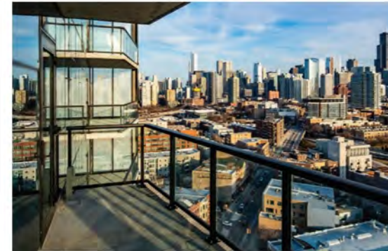
POST SUPPORTED ALUMINUM AND GLASS GAURDRAIL
