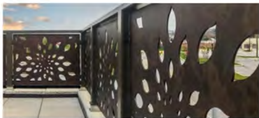
BALCONY RAILING INFILL METAL PANEL
