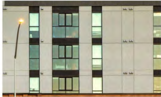
EIFS - EXTERIOR INSULATION AND FINISH SYSTEM
