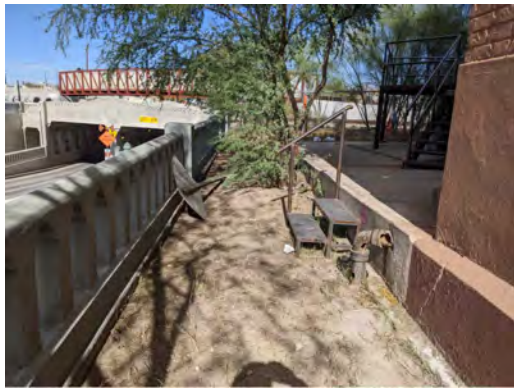
LOOKING NORTH AT EXISTING STAIRS
