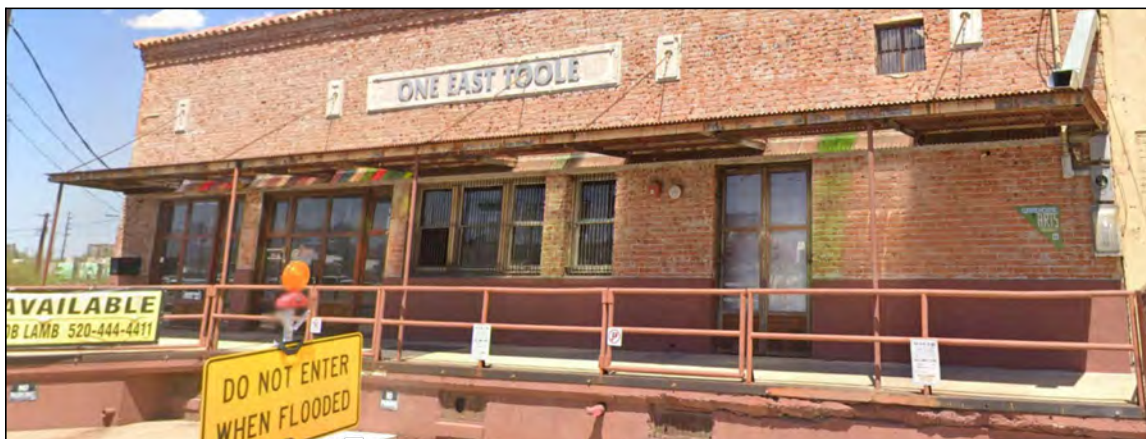
LOOKING NORTH WEST
