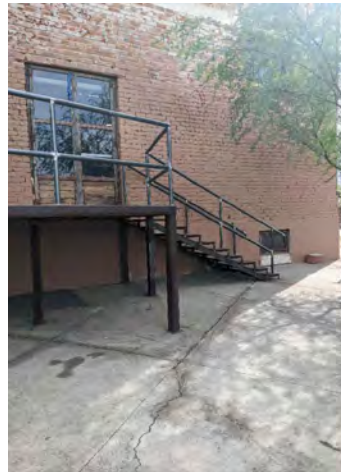
LOOKING EAST AT EXISTING STAIRS
