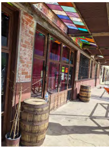
LOOKING EAST UNDER AWNING
