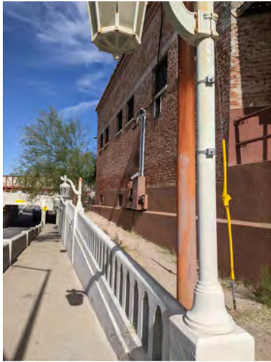
LOOKING NORTH WEST ALONG WALKWAY
