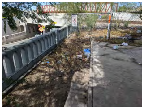
EXISTING CONCRETE LANDING
