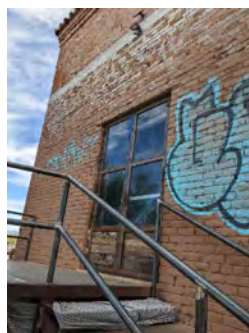
EXISTING METAL LANDING
