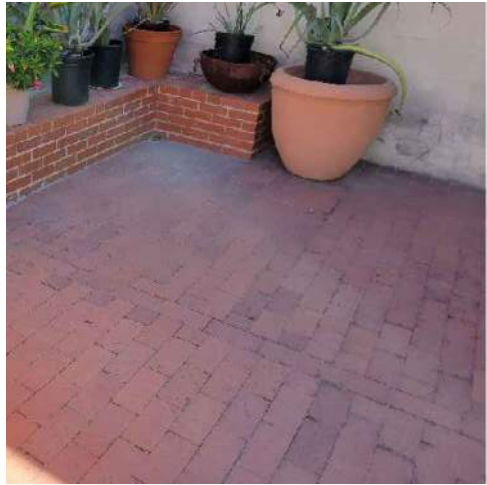
Brick pavers - reused from on-site
