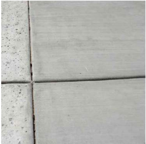
Gray concrete - header, sidewalk and seatwall cap
