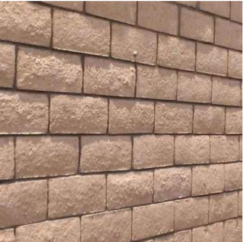
Seatwall - slump block with concrete cap
