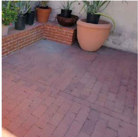
Brick pavers - reused from on-site
