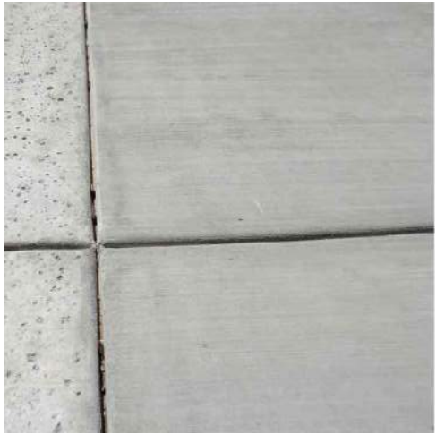
Gray concrete - header, sidewalk and seatwall cap
