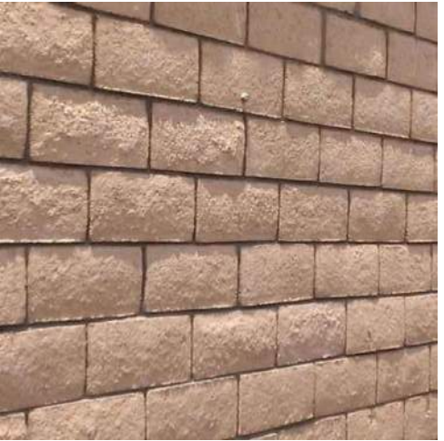
Seatwall - slump block with concrete cap
