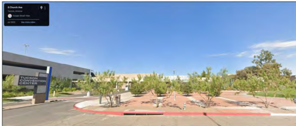
248 S Church Ave. – Convention Center Entrance. Set back from the road, but what is seen is a color palate that blends with proposed color choice for projects shade structures.
