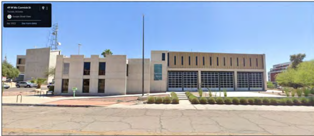
49 E Mc Cormick St - Museum of Contemporary Art. The contemporary windows mirror a similar look to solar modules. The paint color is in the same range as the projects proposed color.
