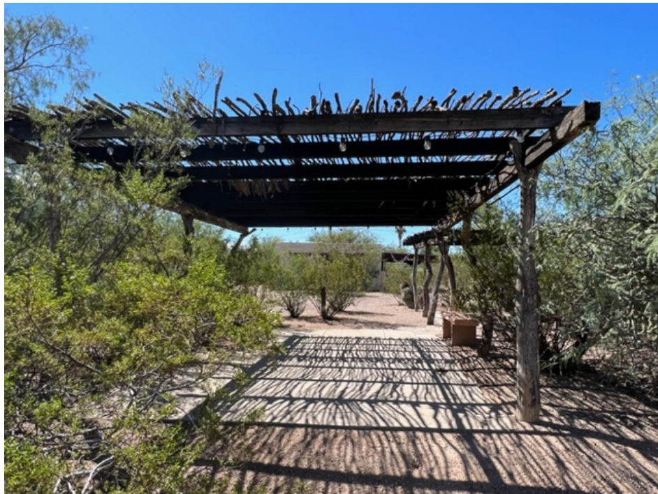
Looking North across the site, showing a detail Ramada, characterized by this vernacular architecture.
