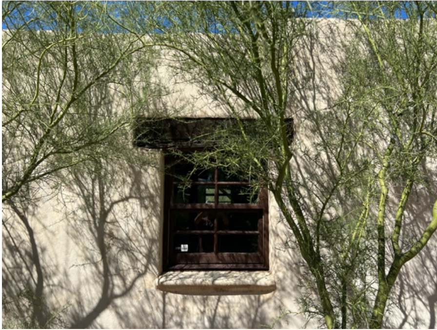
Looking South showing window style and detail , as well wall texture.
