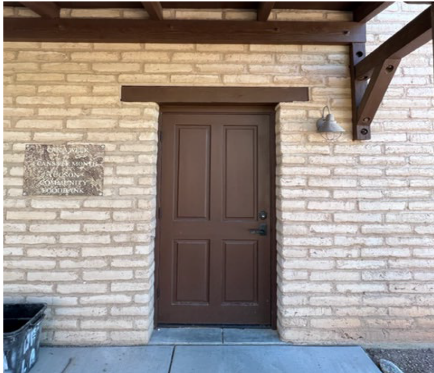
Looking North showing door style and detail , as well wall texture
