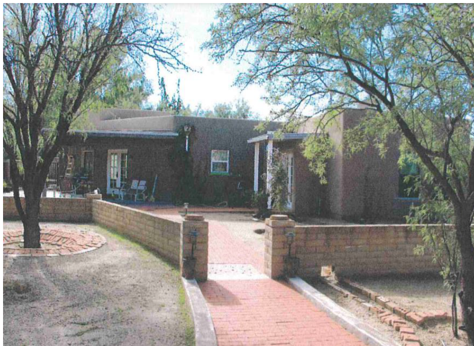
Looking at rear elevation of 5611 E Fort Lowell Rd property.
