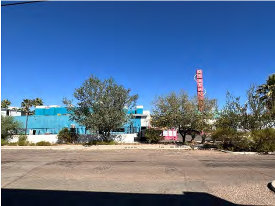
Looking north across 2 nd Street at Sahara Apartments from north side of Property.
