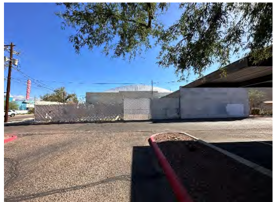
Looking east at back of building on west side of Property from parking lot west of Property.
