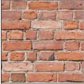
LOW BRICK WALL 03
