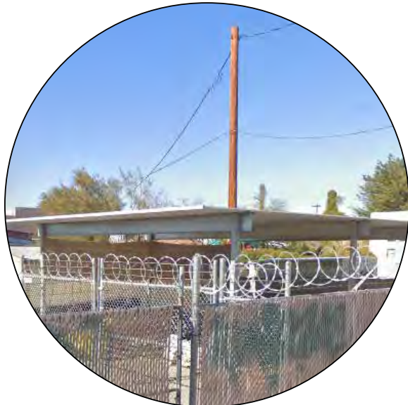
(9) STEEL SHADE STRUCTURE 733 S Arizona Ave.
