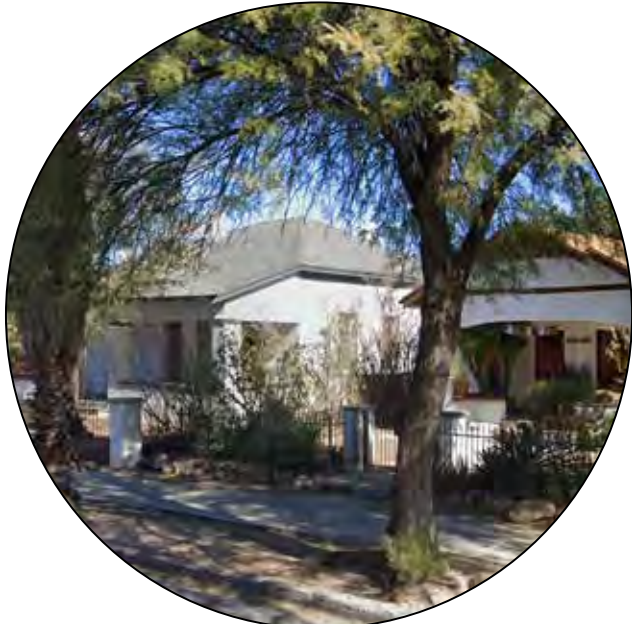
(13) LANDSCAPED SIDEWALK BUFFER 707 S 6th Ave (FRONT)
