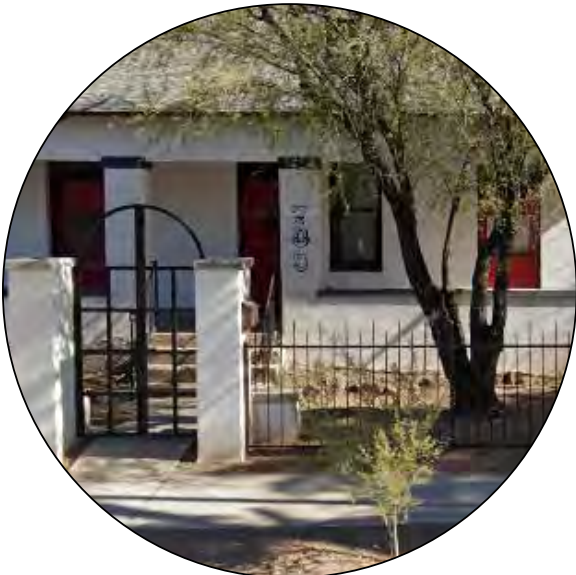
(7) METAL PICKET FENCE 705 S 6th Ave
