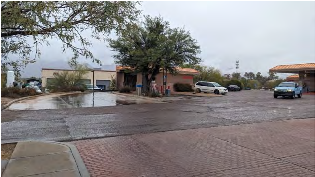
PHOTO #9: View of the adjacent gas station and accessory car wash tunnel from the southeast property corner looking northeast.
