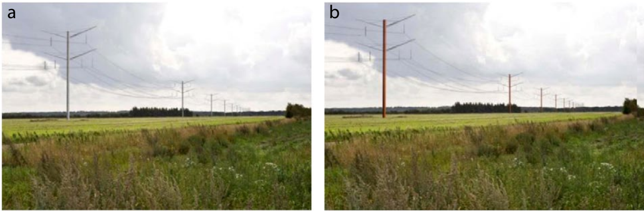
Figure 11.—When presented with two options, the public choose galvanized (a) over weathering steel (b) for the Bystrup eagle pylon. Photos by Bystrup Architects, used with permission.
