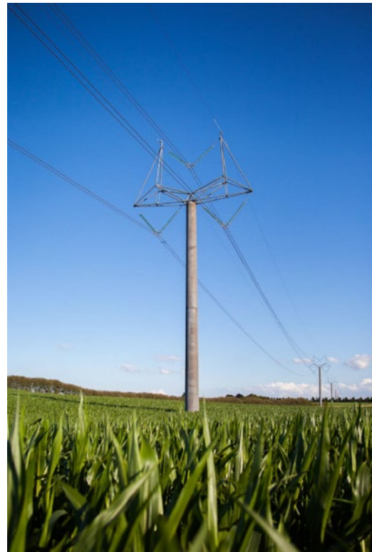
Figure 10.—The design pylon, the first pylon developed by the architectural firm Bystrup, is 60 percent the size of a traditional lattice tower. This design won a Danish government design competition in 2001. Referred to by local residents as “magic wands.” Photos by Bystrup Architects, used with permission.
