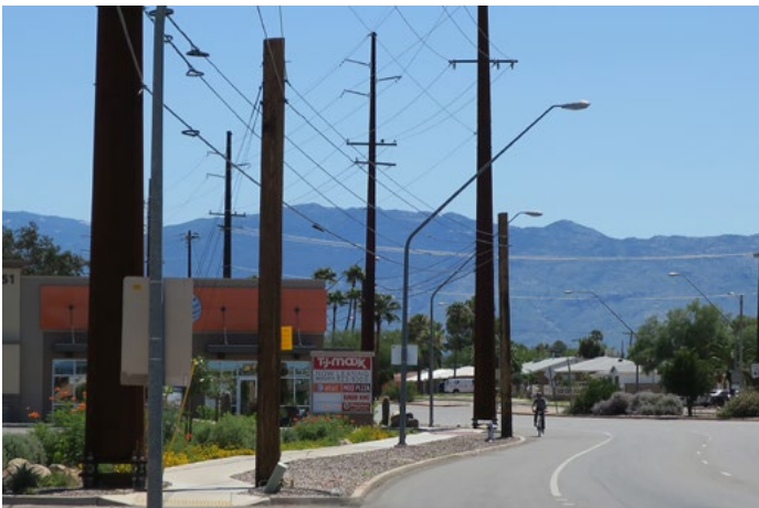
Figure 4.—Poles that remain after the pole owner has relocated to a new pole are known as redundant poles. Photos by Ellen Barth Alster, used with permission.
