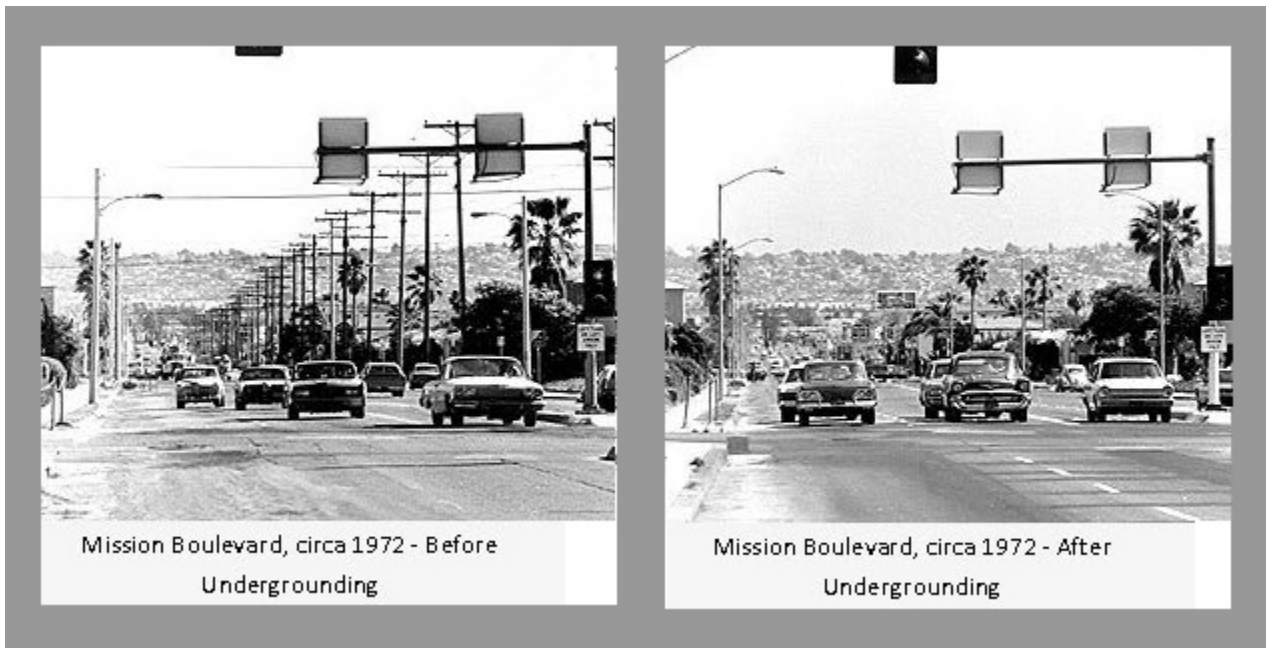
Figure 8.—Before and after illustration of Mission Boulevard in San Diego from the Master Plan, Utilities Undergrounding Program. Photos from City of San Diego 2017.
