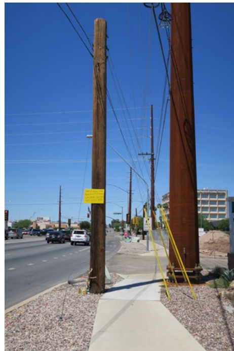
Figure 4.—Poles that remain after the pole owner has relocated to a new pole are known as redundant poles. Photos by Ellen Barth Alster, used with permission.
