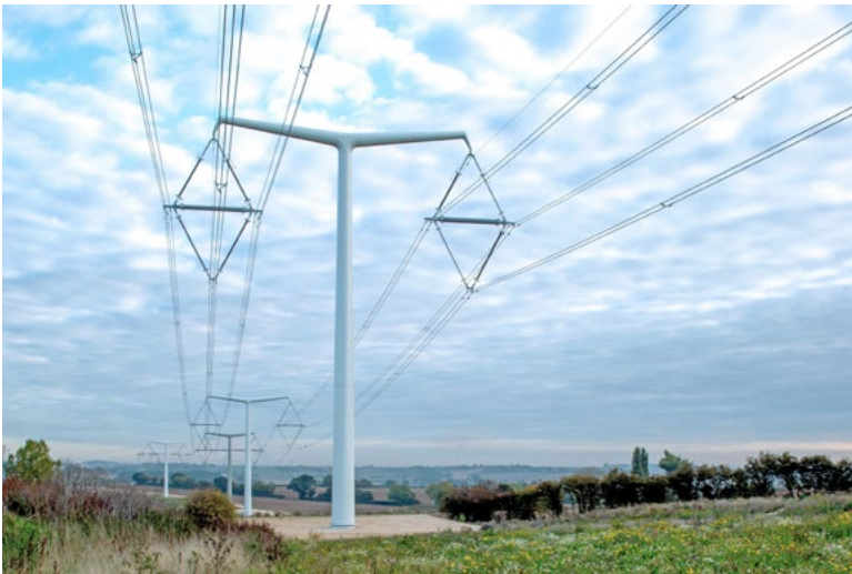
Figure 12.—A test line using the T-pylon, by the architectural firm Bystrup, won a design competition in the United Kingdom in 2011 as its national grid expands, moving away from coal, oil, and gas, toward newer sustainable energy sources. A test line is shown here. Photo by Bystrup Architects, used with permission.
