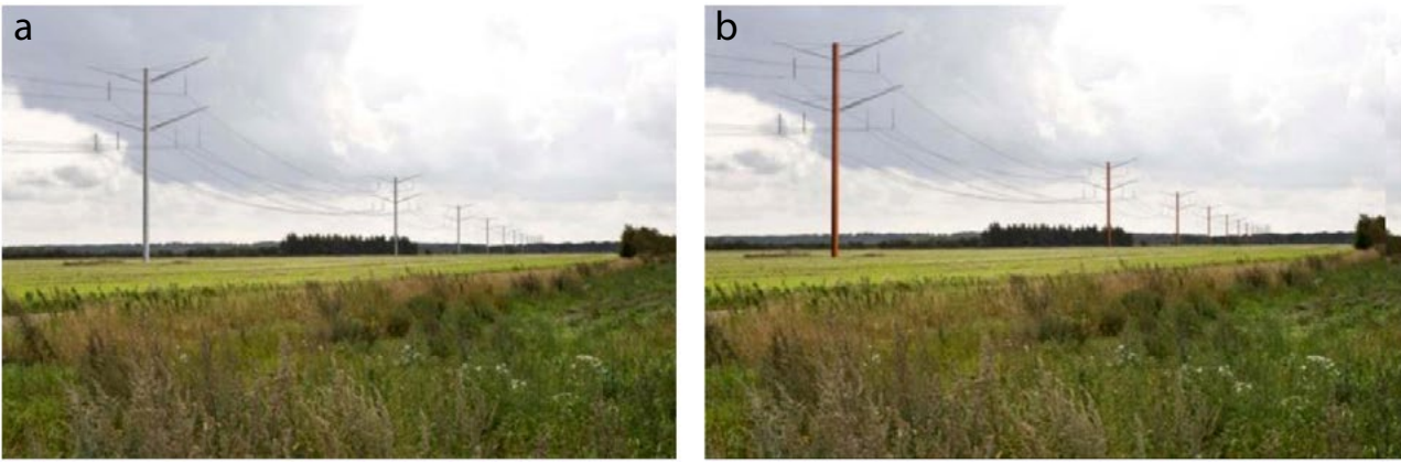
Figure 11.—When presented with two options, the public choose galvanized (a) over weathering steel (b) for the Bystrup eagle pylon. Photos by Bystrup Architects, used with permission.
