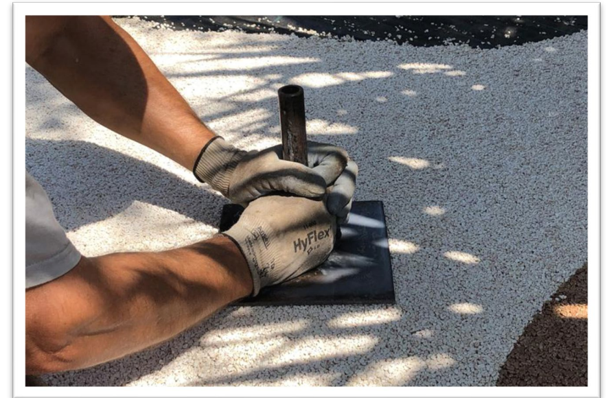
Dust Proof Paving Example
