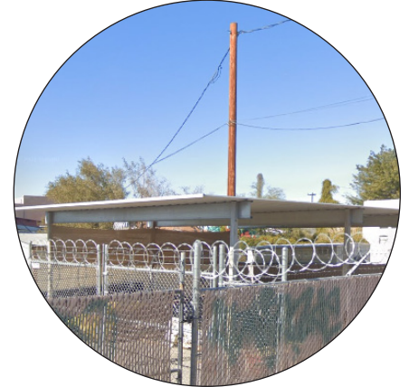
(9) STEEL SHADE STRUCTURE 733 S Arizona Ave.
