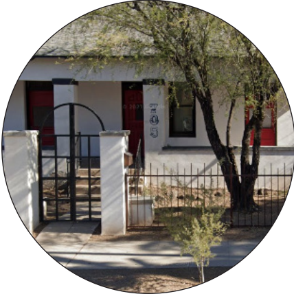
(7) METAL PICKET FENCE 705 S 6th Ave
