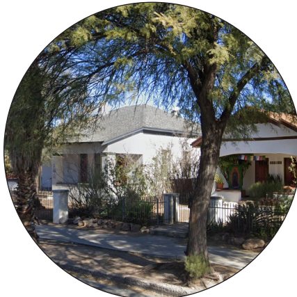
(13) LANDSCAPED SIDEWALK BUFFER 707 S 6th Ave (FRONT)
