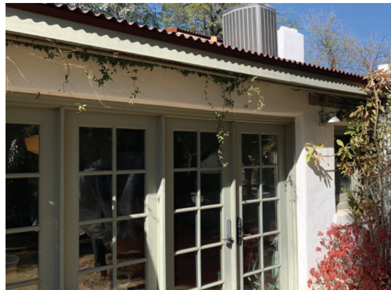
View of east facade windows and french door
