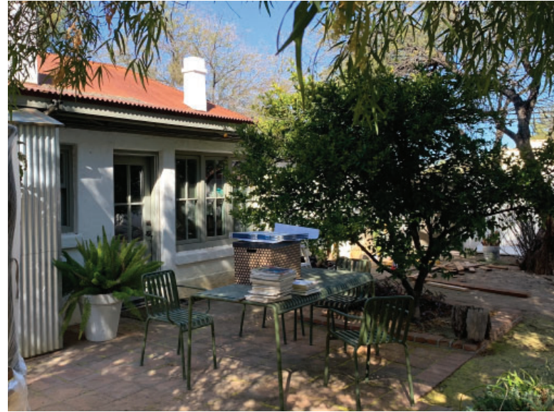
View of east facade windows and door
