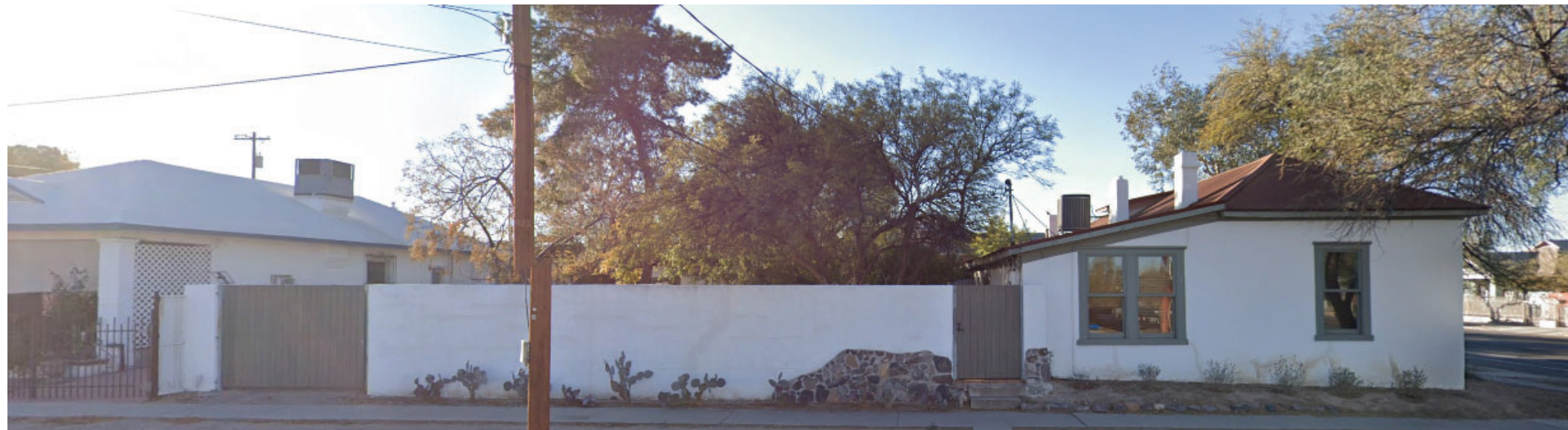
View of north facade (E 18th st)
