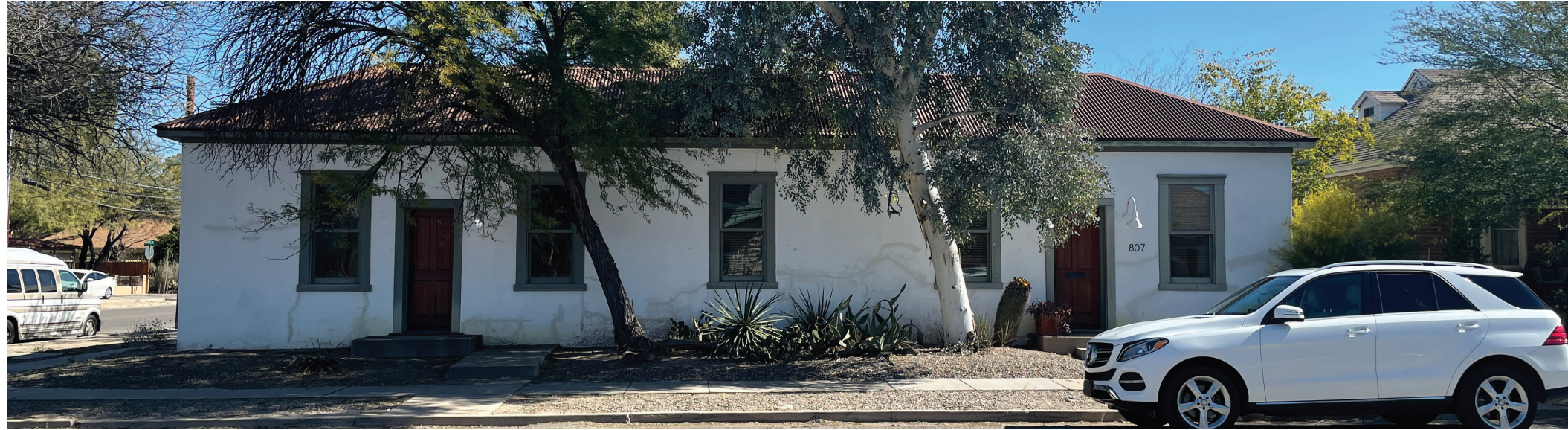
View of west facade (S 4th ave)
