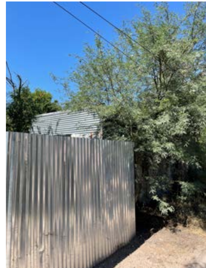
408 W Simpson, Side yard Alley. Accessory Structure, shed, 9 to 11' tall near lot line.
