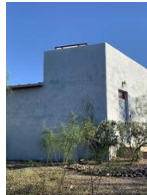
701 S. Osborne Steel Column and Shade Cloth
