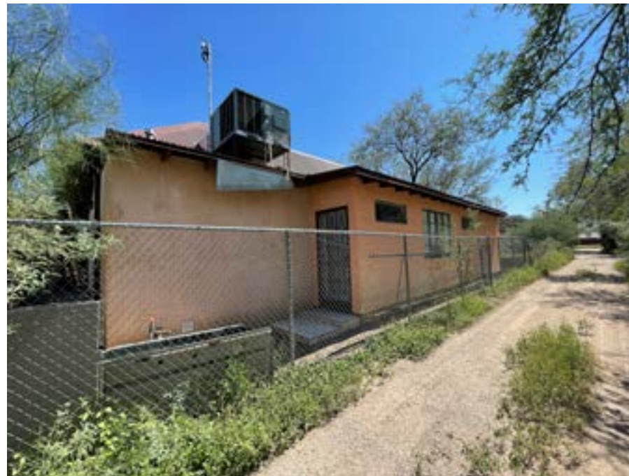
552 Samaniego Ave, Alley. Accessory Structure, converted porch, 10' tall near lot line.
