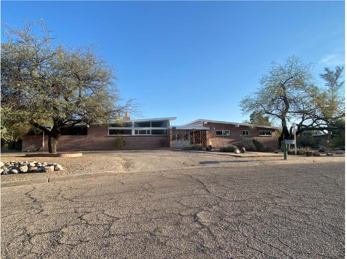
Photo 7, WH 079, Bernard Friedman House II, 5602 E North Wilshire Drive, 1956, looking south.
