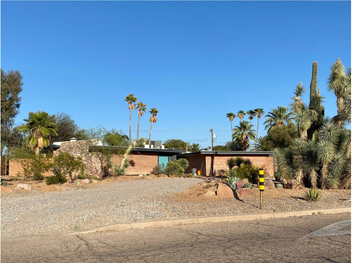
Photo 4, WH 032, Harry and Darlyne Walker House, 5823 East North Wilshire Drive, 1958, looking southeast.
