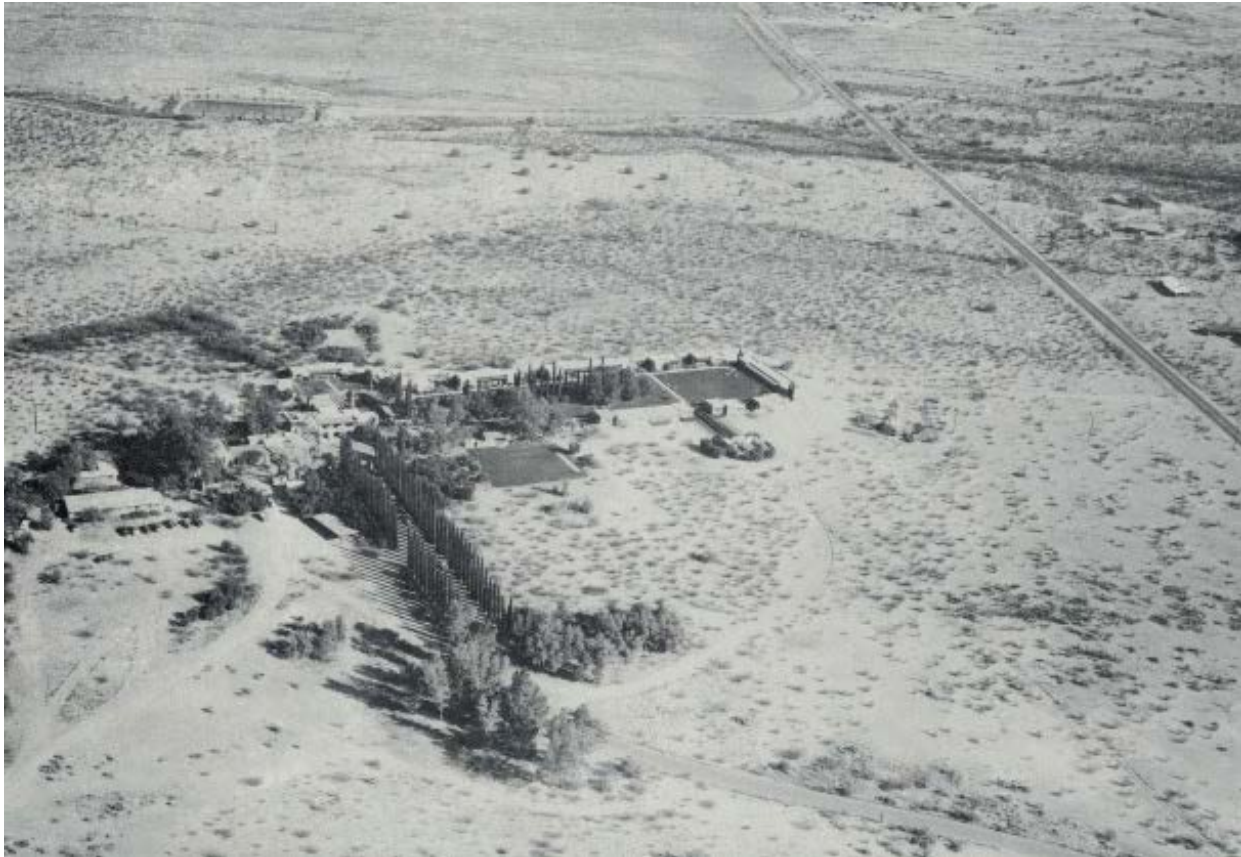
Figure 20. El Dorado Lodge Aerial View, 1950.
