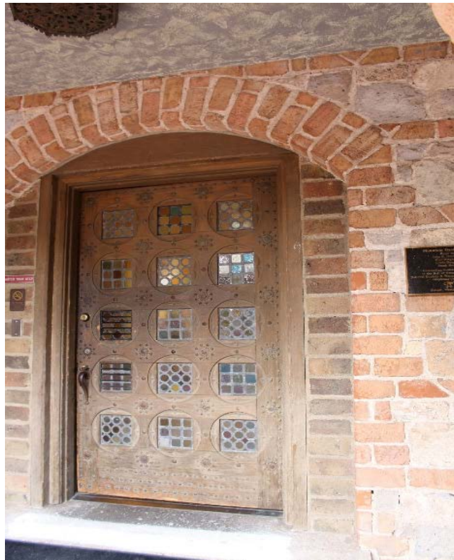
Figure 4. Hand-hewn Main Entry door of wood, iron and colored glass.
