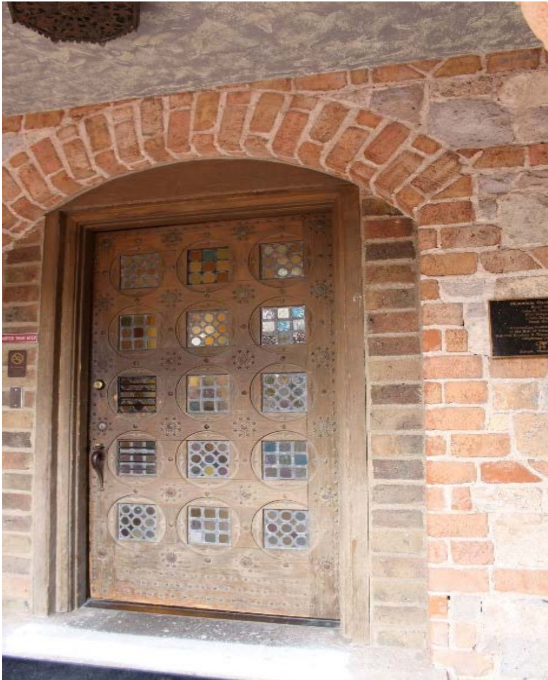
5 of 16. AZ_PimaCounty_ElDoradoLodge_0005 Hand-hewn Main Entry door of wood, iron and colored glass, Mountain Oyster Club. Facing East
