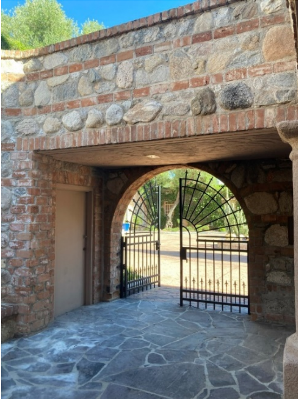
9 of 16 . AZ_PimaCounty_ElDoradoLodge_0009 B Building. Arched wrought iron entrance to Inner Courtyard at Mountain Oyster Club. Facing Northwest
