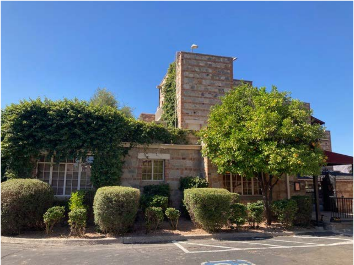
7 of 16 . AZ_PimaCounty_ElDoradoLodge_0007 South façade of the Mountain Oyster Club from parking lot. Facing North
