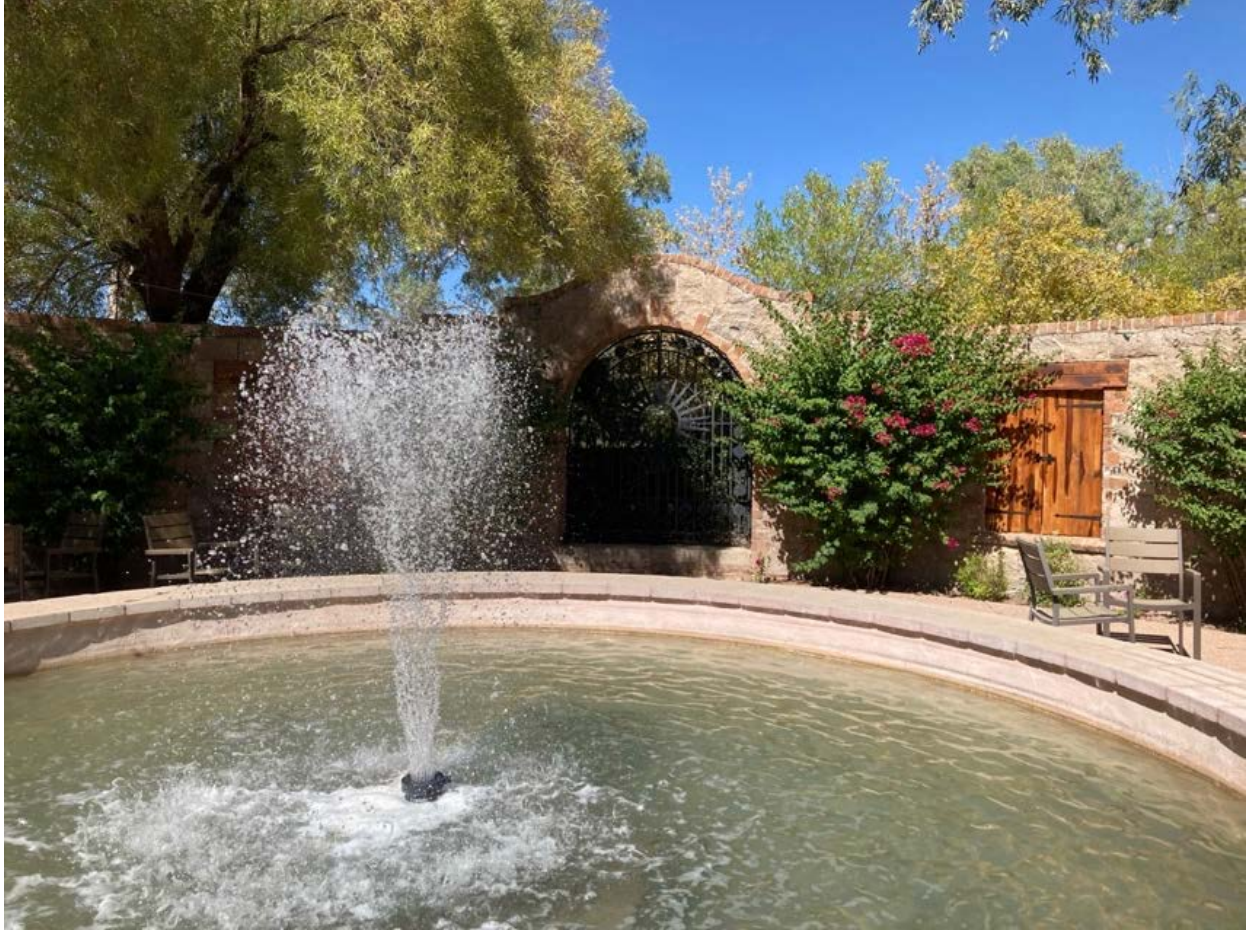
16 of 16 . AZ_PimaCounty_ElDoradoLodge_0016 Existing site of Water-Cooling Tower on the Lower Back Patio of Mountain Oyster Club. Facing West
