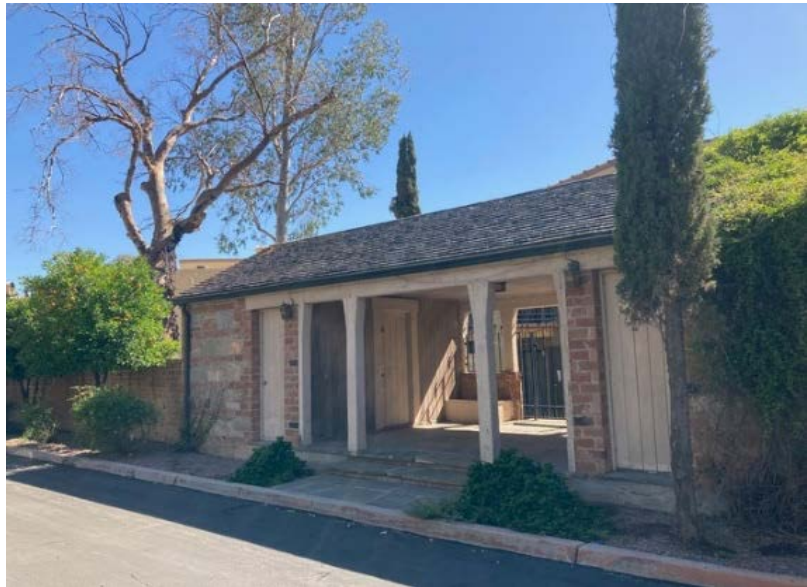
Figure 5. The Bathhouse, Eastern Perimeter of South Parking Lot. AZ_PimaCounty_ElDoradoLodge_0006
