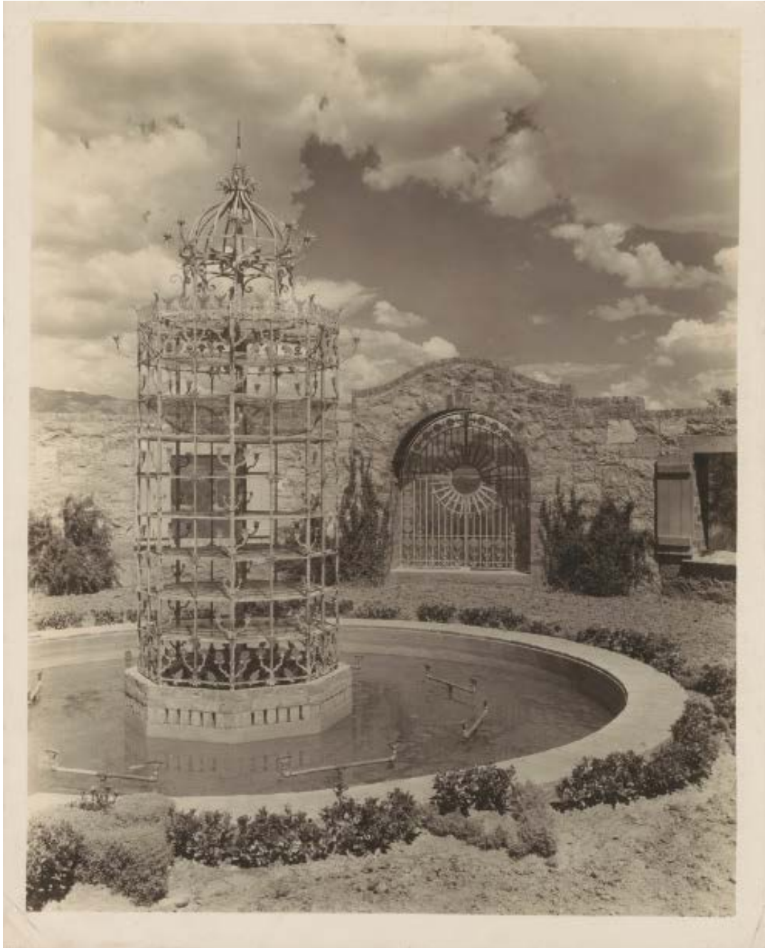
Figure 22. Original Wrought Iron Water-Cooling Tower, Circa 1946.
