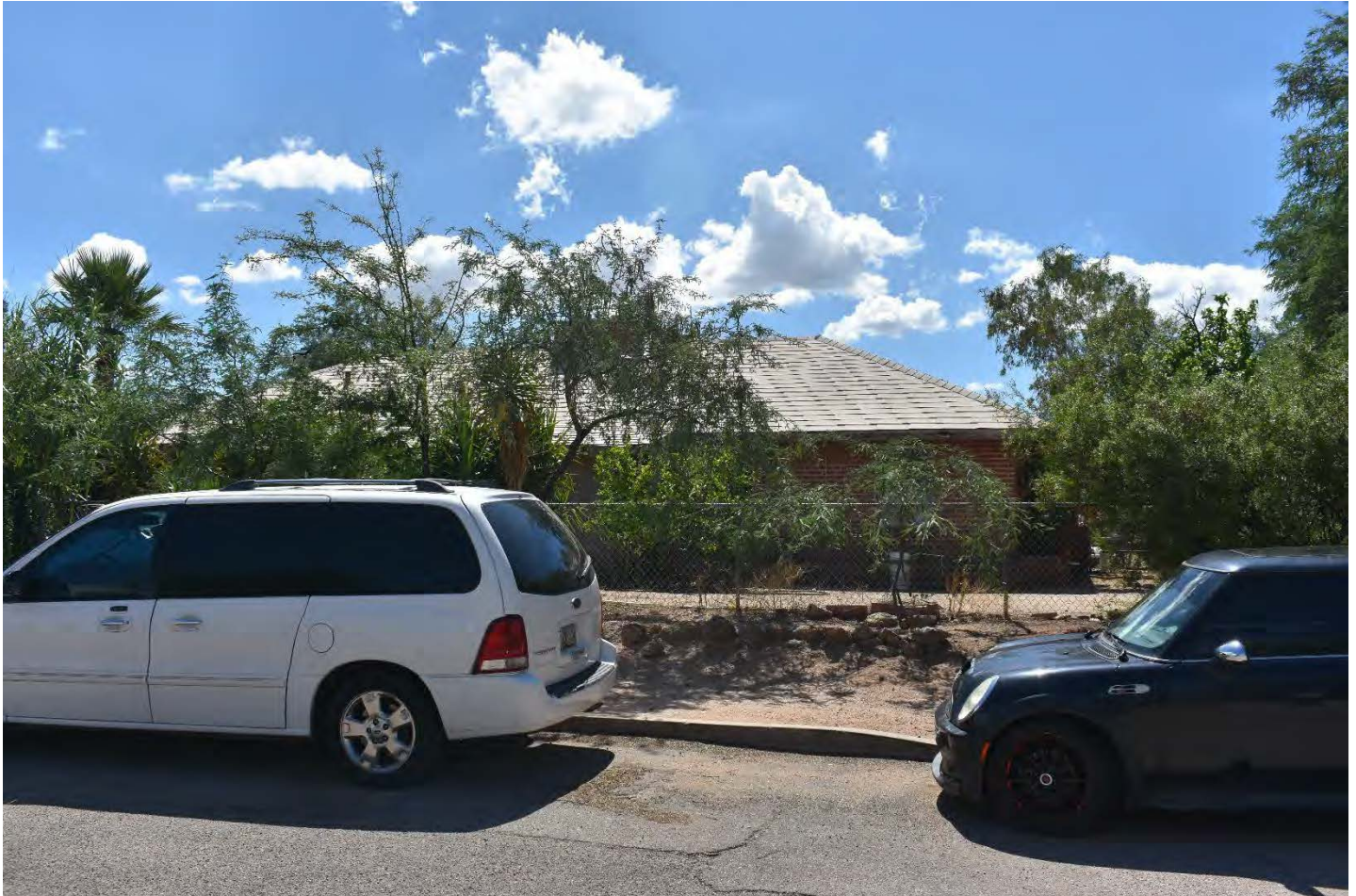
634 South Santa Rita Avenue, east elevation, view looking west, Logan Simpson, 2021.
