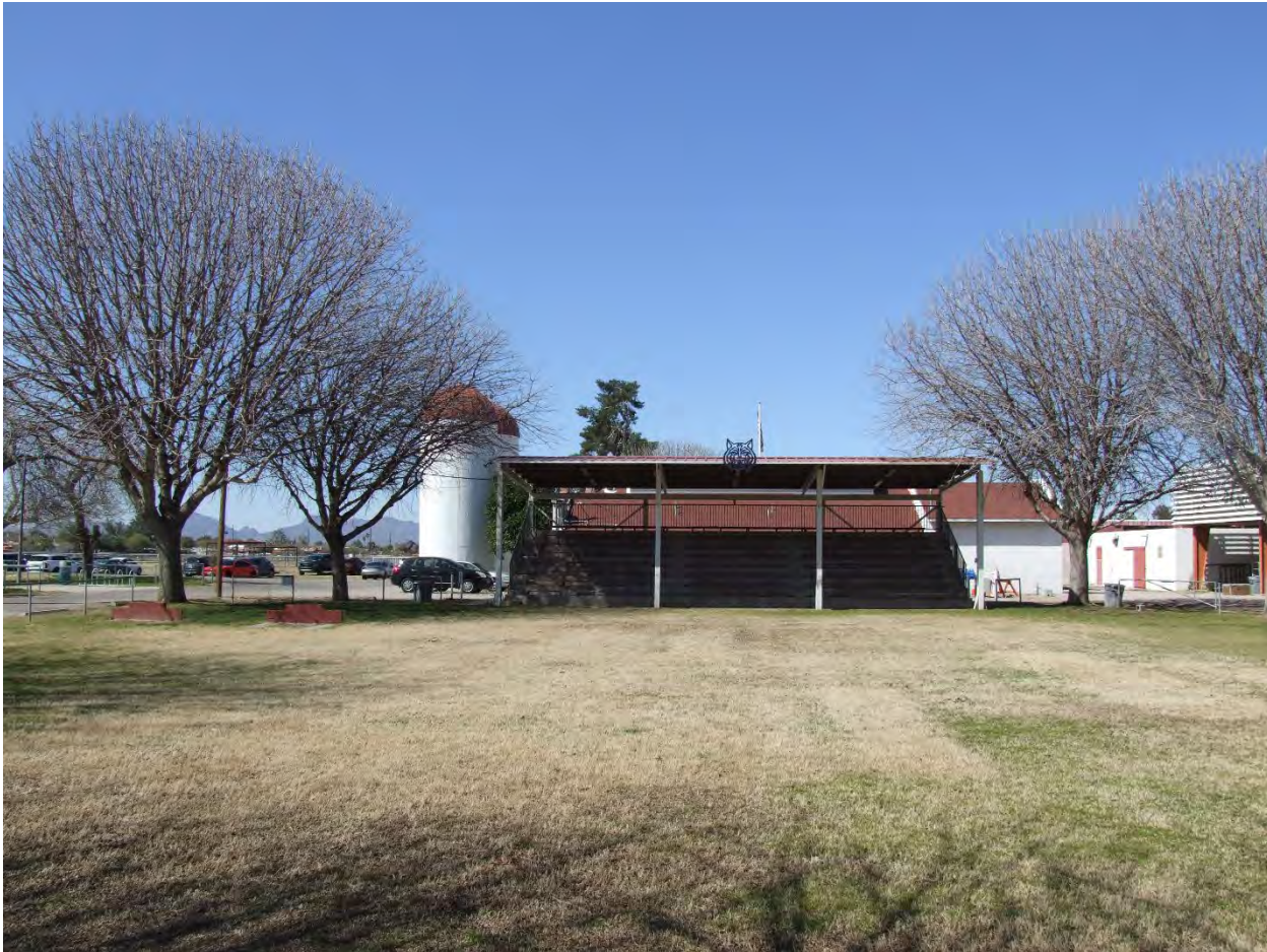
The University of Arizona Campus Agricultural Center, Grandstand and Field, view facing west. WestLand Resources, Inc., March 8, 2023.
