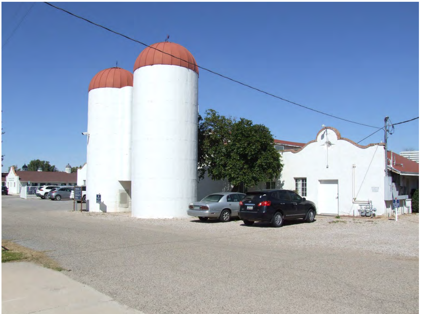
The University of Arizona Campus Agricultural Center, Office Building, view facing northwest, WestLand Resources, Inc., March 8, 2023.
