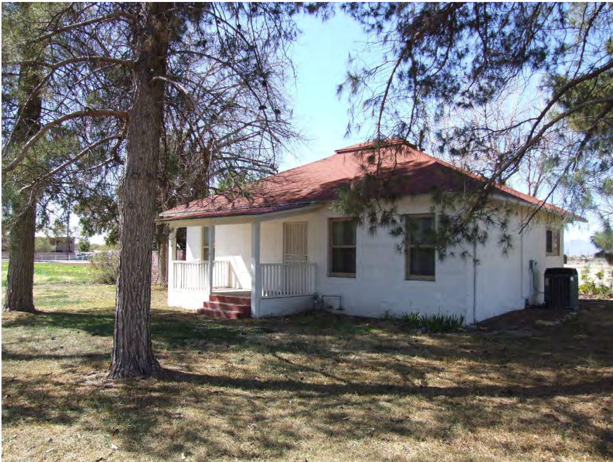
The University of Arizona Campus Agricultural Center, Main Residence, east and north elevations, view facing southwest. WestLand Resources, Inc., March 8, 2023.
