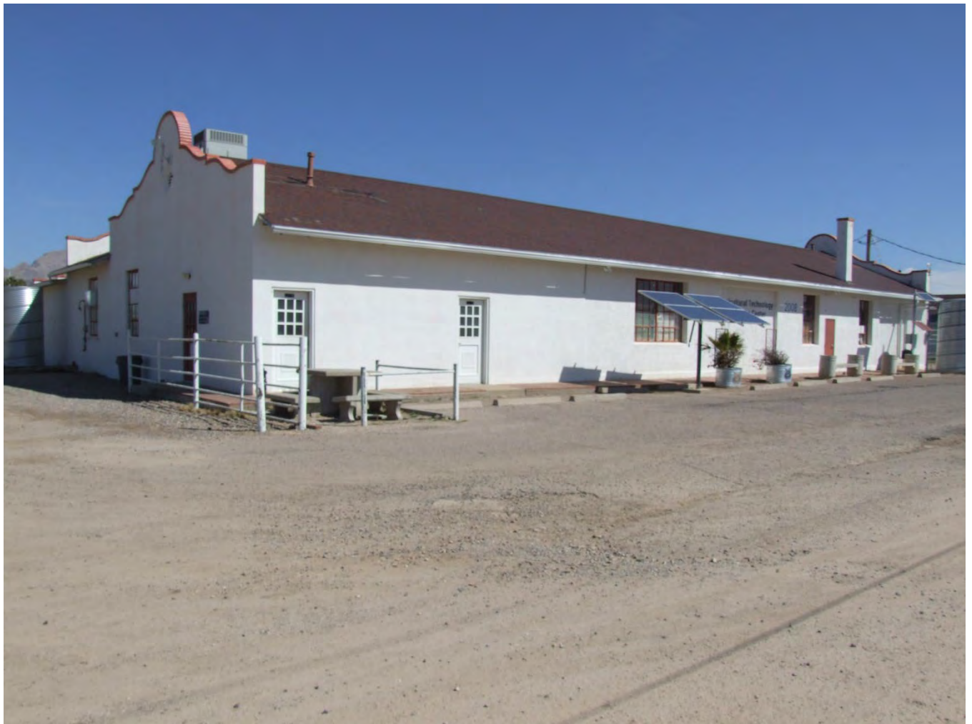
The University of Arizona Campus Agricultural Center, Agricultural Education Facility Building, view facing northeast. WestLand Resources, Inc. March 8, 2023.
