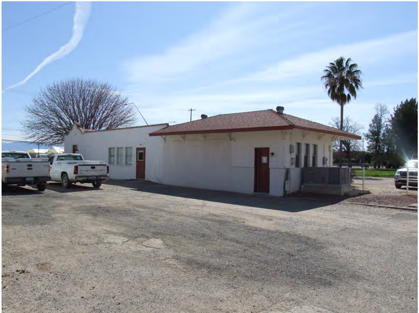
Photograph 24. West and north elevations of the Farm Office; view facing southwest (AZ_Pima County_UA Campus Agricultural Center Historic District_0024).
