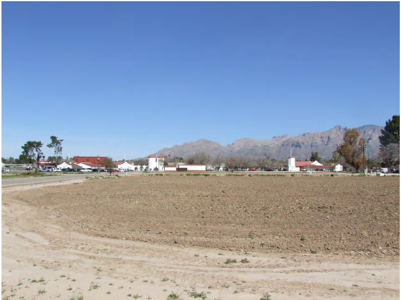
Photograph 7. Overview of agricultural fields and pastures; view facing north (AZ_Pima County_UA Campus Agricultural Center Historic District_0007).
