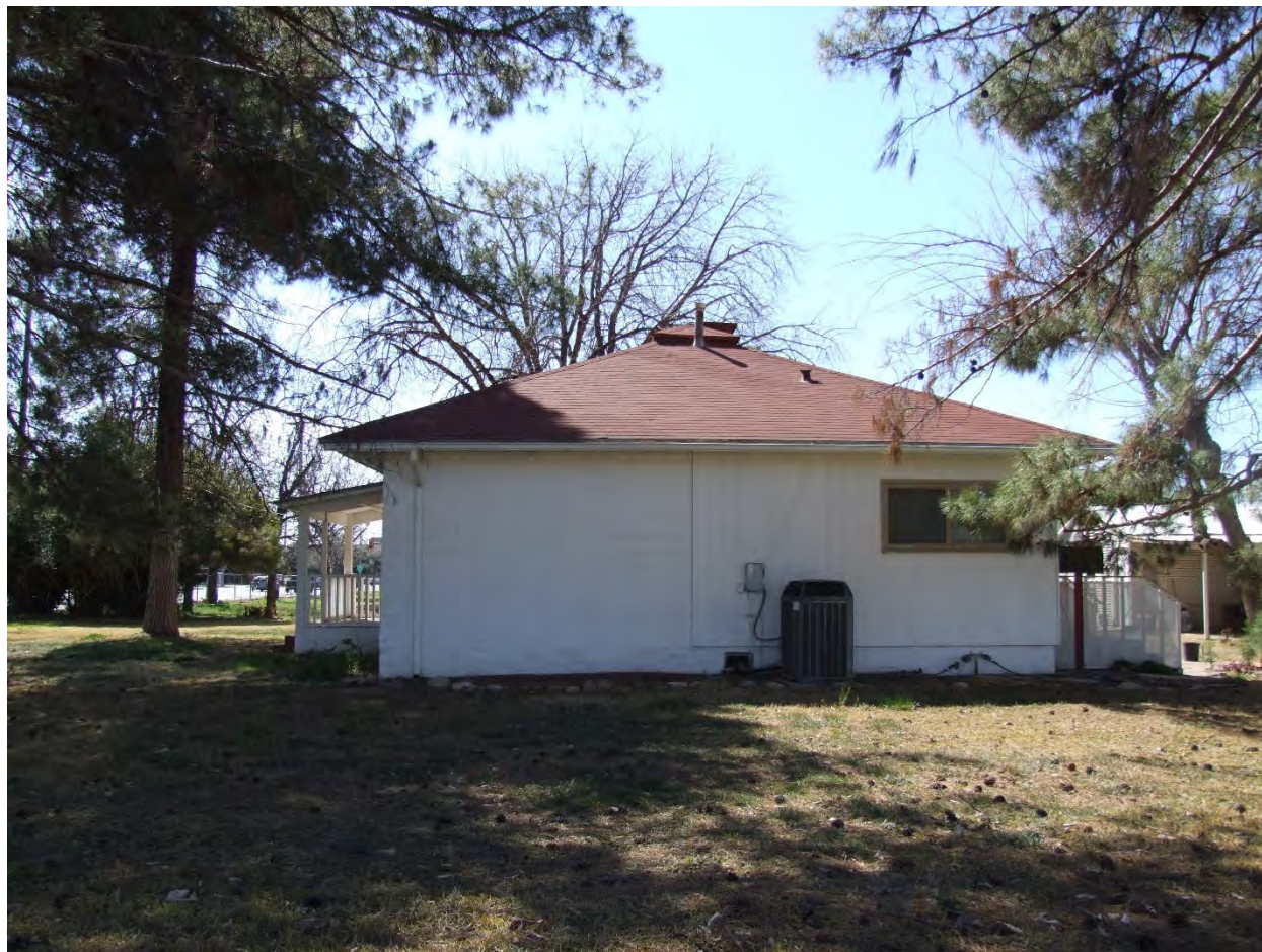
Photograph 4. Overview of north elevation of the Residence; view facing south (UA_Pima County_UA Campus Agricultural Center Historic District_0004)
