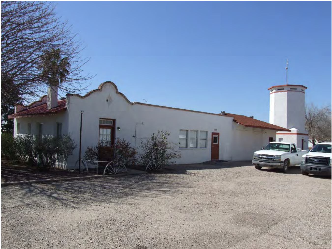
Photograph 23. East and north elevations of the Farm Office; view facing southwest (AZ_Pima County_UA Campus Agricultural Center Historic District_0023).
