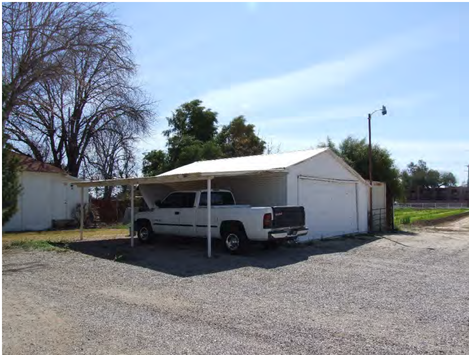
Photograph 3. Overview of the carport at the Residence; view facing southeast (UA_Pima County_UA Campus Agricultural Center Historic District_0003)
