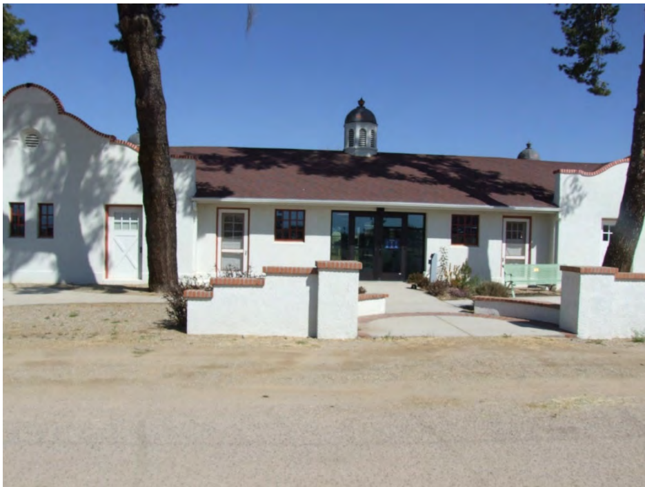
Photograph 20. South elevation overview of the Equine Education Building; view facing north (AZ_Pima County_UA Campus Agricultural Center Historic District_0020)
