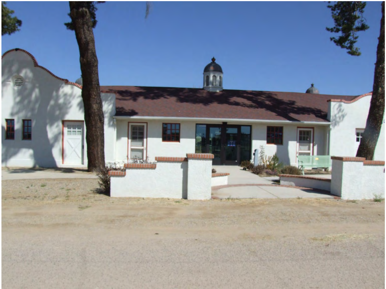
Photograph 20. South elevation overview of the Equine Education Building; view facing north (AZ_Pima County_UA Campus Agricultural Center Historic District_0020).
