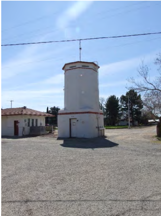
Photograph 11. East and north elevations of the Network Storage Building and Water Tower; view facing southeast (AZ_Pima County_UA Campus Agricultural Center Historic District_0011)
