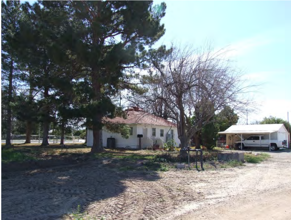
Photograph 2. North and west elevations of the Residence with carport; view facing southeast (UA_Pima County_UA Campus Agricultural Center Historic District_0002)
