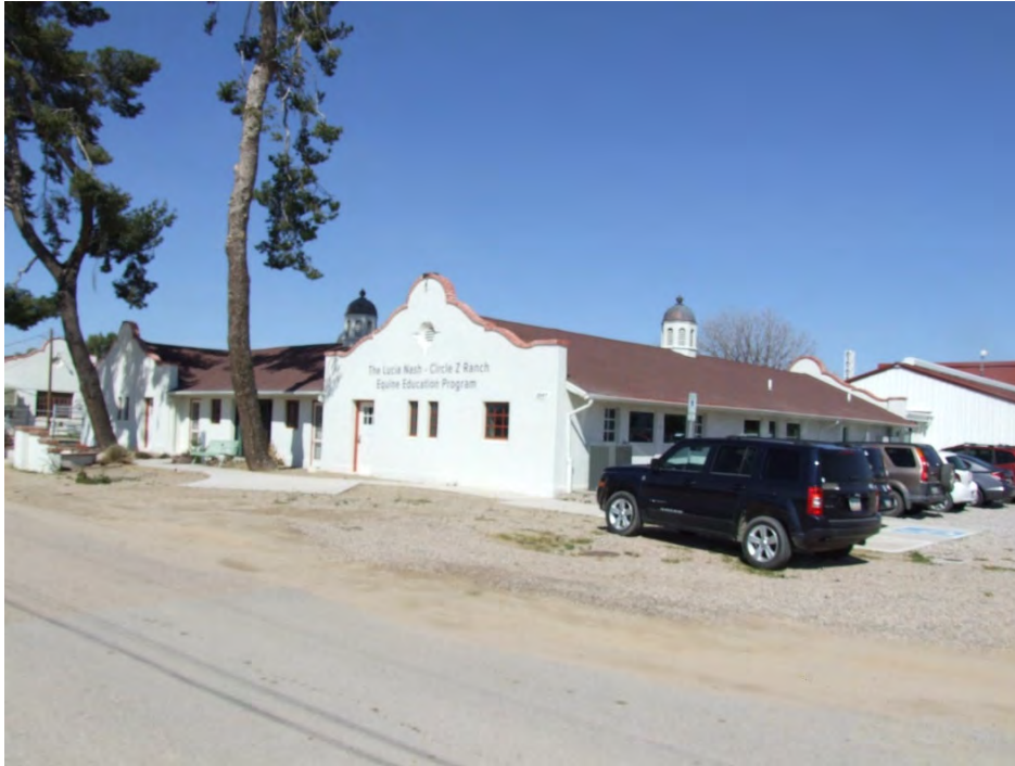
Photograph 19. East and south elevations of the Equine Education Building; view facing northwest (AZ_Pima County_UA Campus Agricultural Center Historic District_0019)
