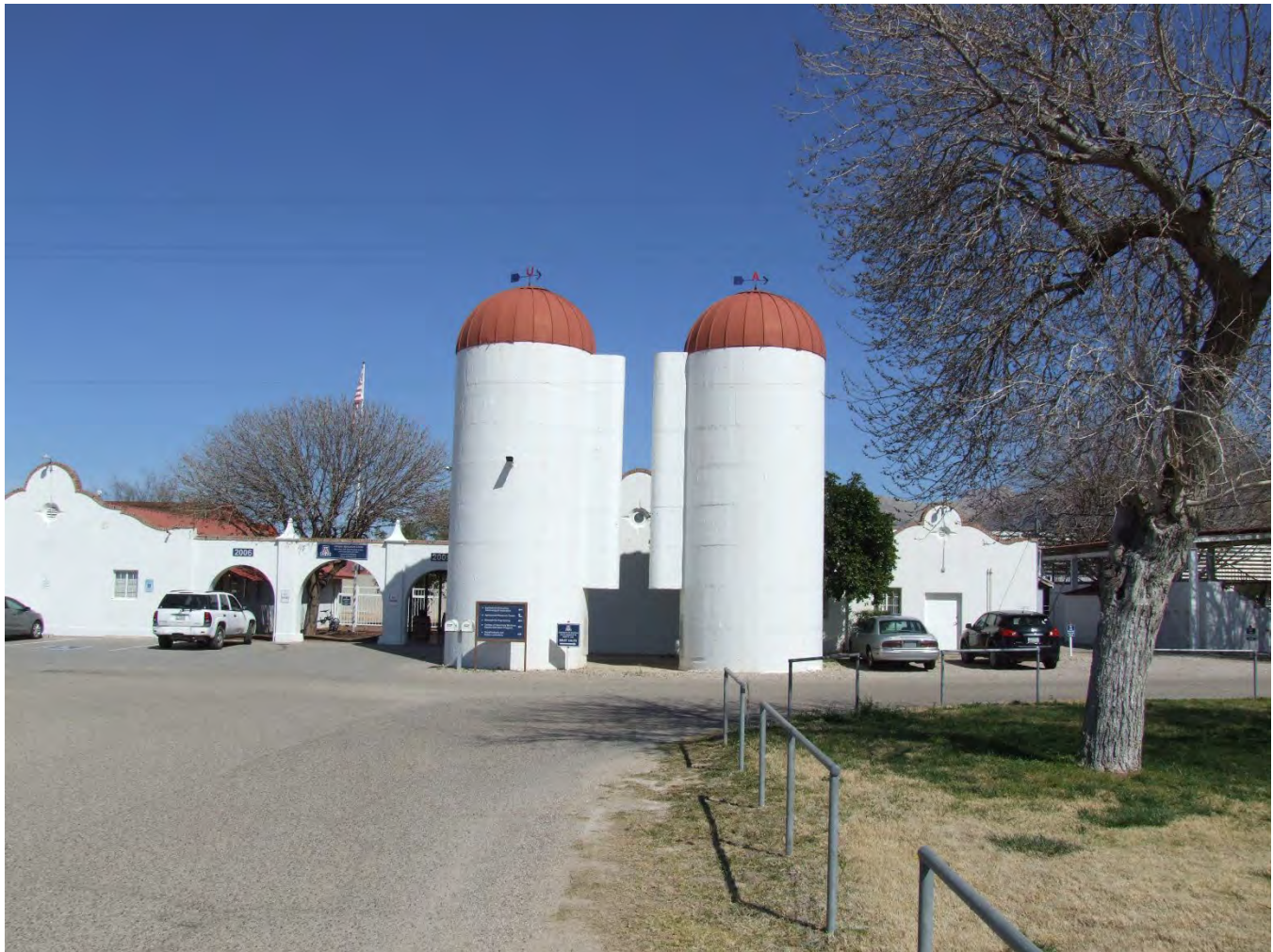
Photograph 15. Overview of south elevations of the two paired silos; view facing north (UA_Pima County_UA Campus Agricultural Center Historic District_0015).
