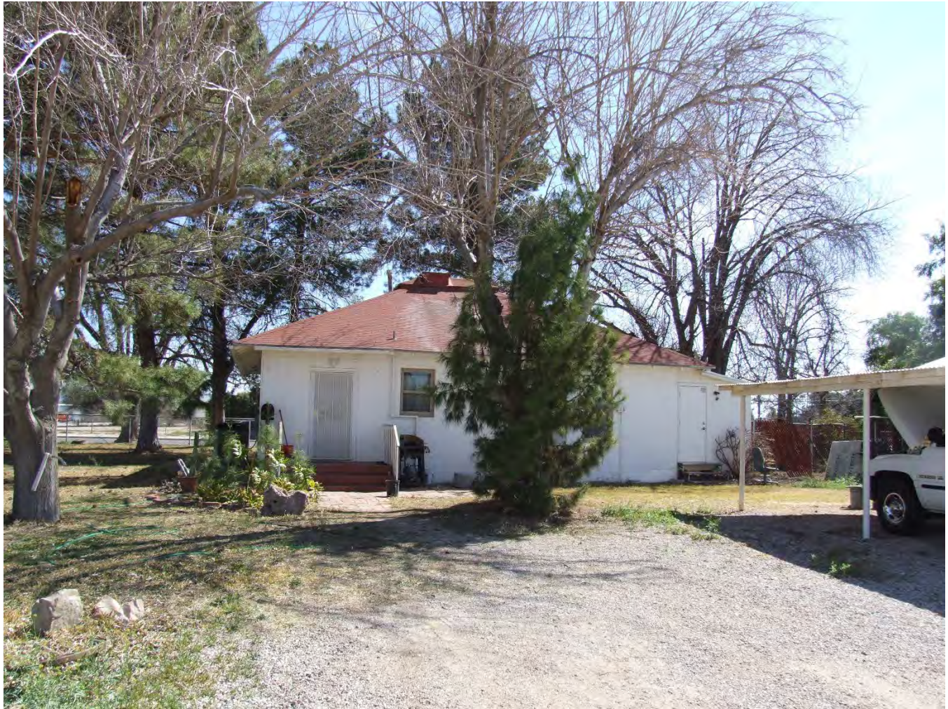
Photograph 5. West elevation of the Residence and back entryway; view facing east (UA_Pima County_UA Campus Agricultural Center Historic District_0005).
