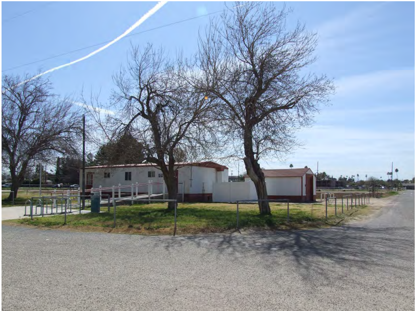
Photograph 28. West and north elevations of the modular Storage building and storage shed; view facing southeast (UA_Pima County_UA Campus Agricultural Center Historic District_028).
