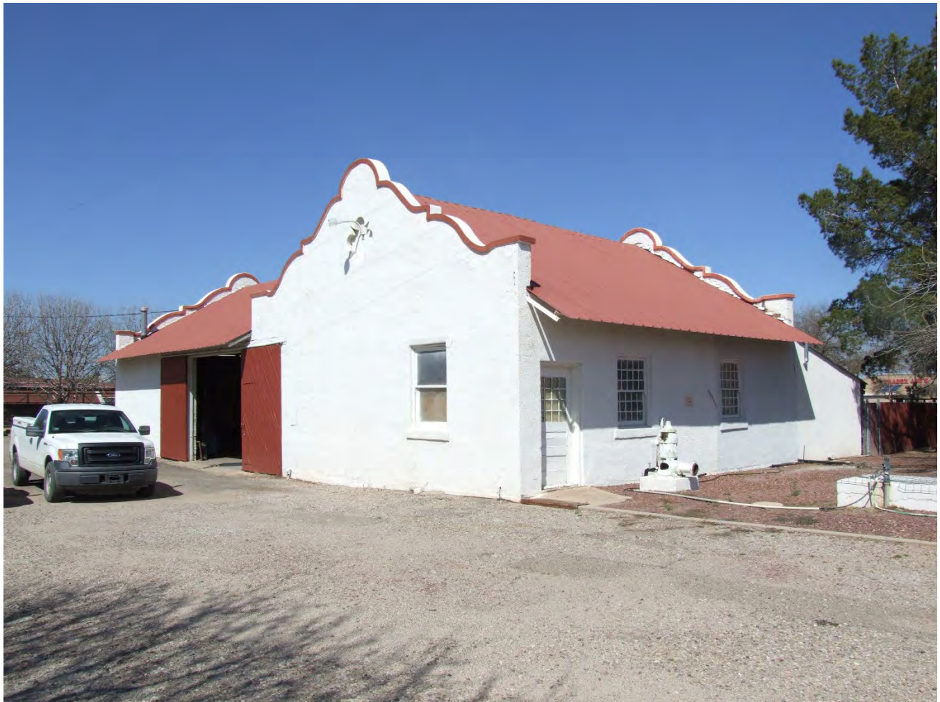
Photograph 10. East and south elevations of the Machine Shop; view facing northwest (AZ_Pima County_UA Campus Agricultural Center Historic District_0010).
