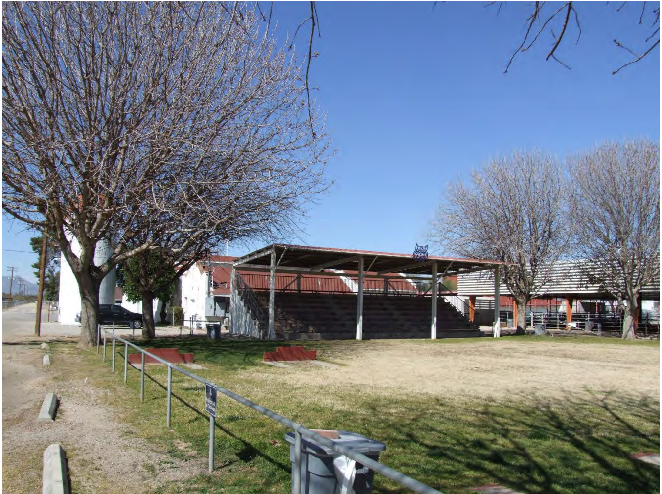
Photograph 26. Overview of Grandstand and field; view facing northwest (AZ_Pima County_UA Campus Agricultural Center Historic District_0026).
