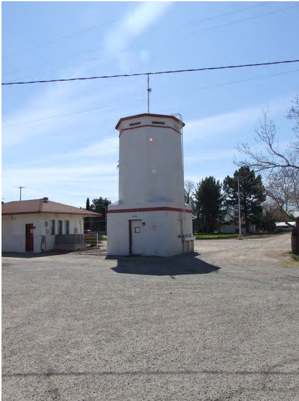
Photograph 11. East and north elevations of the Network Storage Building and Water Tower; view facing southeast (AZ_Pima County_UA Campus Agricultural Center Historic District_0011).
