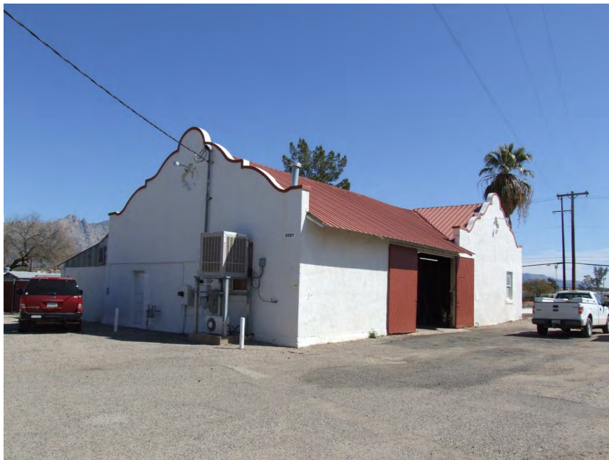
Photograph 9. West and south elevations of the Machine Shop; view facing northeast (AZ_Pima County_UA Campus Agricultural Center Historic District_0009)
