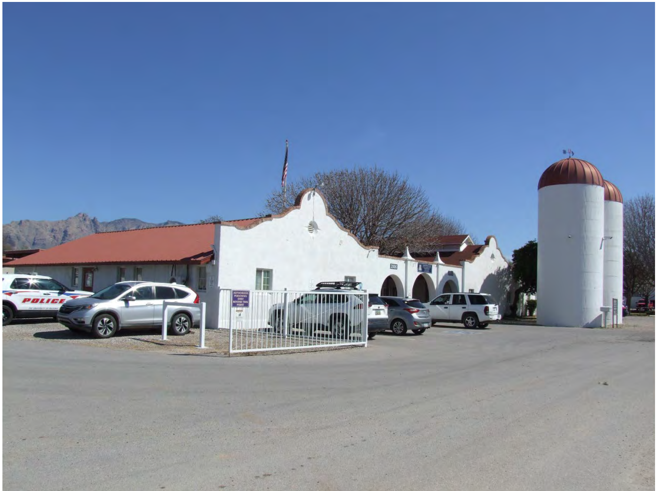
Photograph 18. West and south elevations of the Classroom Building; view facing northeast (AZ_Pima County_UA Campus Agricultural Center Historic District_0018).
