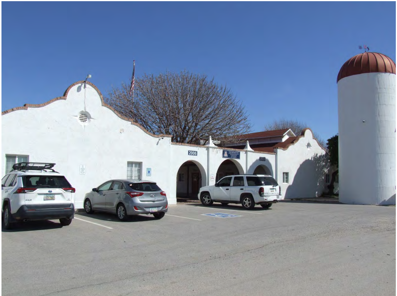
Photograph 16. South elevation of the Office Building and arched arcade openings; view facing northeast (AZ_Pima County_UA Campus Agricultural Center Historic District_0016).
