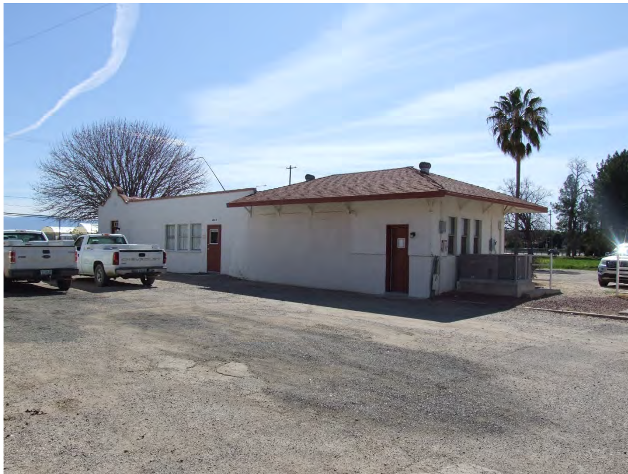
Photograph 24. West and north elevations of the Farm Office; view facing southwest (AZ_Pima County_UA Campus Agricultural Center Historic District_0024)
