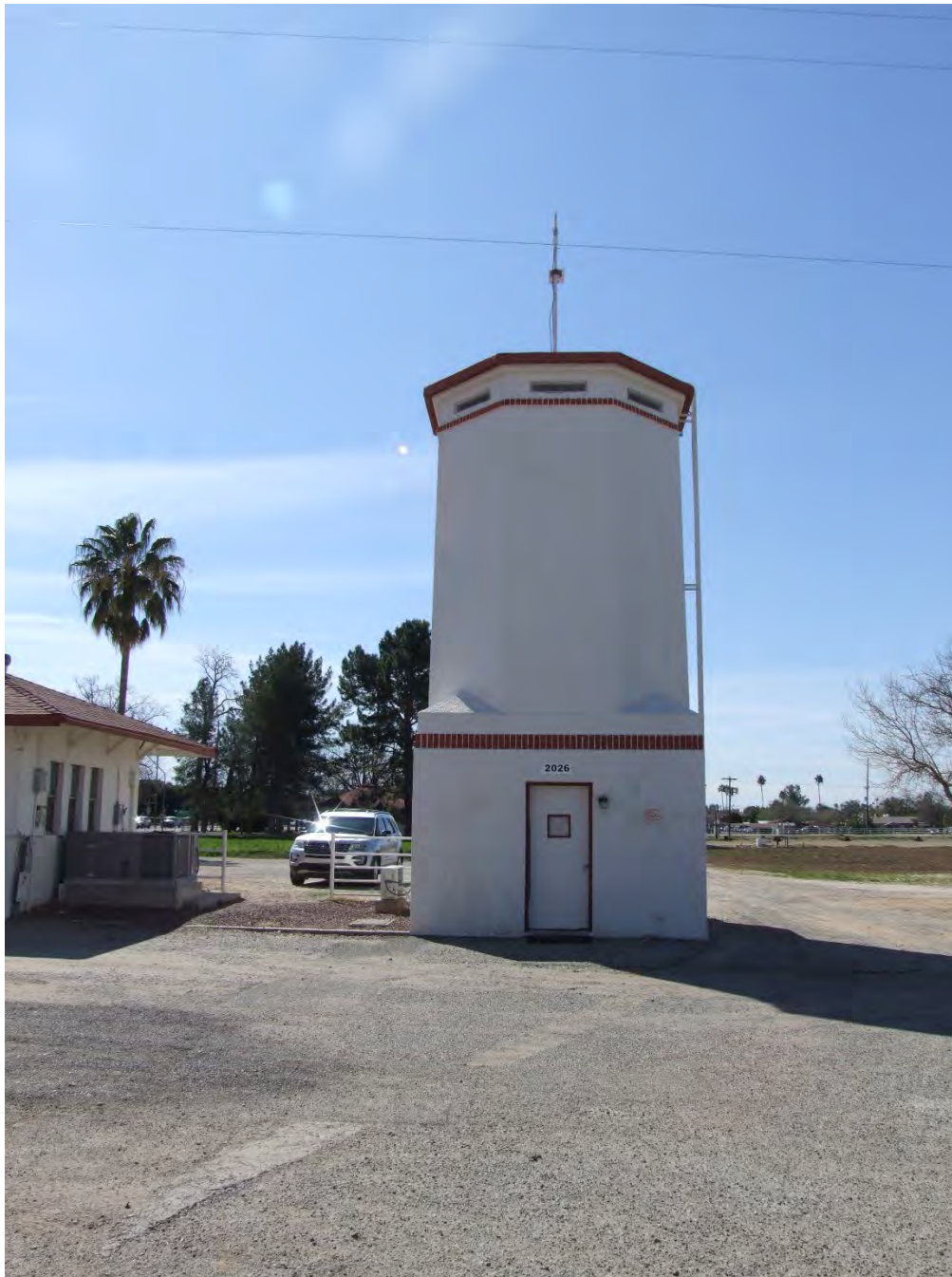
Photograph 12. Overview of north elevation of the Network Storage Building and Water Tower; view facing southeast (AZ_Pima County_UA Campus Agricultural Center Historic District_0012).
