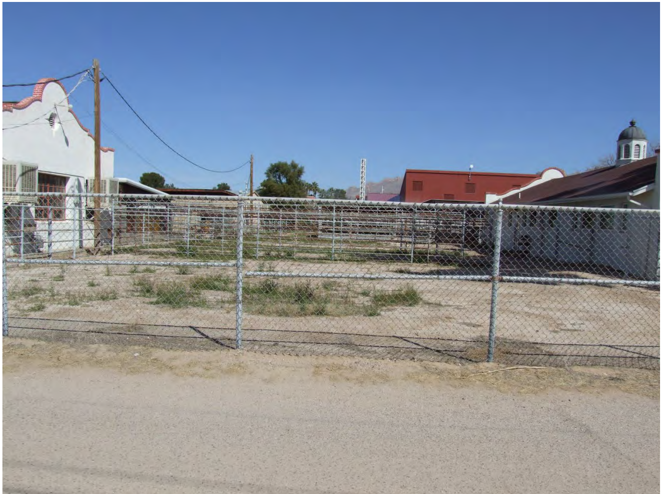
Photograph 14. Overview of Corral and fencing; view facing north (AZ_Pima County_UA Campus Agricultural Center Historic District_0014).
