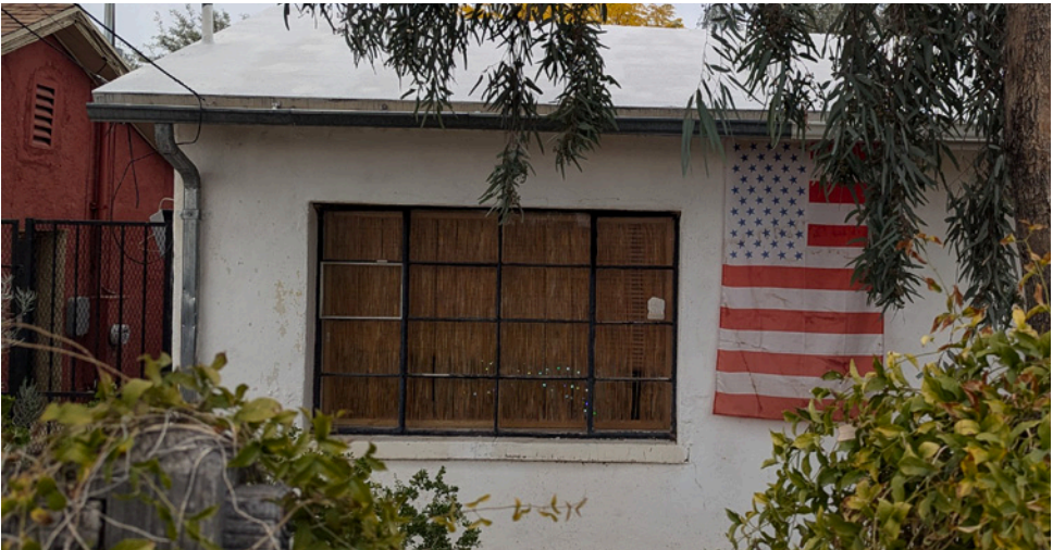
Fig 5 ~ 534 W 17th St metal casement window
