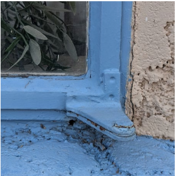
[3] 400 W Simpson - hinge & exterior seal
